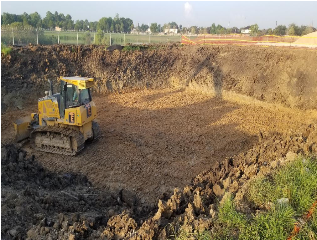
Backfilling the future Headworks area
