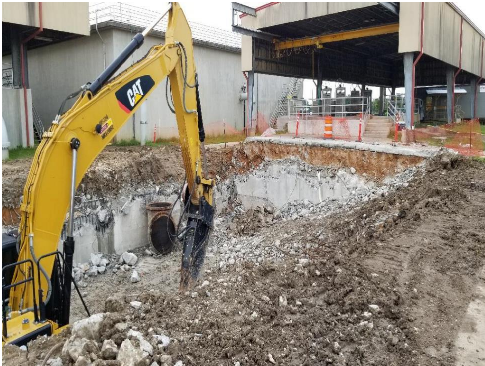
Demolition of the Surge Basin
