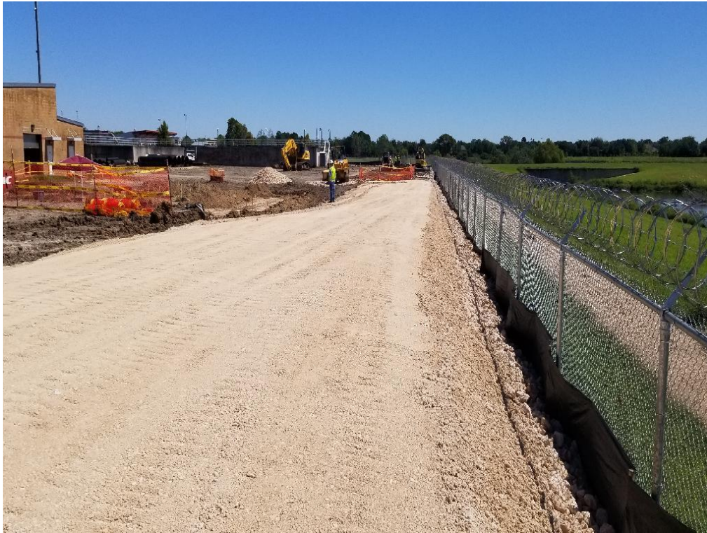
Site drainage on the south side of the plant site.
