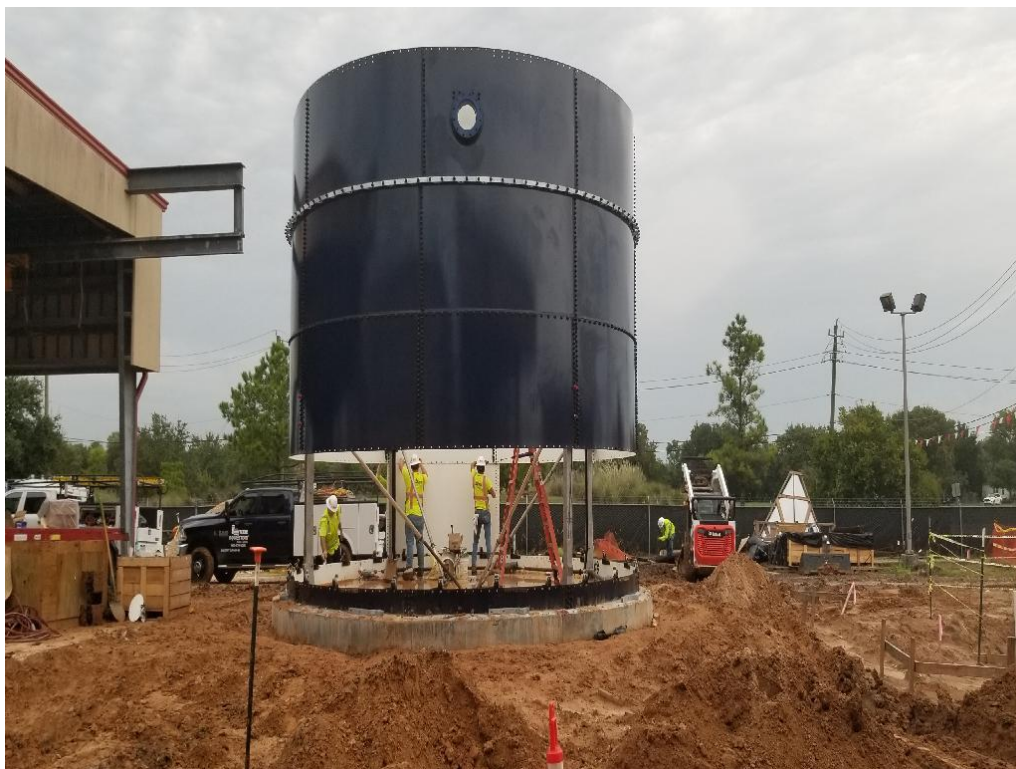
Construction of the Non-Potable Water (NPW) tank
