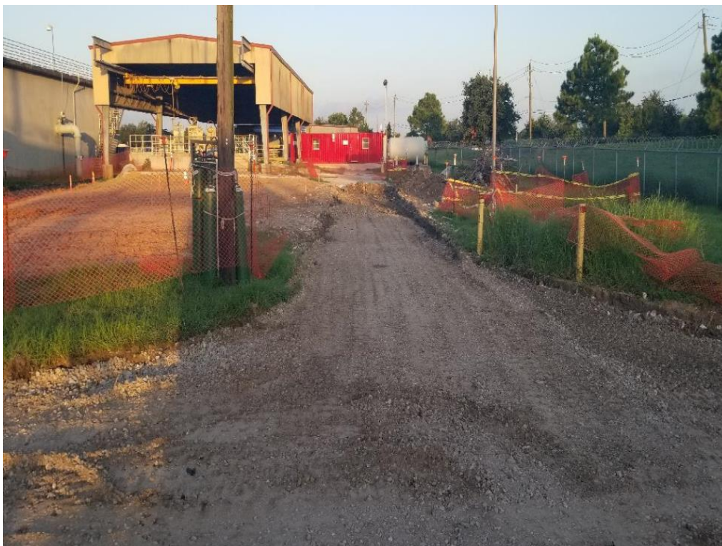
Construction Materials Testing on-site Laboratory location
