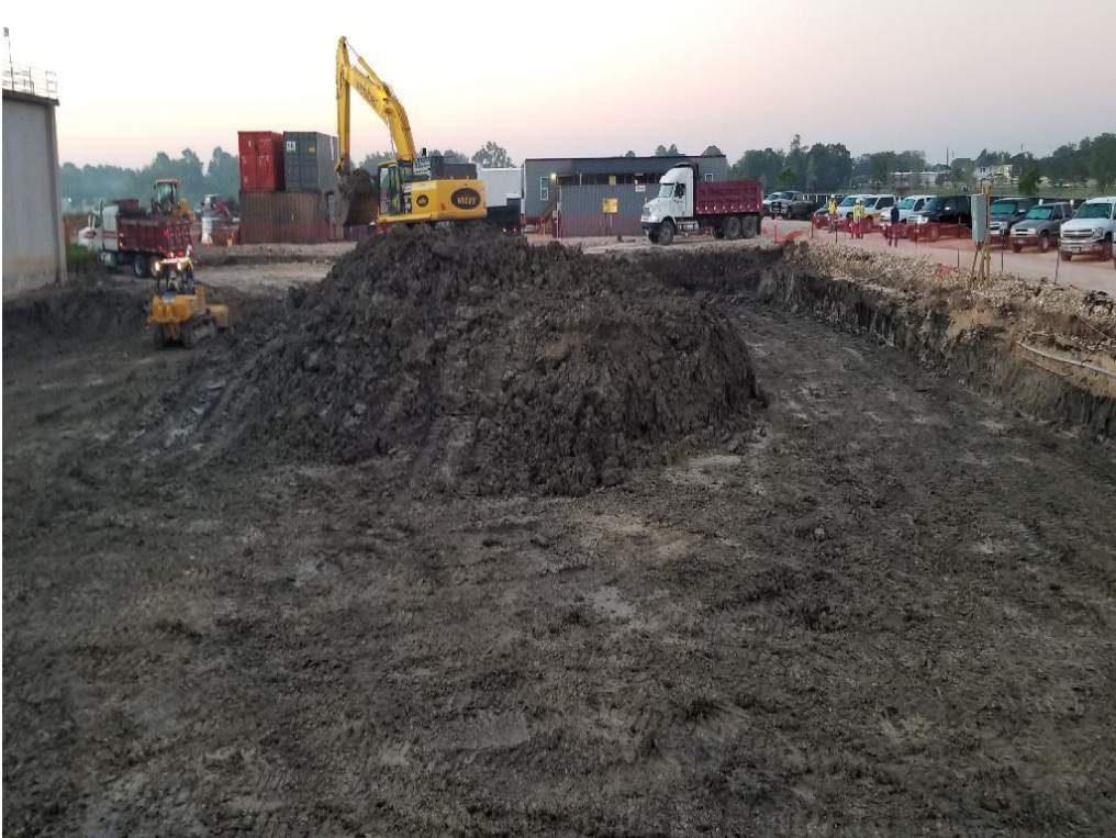
Removal of material from SBR 5 & 6 locations
