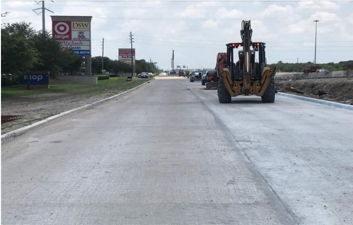
Newly Poured Northbound Frontage Road
