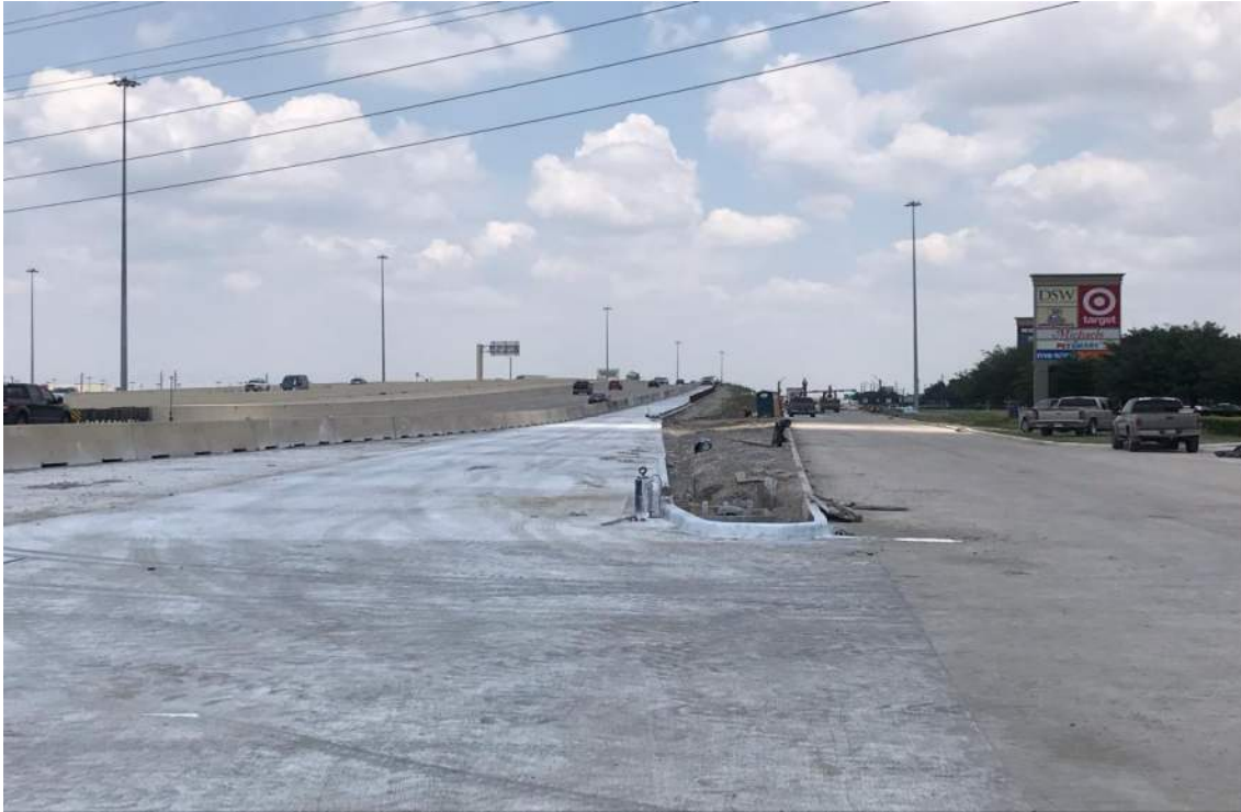
Northbound Entrance Ramp Cast-In-Place Concrete Railings
