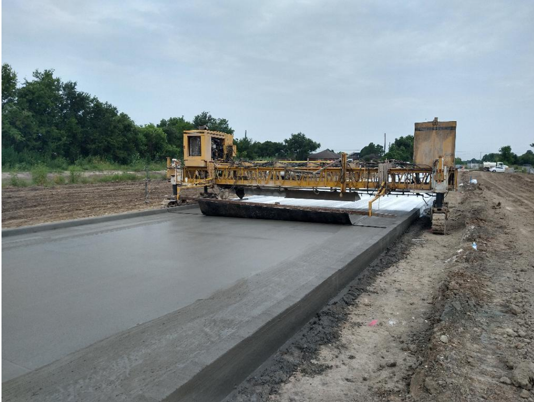
Slip-form paving operations between O'Day Rd. and Hatfield Rd.
