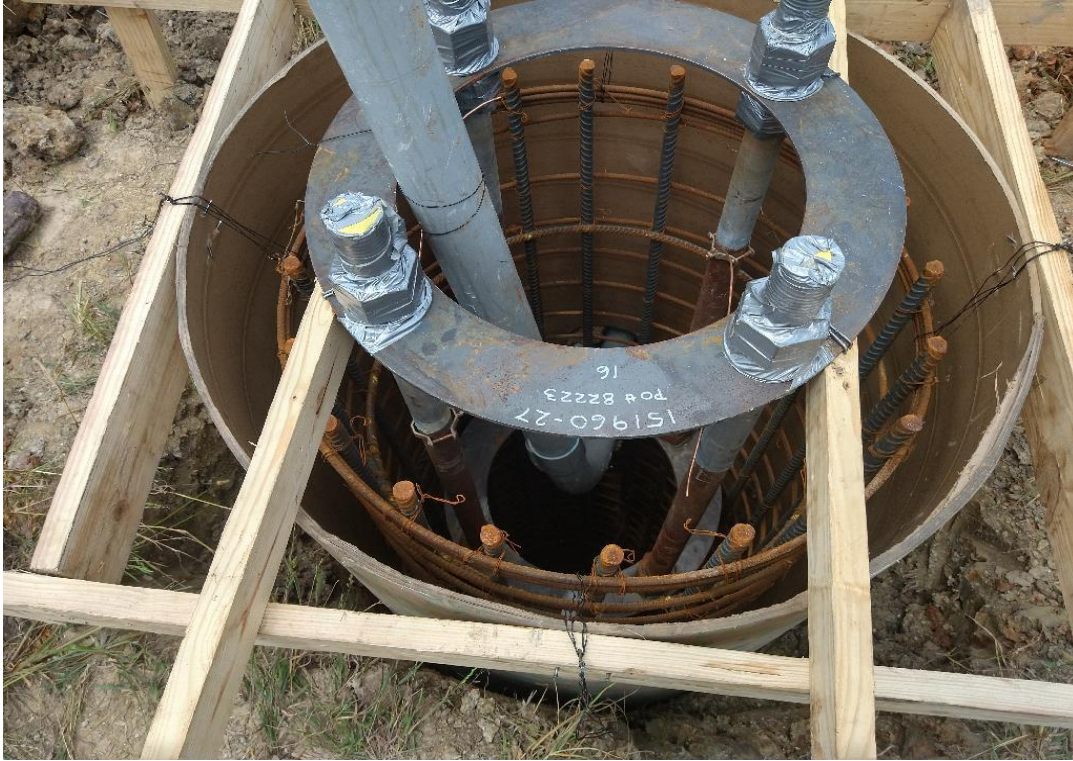
Traffic signal drill shaft at Max Rd.
