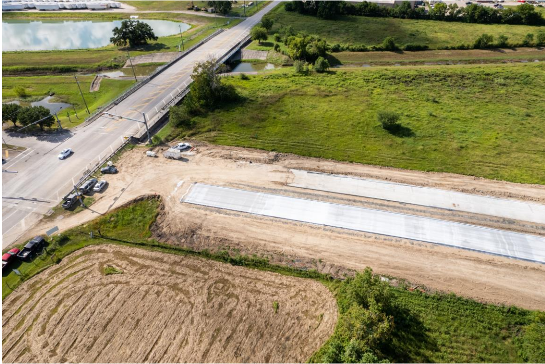
East and West bound paving operations at Mykawa Rd.
