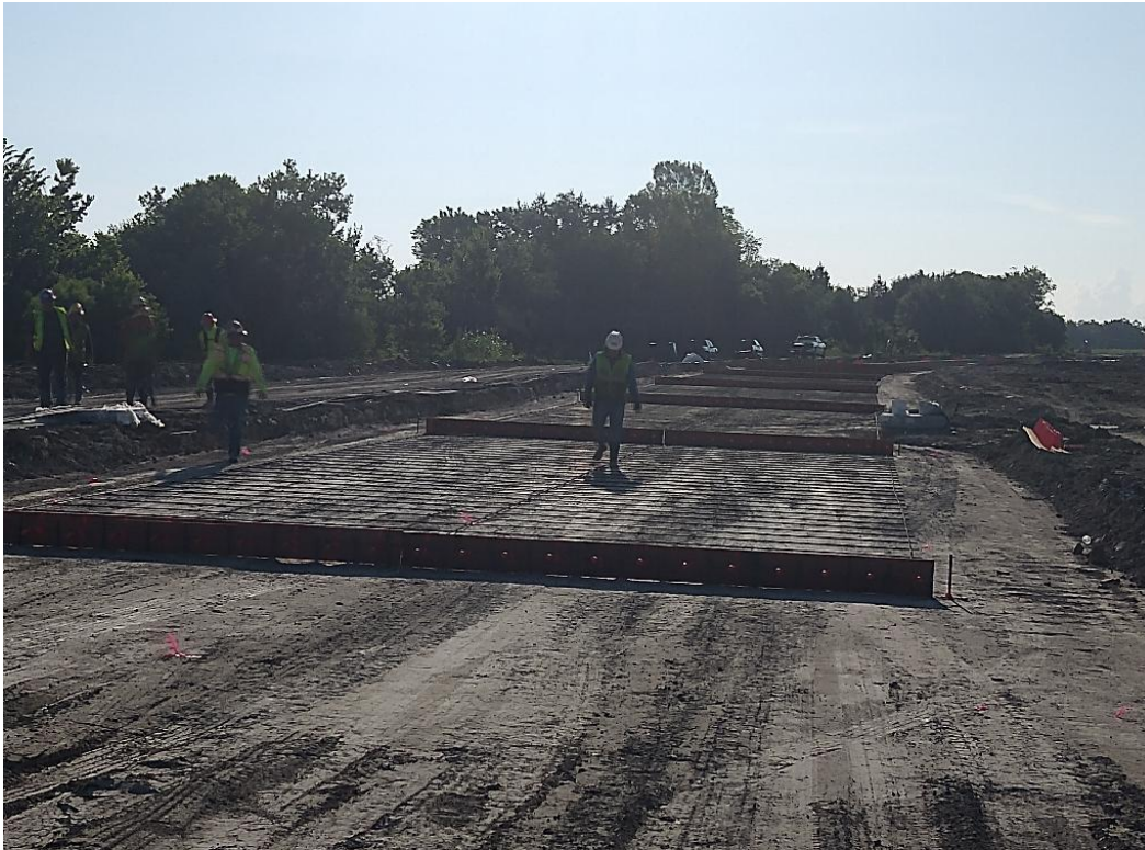
Rebar installation between Harkey Rd. and Woody Rd.
