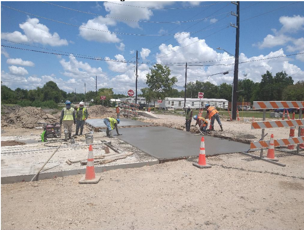
Fast-Track concrete installation at Stone Rd.
