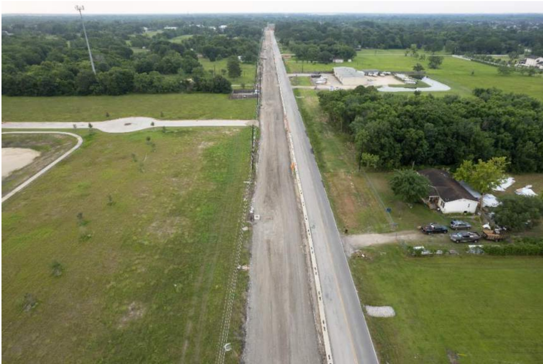
Lime stabilized sub-base between Cullen and Stone Rd.
