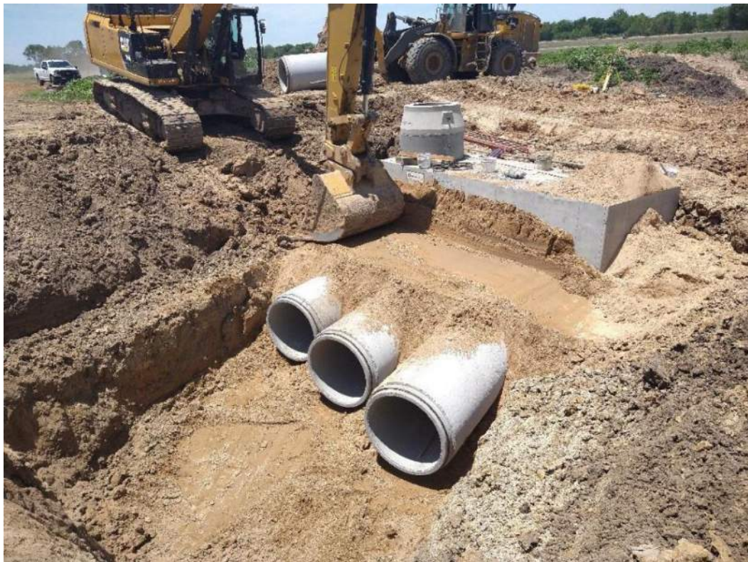
Hickory Slough outfall 19'x6' junction box installation
