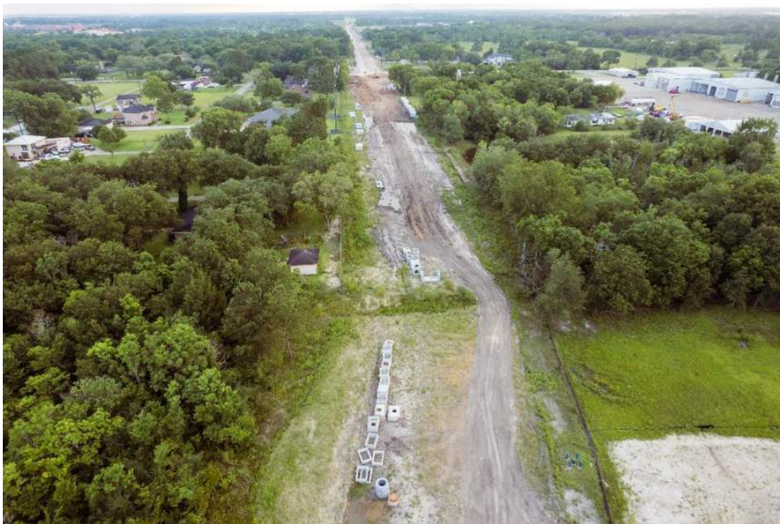
Drainage system installation east of Stone Rd.
