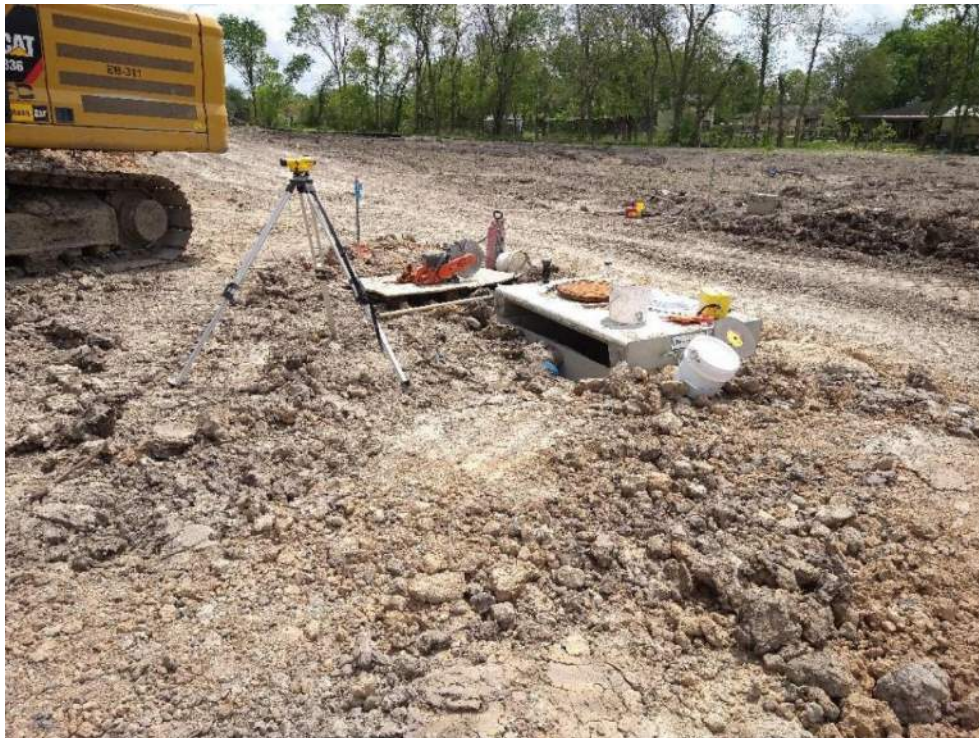
Installation of a curb inlet east of O'Day Rd.
