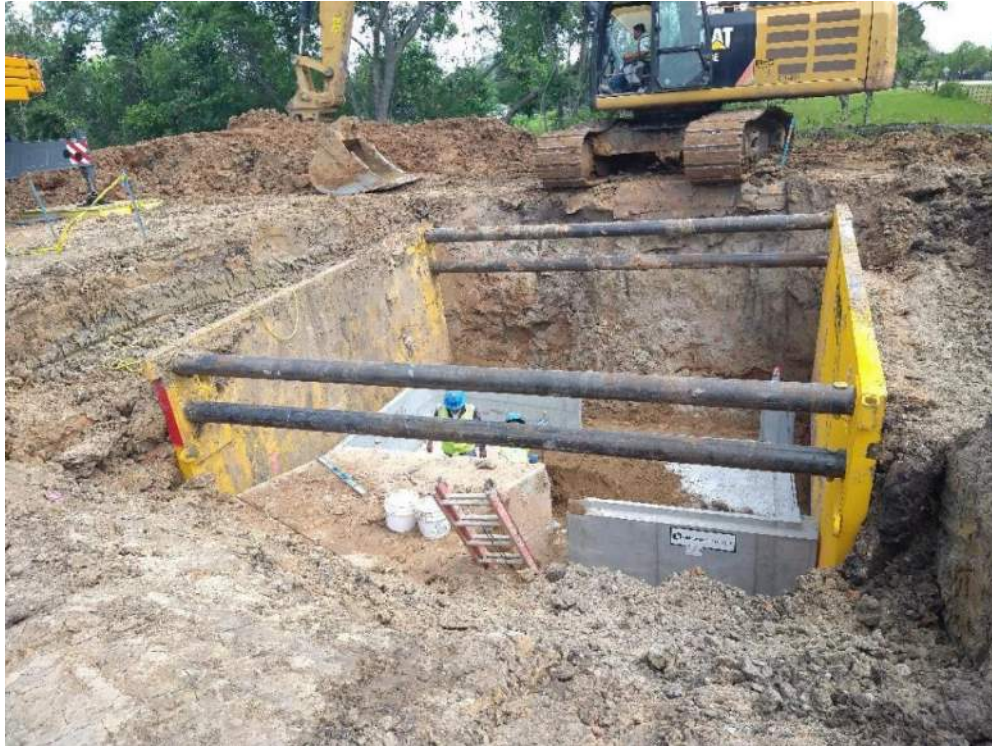
Shoring and ladder per OSHA safety requirements
