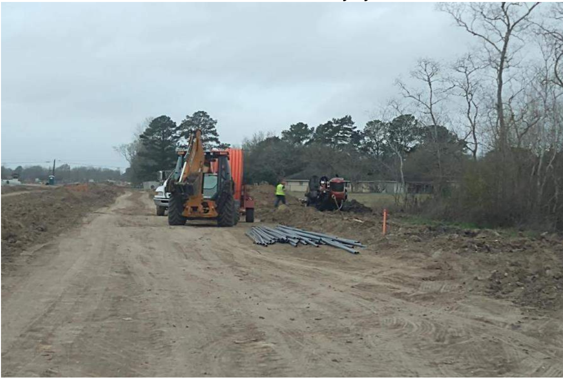
Installation of Conduit for Traffic Signals
