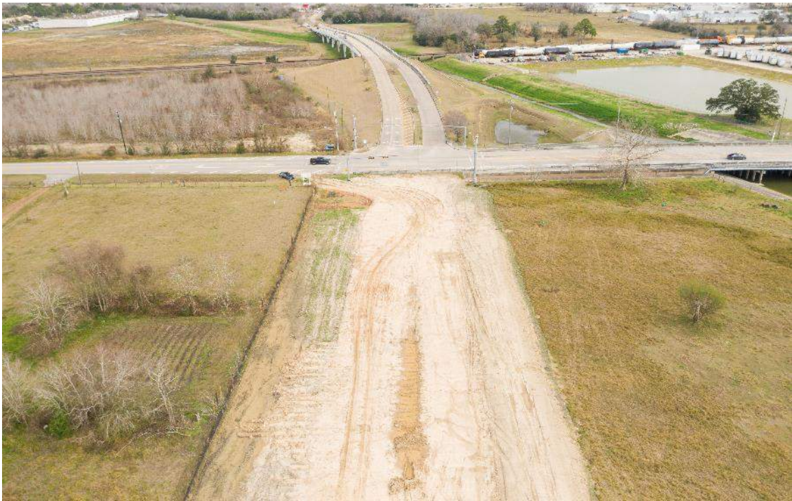
Cleared ROW at the Mykawa intersection
