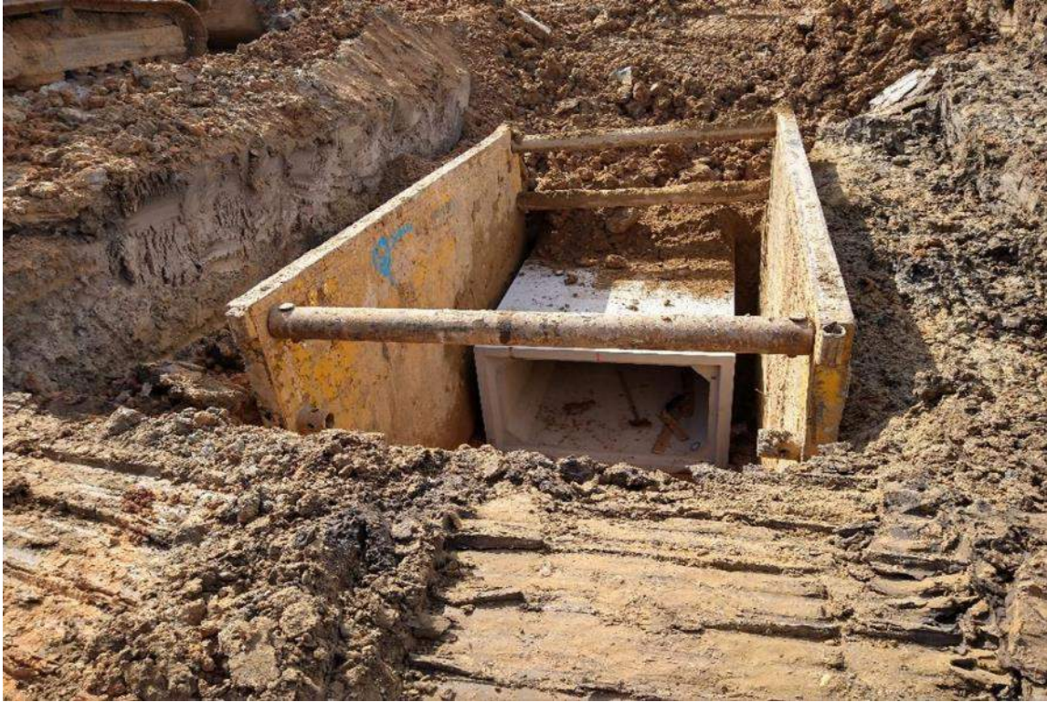
7' x 4' Reinforced Box Culvert (RCB)
