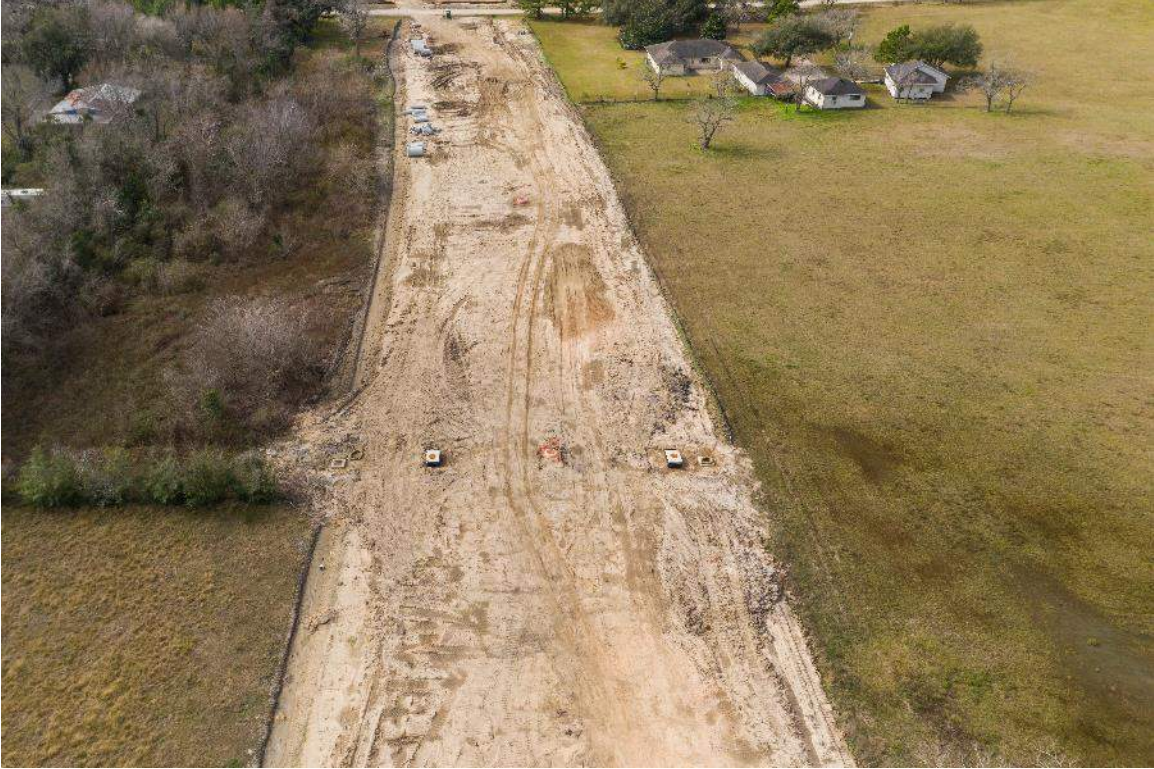
Installed inlets and curb grates
