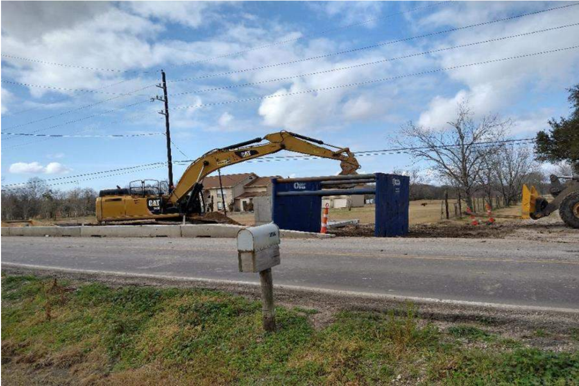
Installation of Trench Safety System
