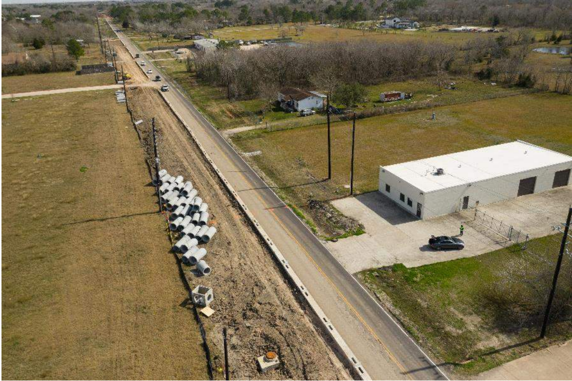
RCP drainage pipe to be installed between Cullen and Stone Rd.
