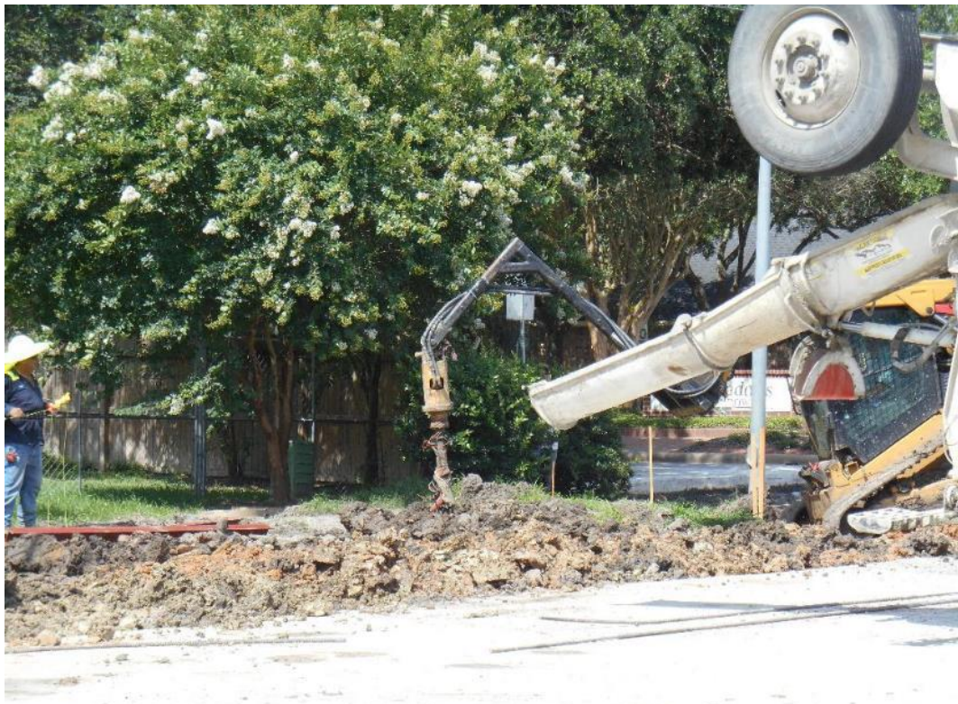
Pouring last drilled shaft foundation for Sound Wall D
