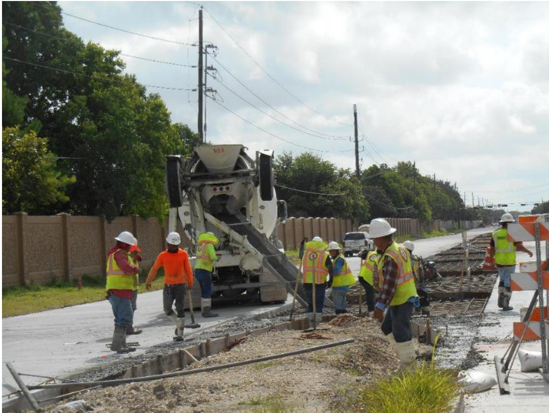
Pouring median crossing pavement (Phase 4 work)
