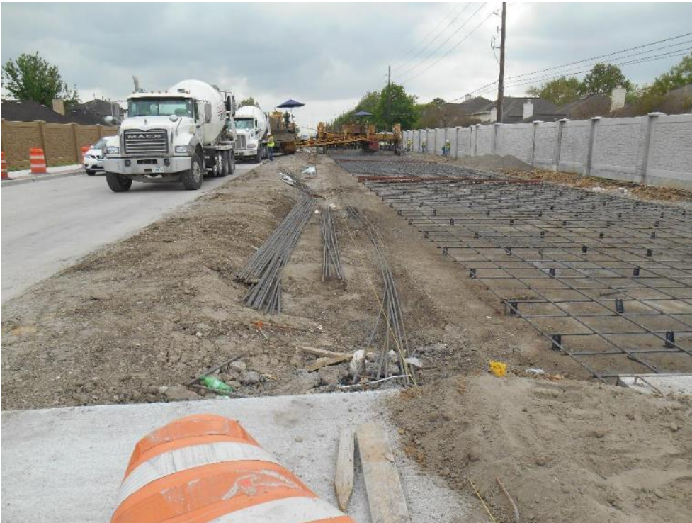
Westbound lane paving approaching Kensington Bridge, looking east
