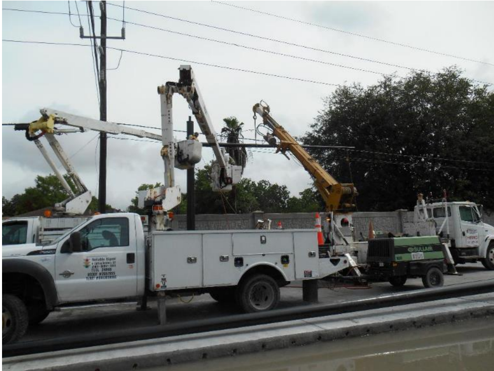
Installation of traffic signal pole at Miller Ranch
