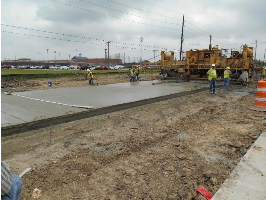
Paving Westbound lanes at Dawson High School
