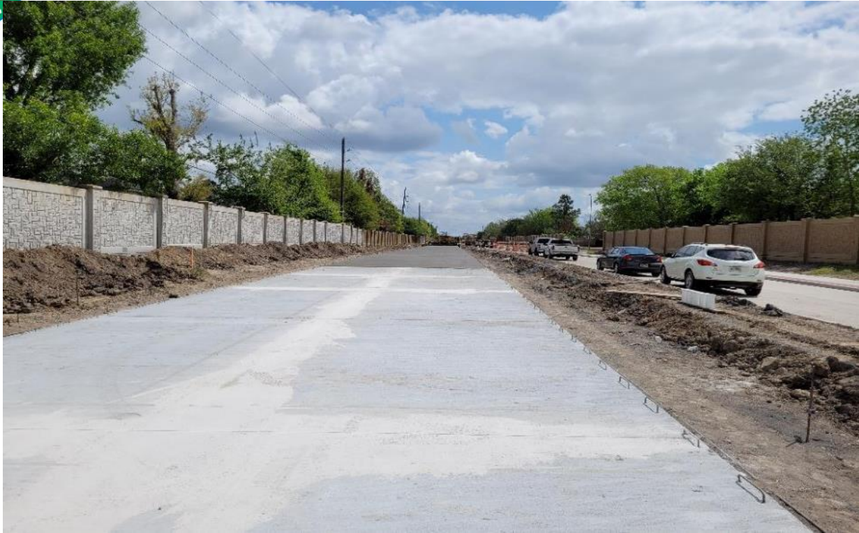
New Pavement on westbound lanes
