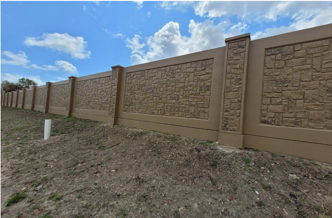
Finished Soundwall after completion of Painting
