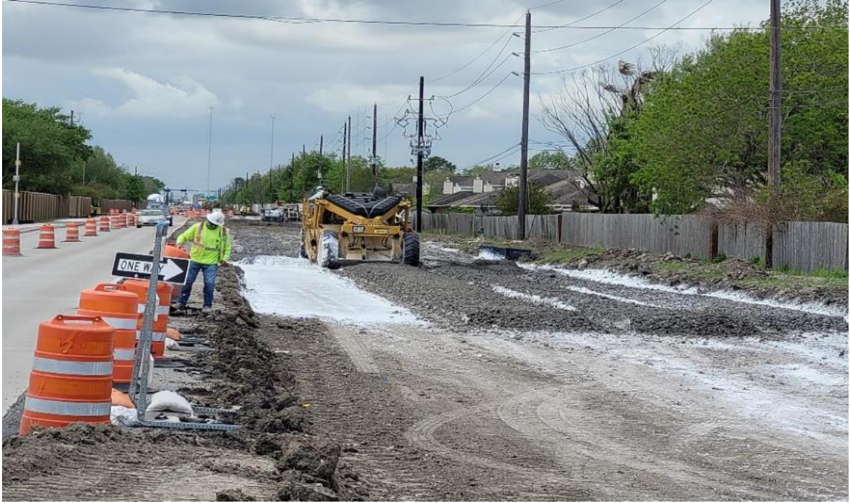
Lime stabilization of subgrade for westbound lanes.
