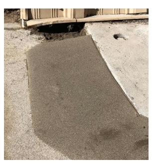
A8 - Slicing (Concrete slicing to remove trip hazard)
