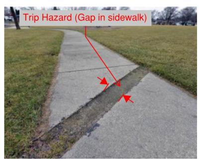
A7 - Temporary Patch (asphalt repair of trip hazard on concrete sidewalk)
