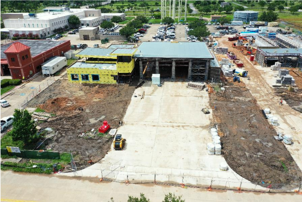
Drone Image of Front of Building
