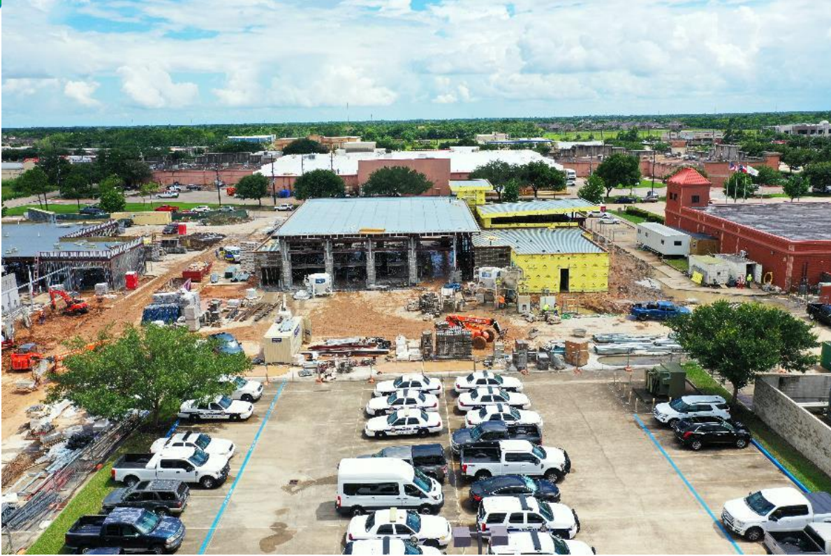
Rear Image of Fire Station
