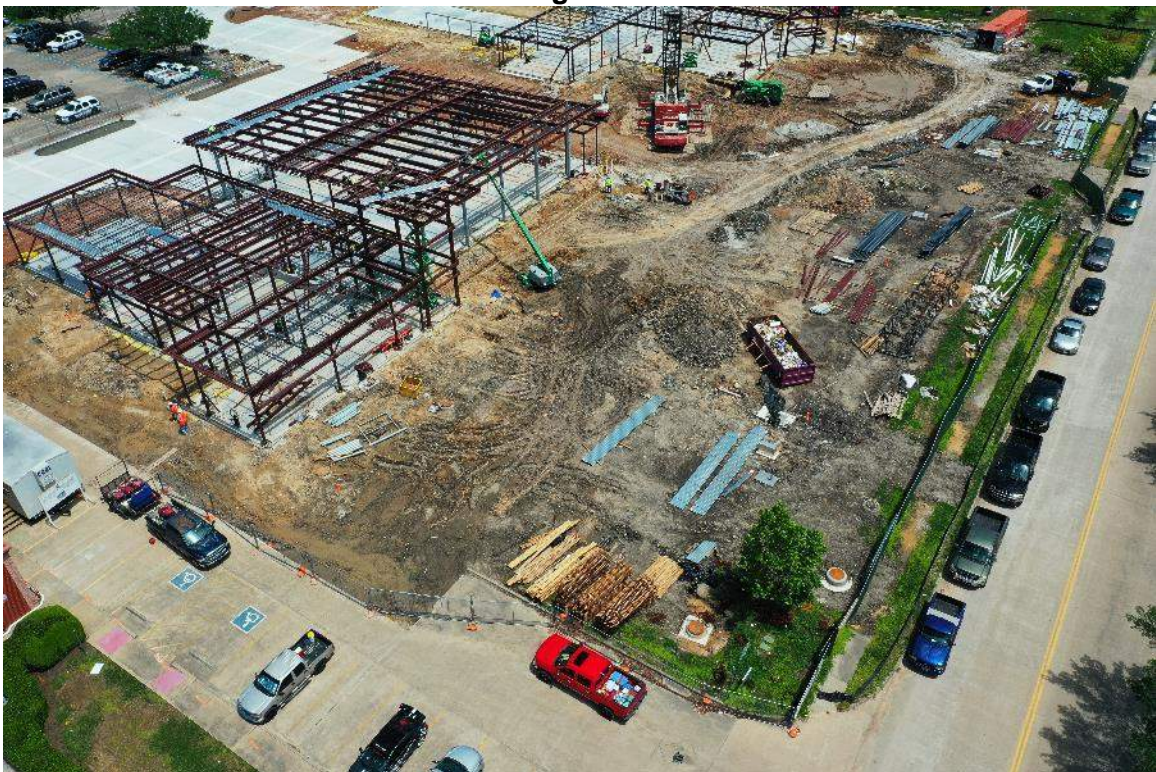
Structural Steel Being Erected
