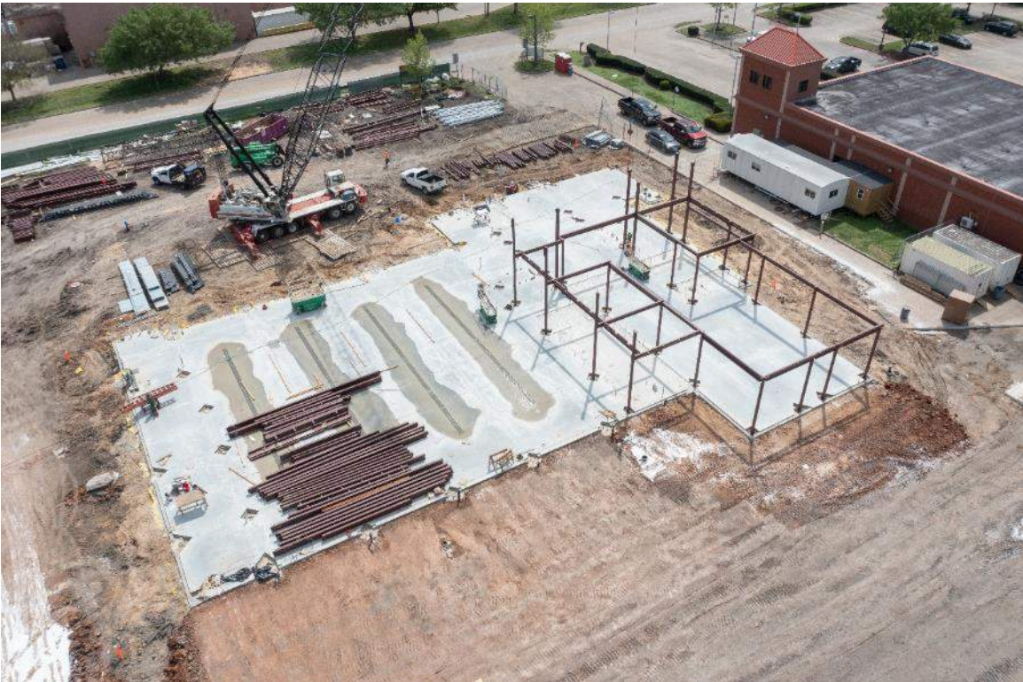
Structural Steel Being Erected
