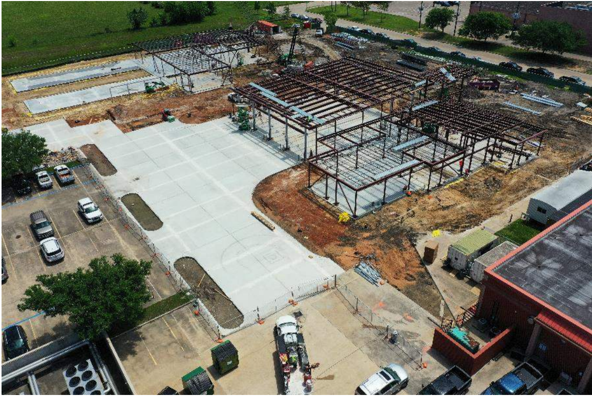
Northern Paving Has Been Poured
