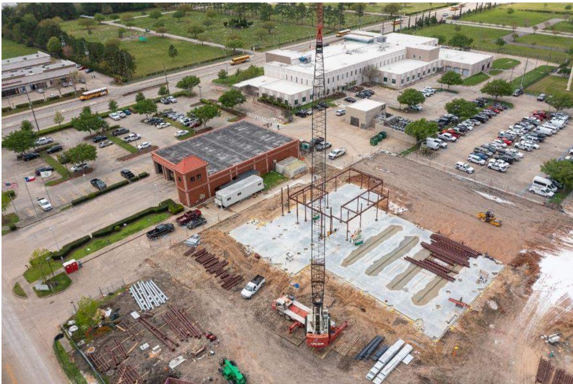
Existing Fire Station #4
