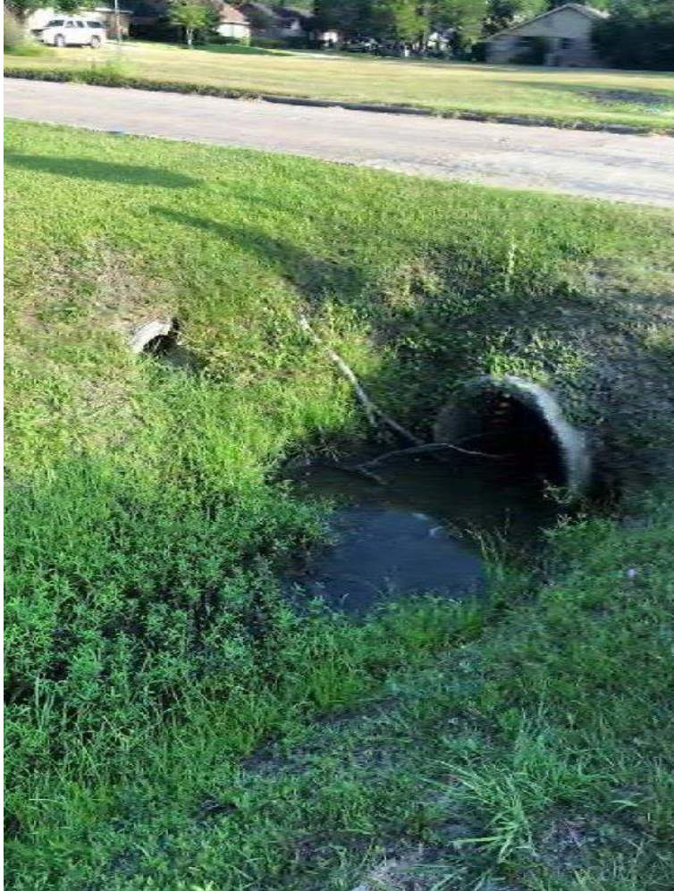
Culvert crossing at the corner of Cherry Street and Mykawa Road
