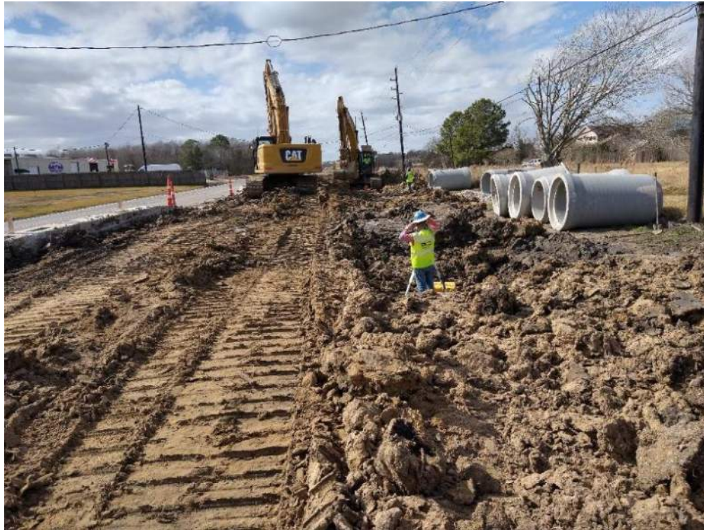
Installation of Drainage System Pipes
