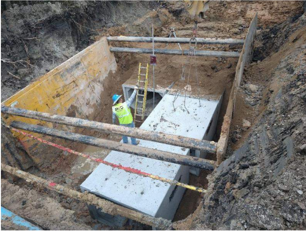
Installation of 6 x 4 Boxes
