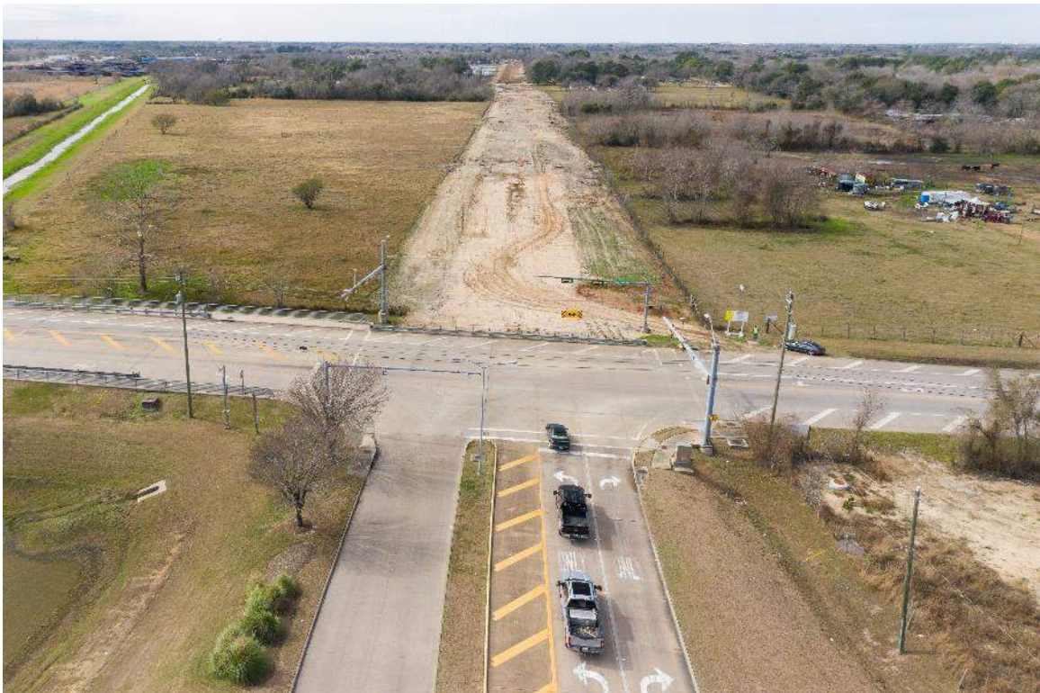
ROW prep at Mykawa Rd.
