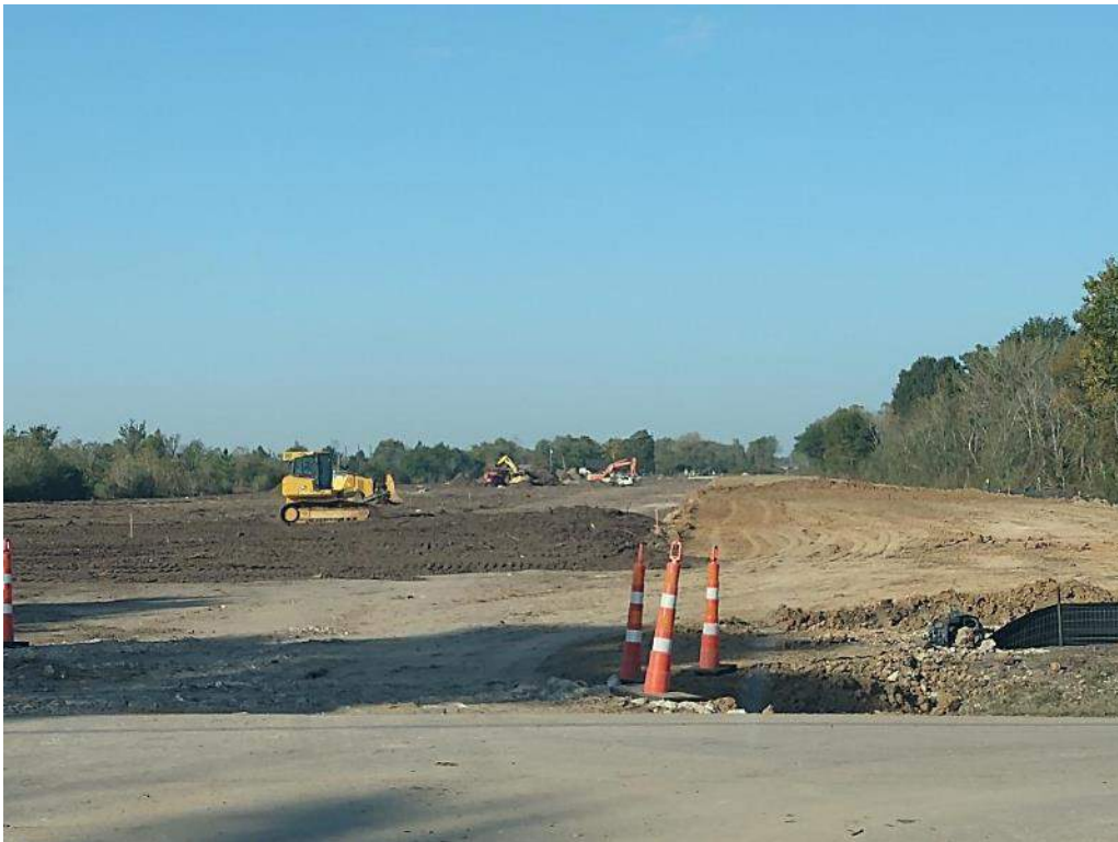
Embankment at Hickory Slough Drainage System Detention Pond 2
