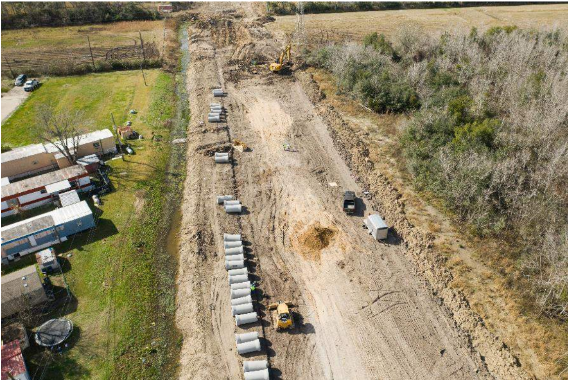
Hickory Slough Drainage System drainage pipe installation near Garden Rd.
