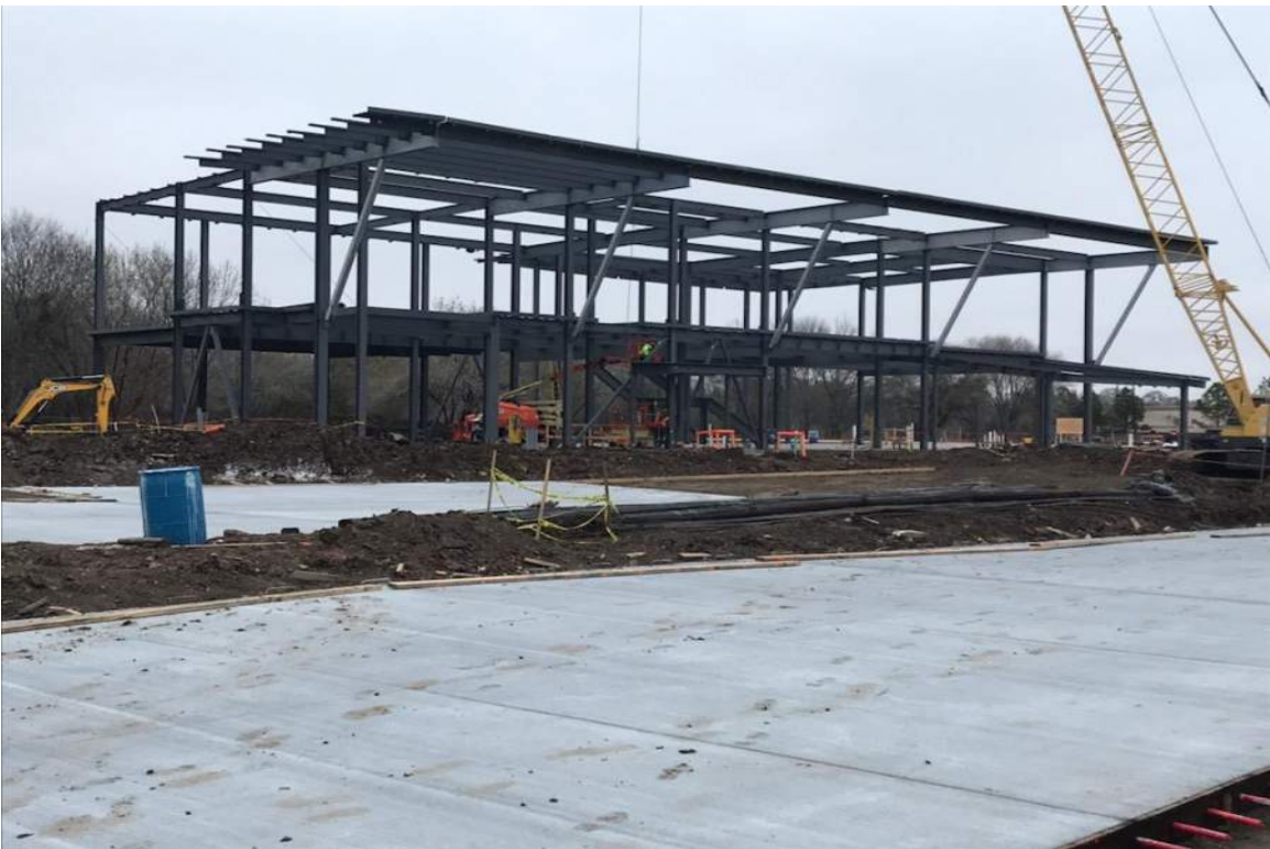
Steel Erection has Begun
