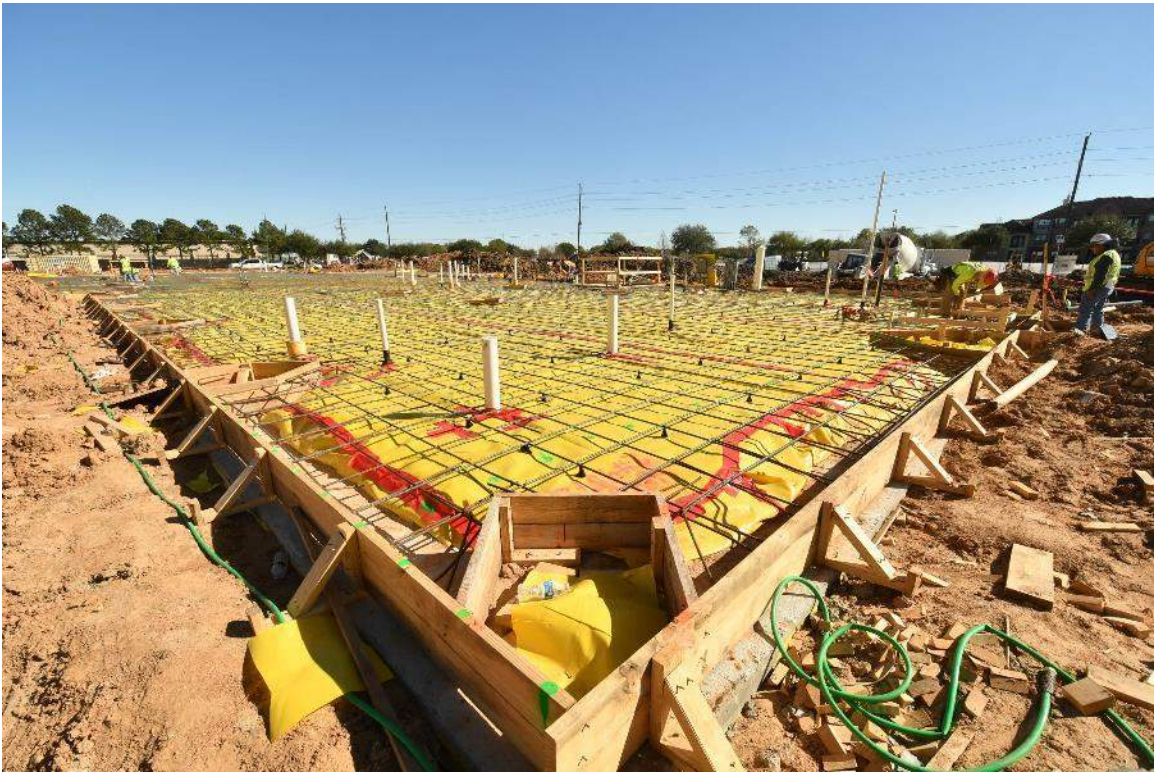
Plumbing Underground Installed
