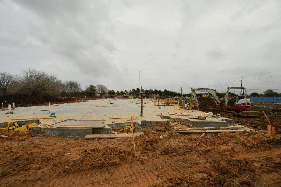
Slab Poured and Forms Removed
