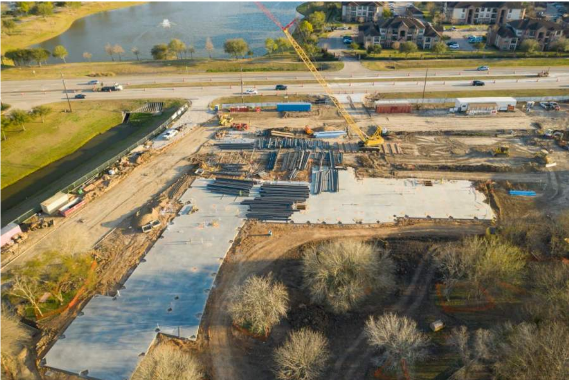
Aerial Photo of Poured Slab
