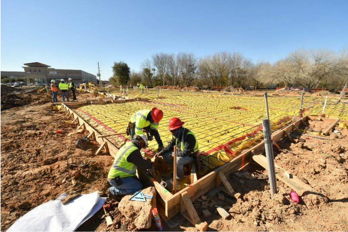
Steel Being Tied-In
