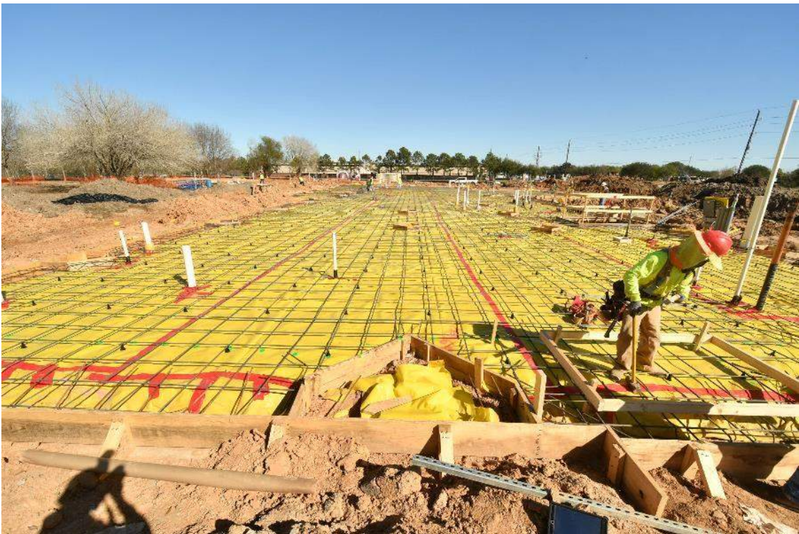
Forms Set and Rebar Tied-In Place
