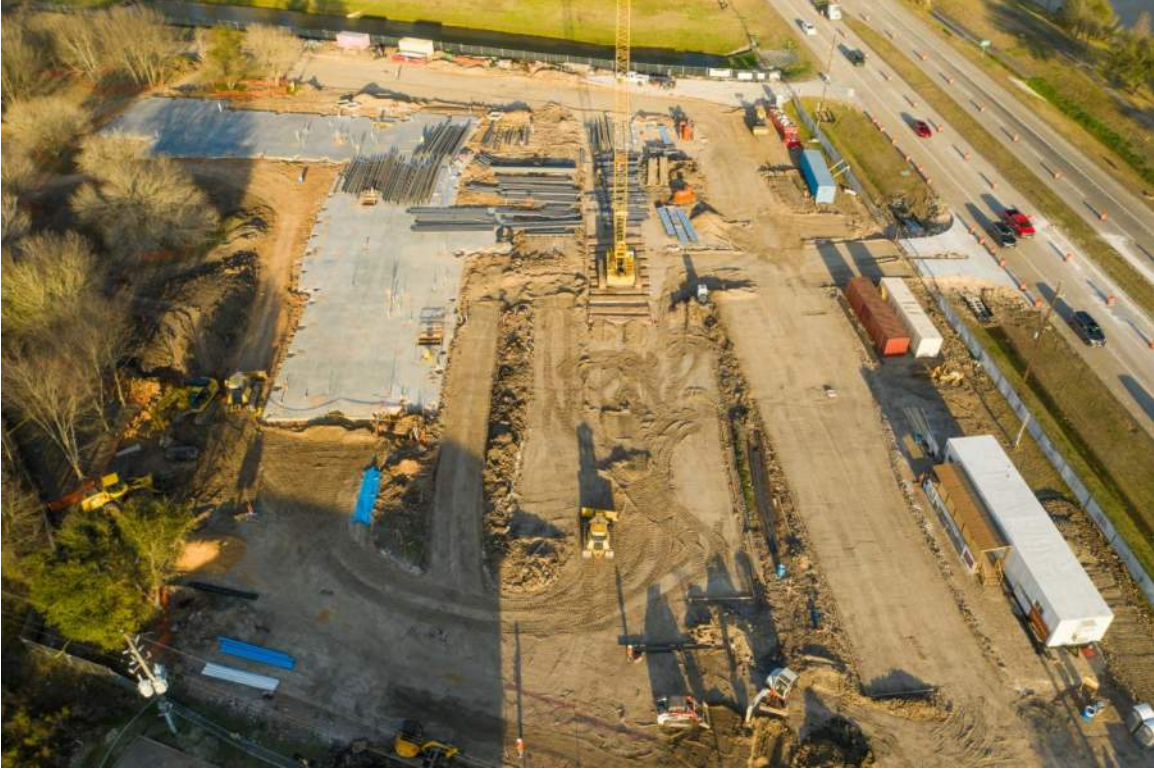
Steel Laid Out for Erection
