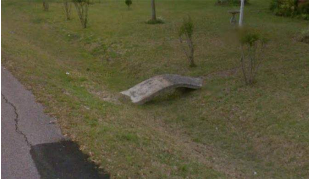
Concrete foot bridge over a drainage ditch that will be regraded
