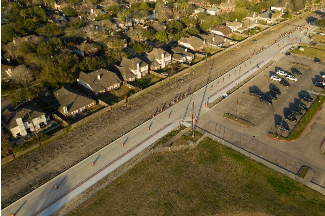
Challenger Elementary Bus Pick-up/ Drop-off and parking
