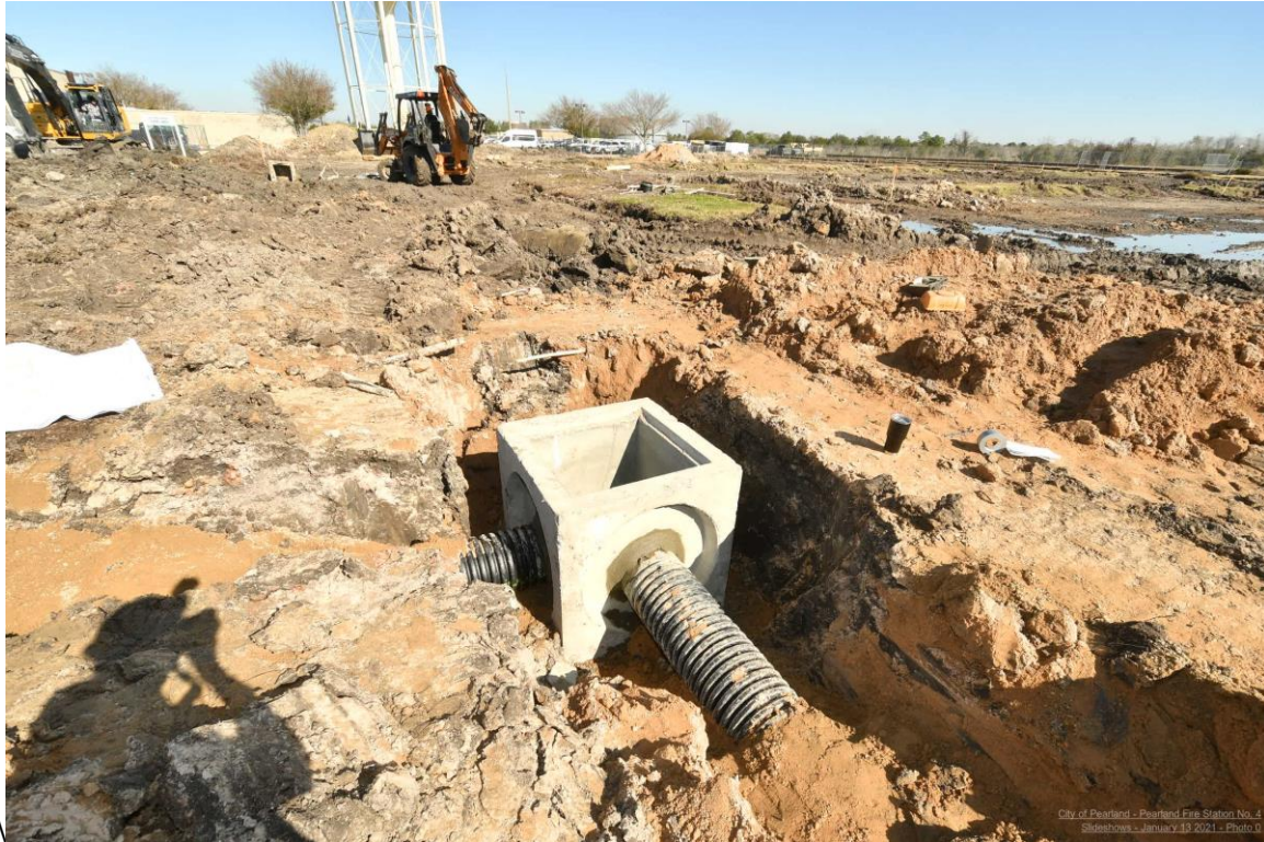
Storm Sewers Being Installed
