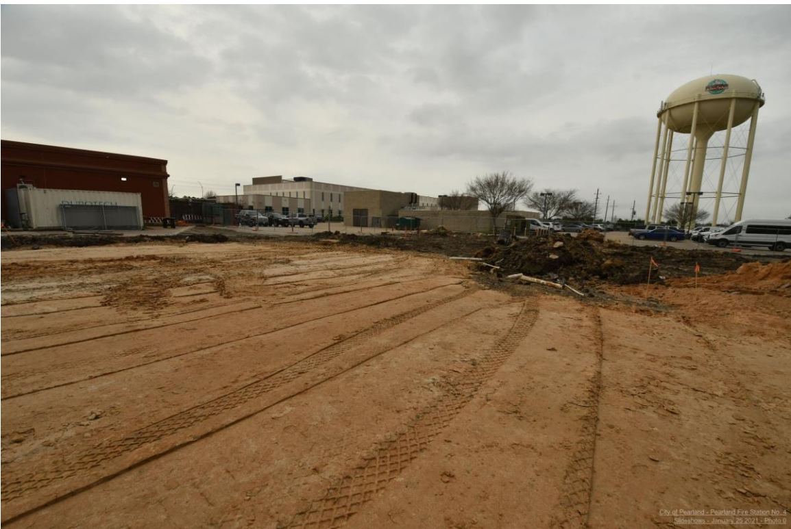
Pad Has Been Imported and Ready for Plumbing Underground
