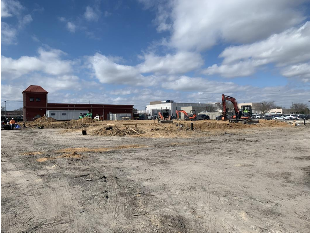
Plumbing Underground Being Installed
