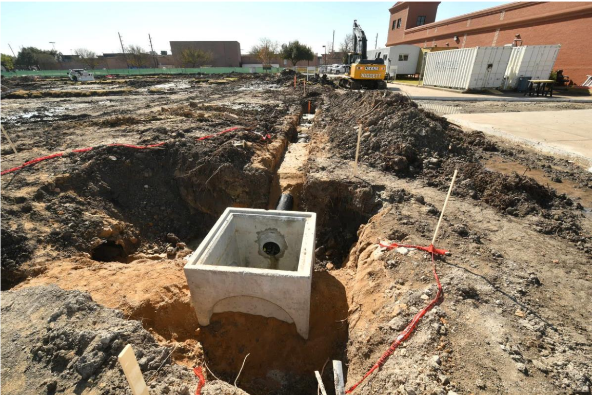
Storm Sewers Being Installed
