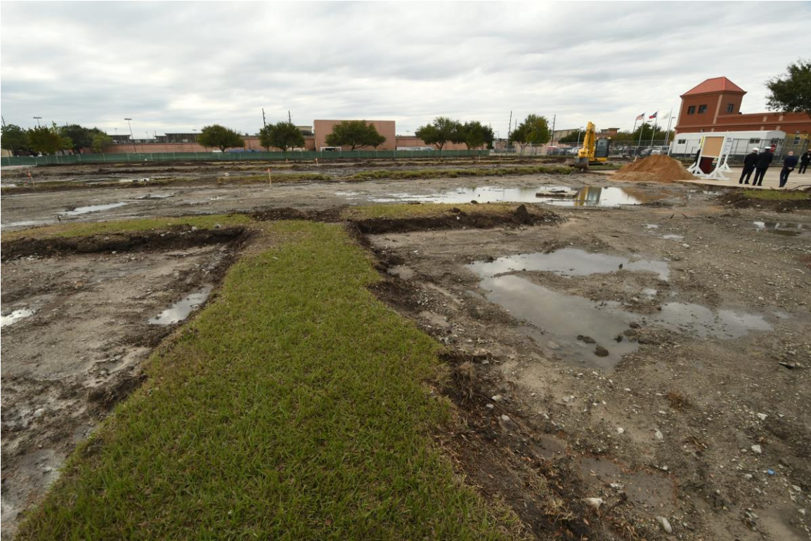
Site Demoed and Ready for Excavation
