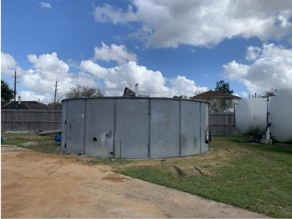
Removal of Tank
