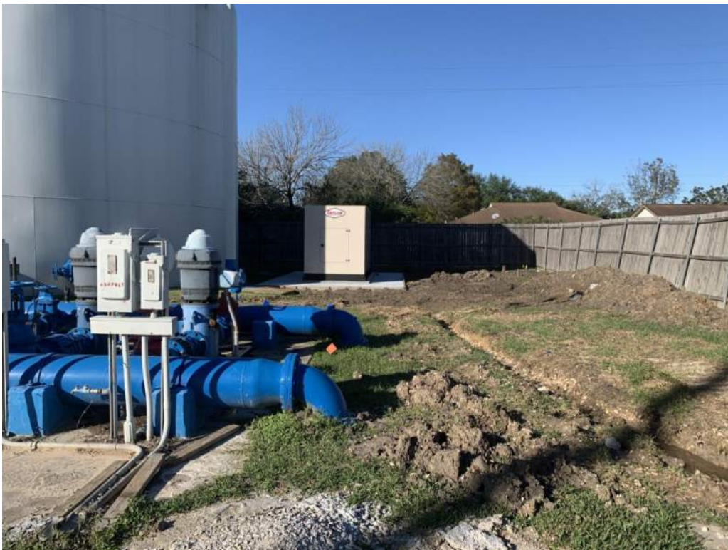
Generator Has Been Installed
