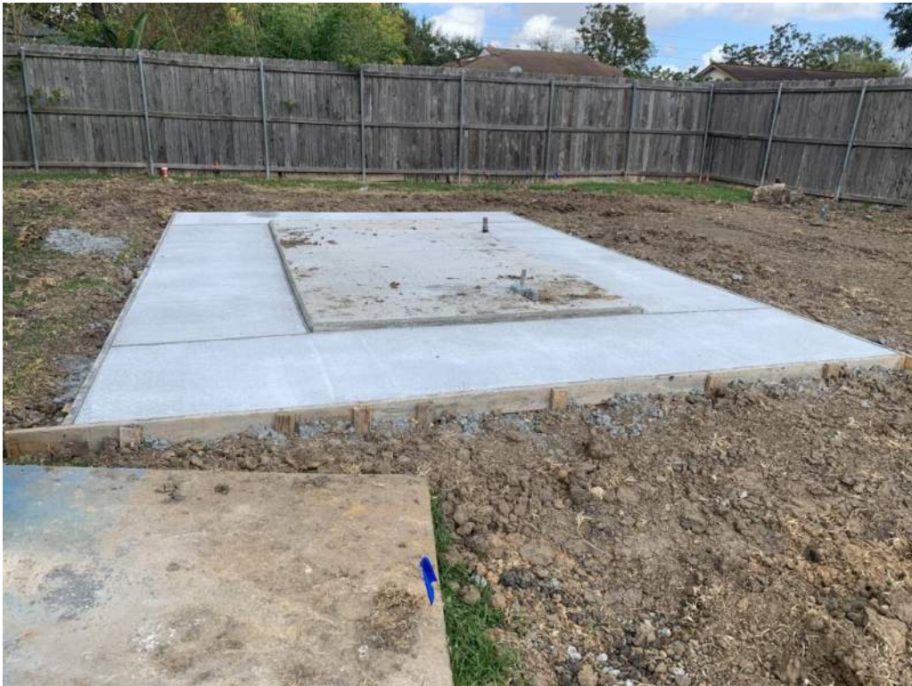
Generator Pad Poured
