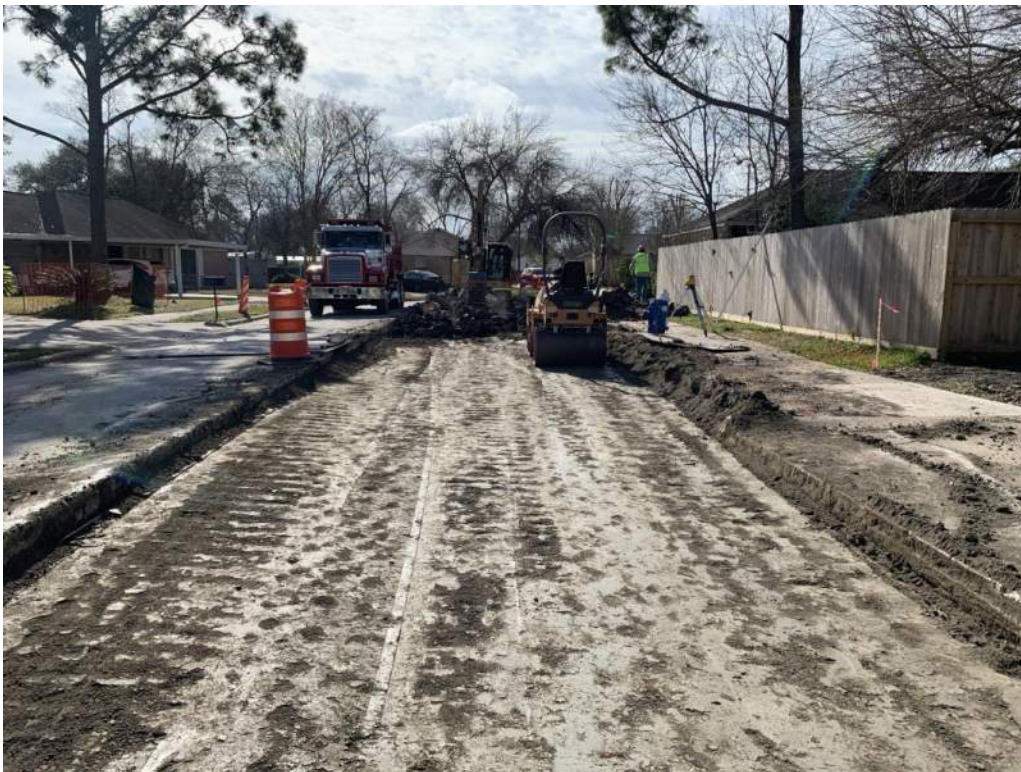
Removal of Old Base Material and Compaction of New Base Material
