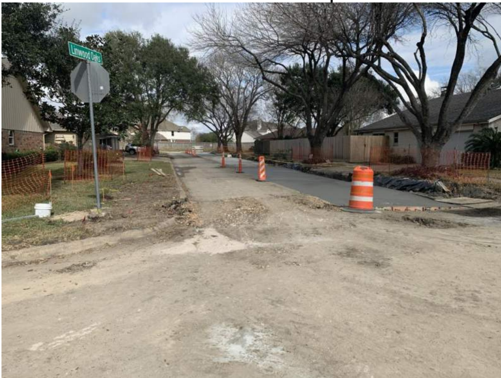
Freshly Poured Paving at Linwood Oaks
