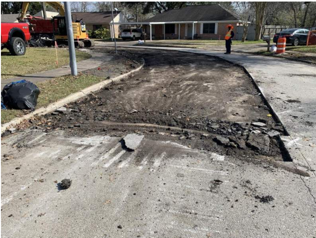
Removal of Paving on Orange Circle South
