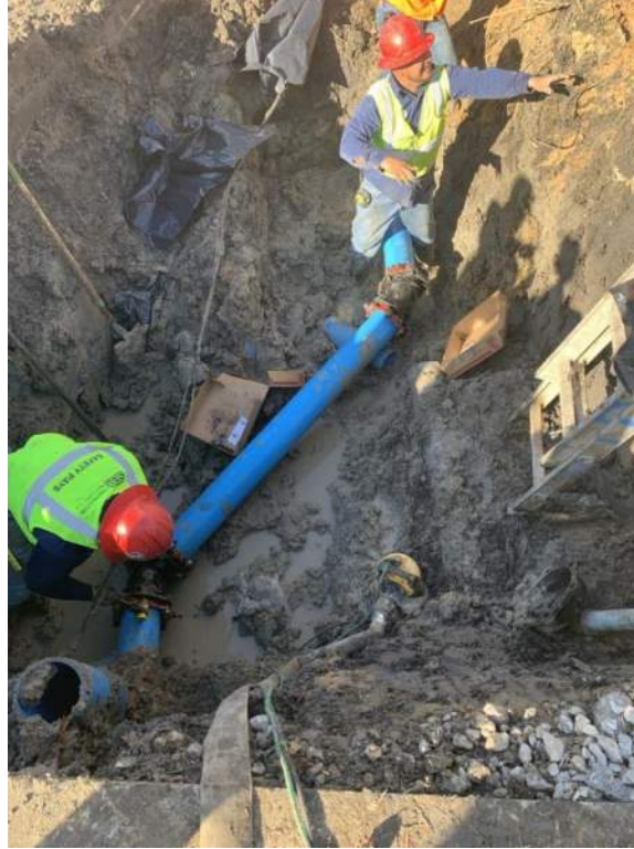
Connection of 6" water line on Orange Circle
