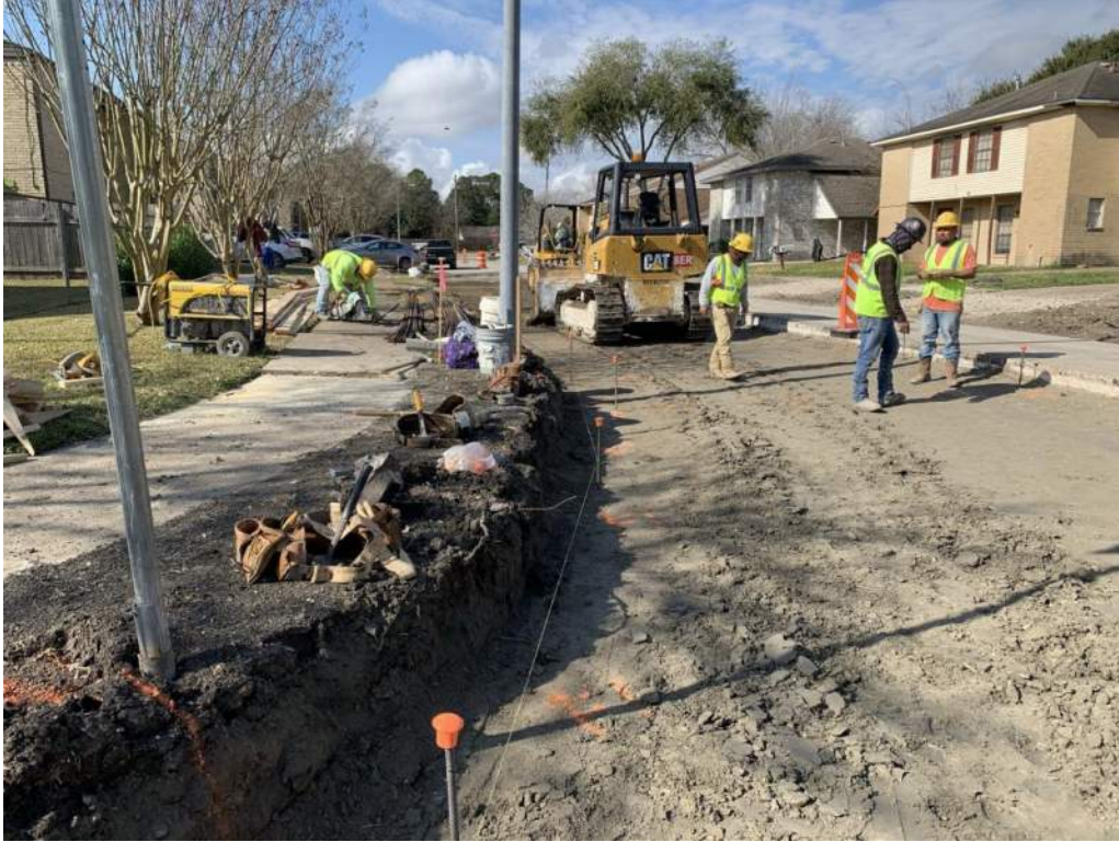
Compaction of Subbase on Orange Circle
