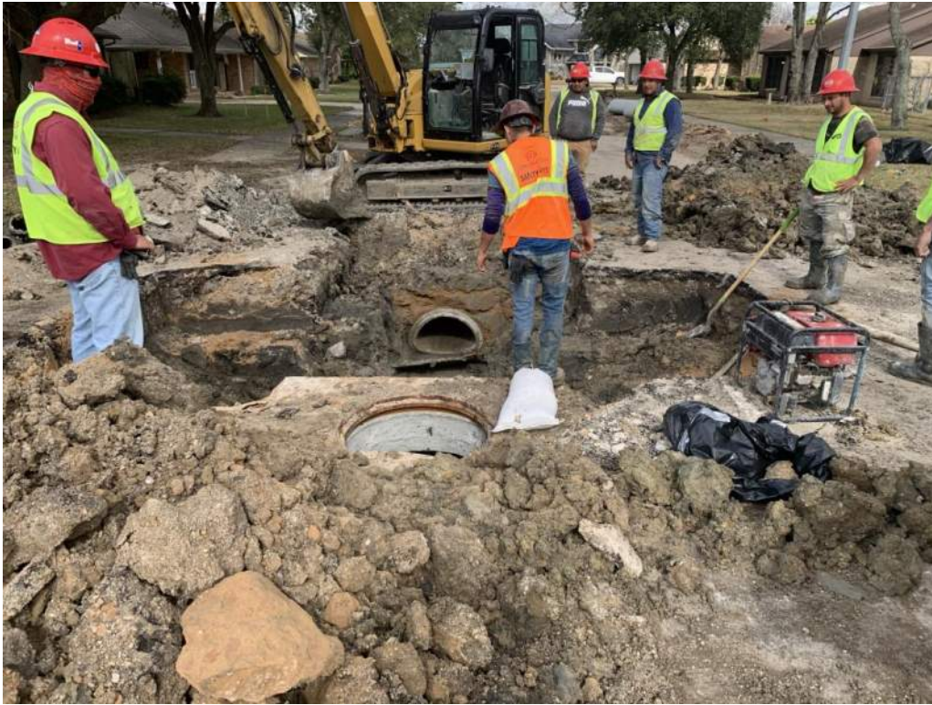
Installation of Storm Sewer at Yupon Circle
