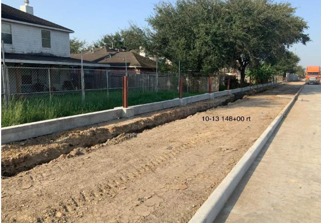
Foundations and Beams set for Soundwall H.
