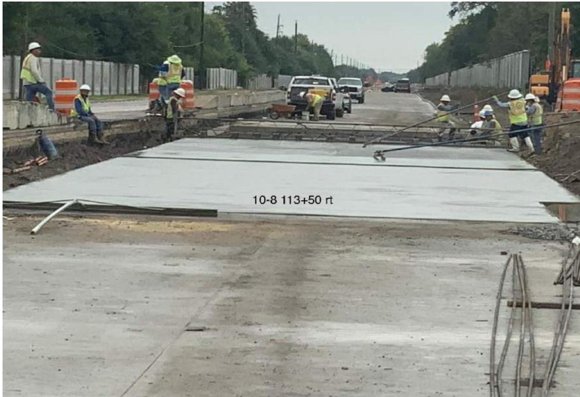
Pouring EB Hughes Ranch Road at May Ct.
