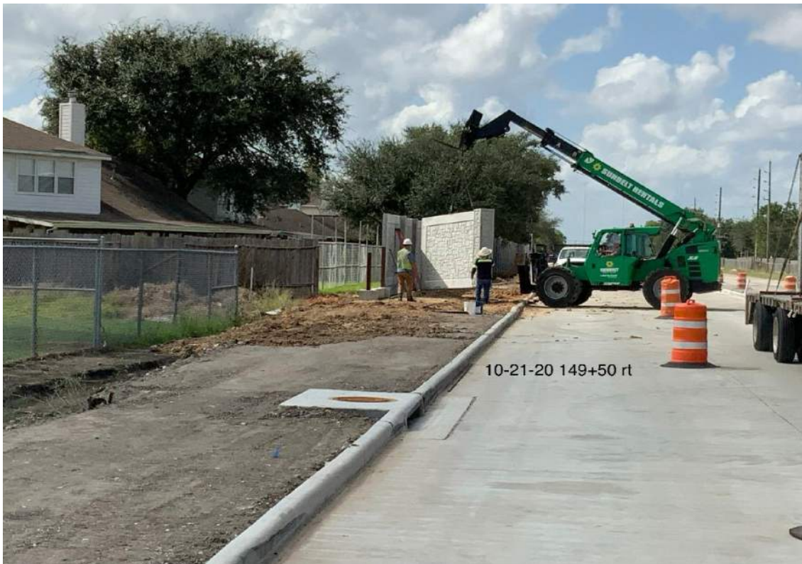
Erection of Wall H.
