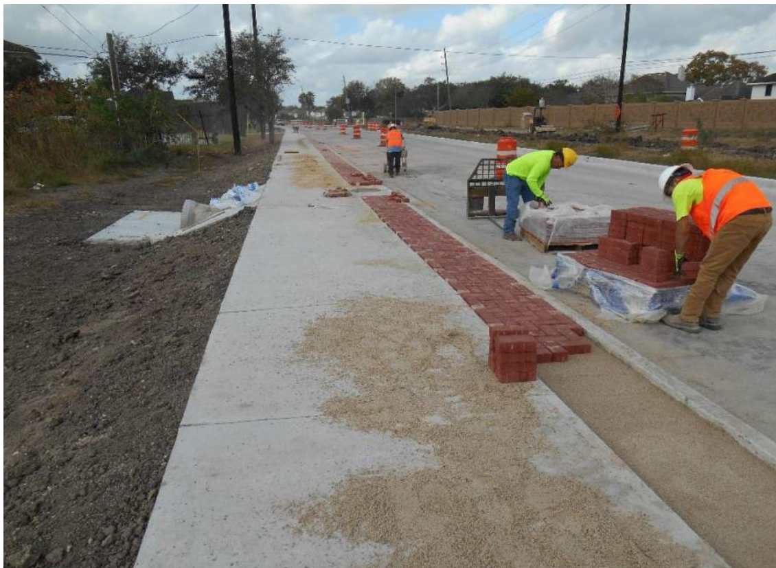
Installation of Brick pavers on south side of Hughes Ranch Road.
