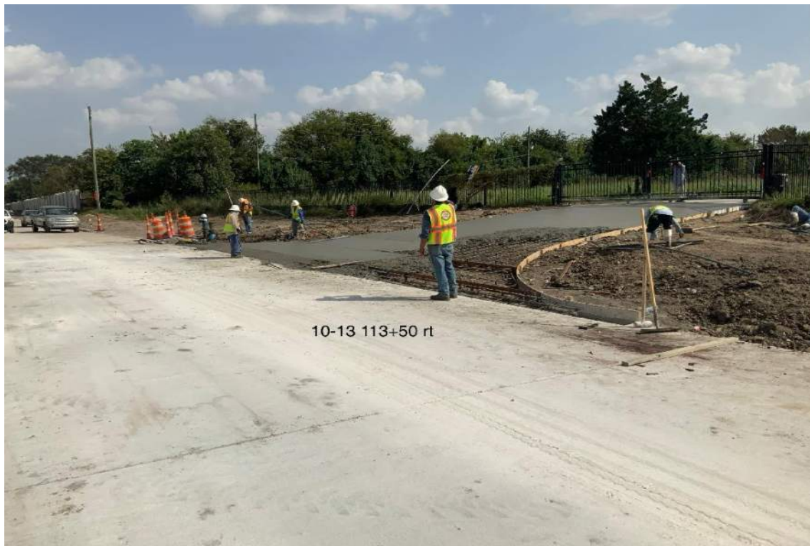
Pouring Intersection at May Court.
