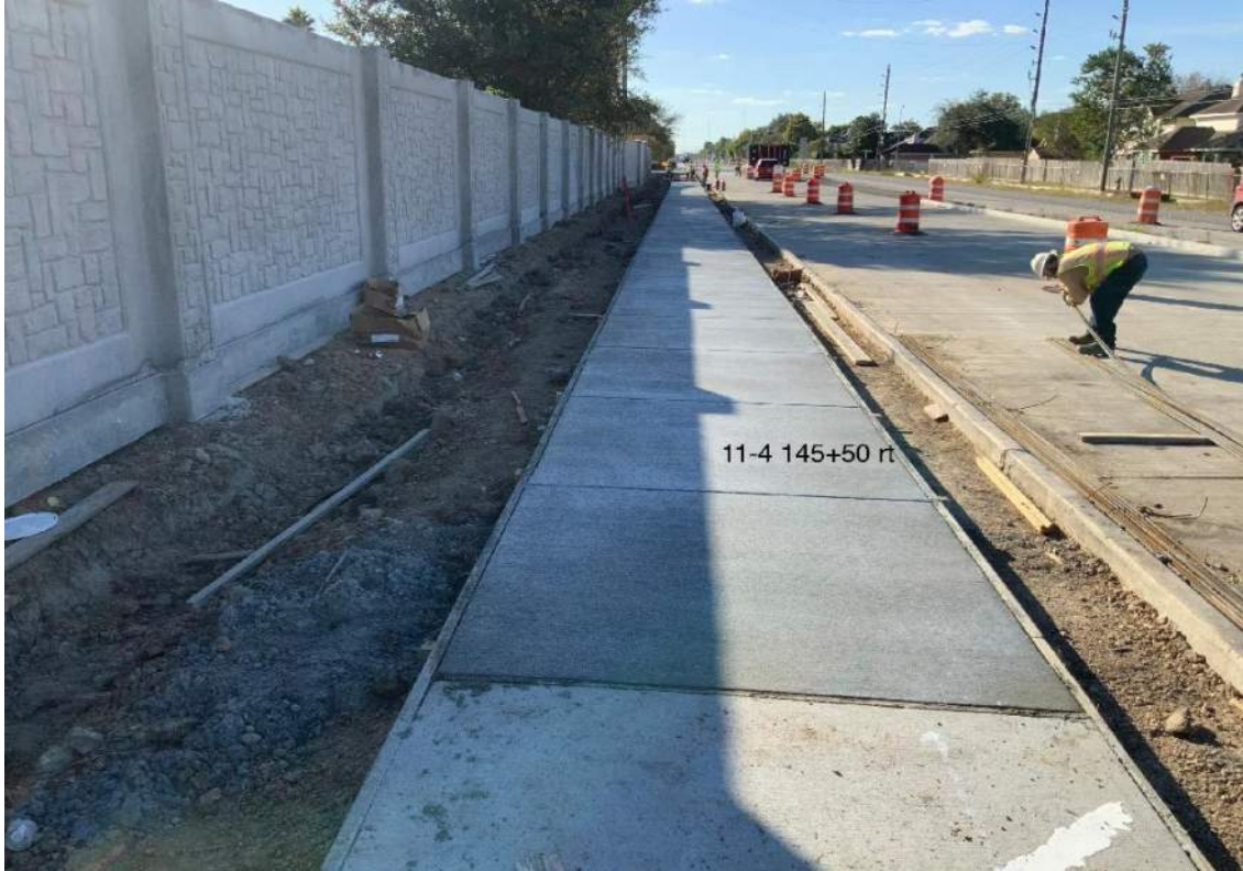
Sidewalk Construction along south side of Hughes Ranch Road.
