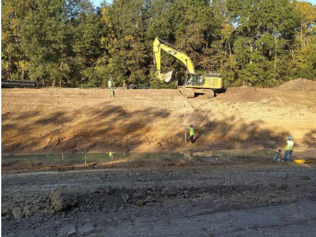
Excavation of Detention Basin #1
