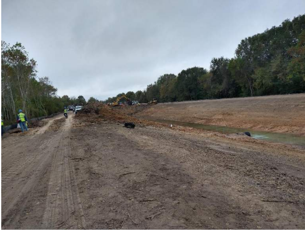
Clearing the Detention Basin
