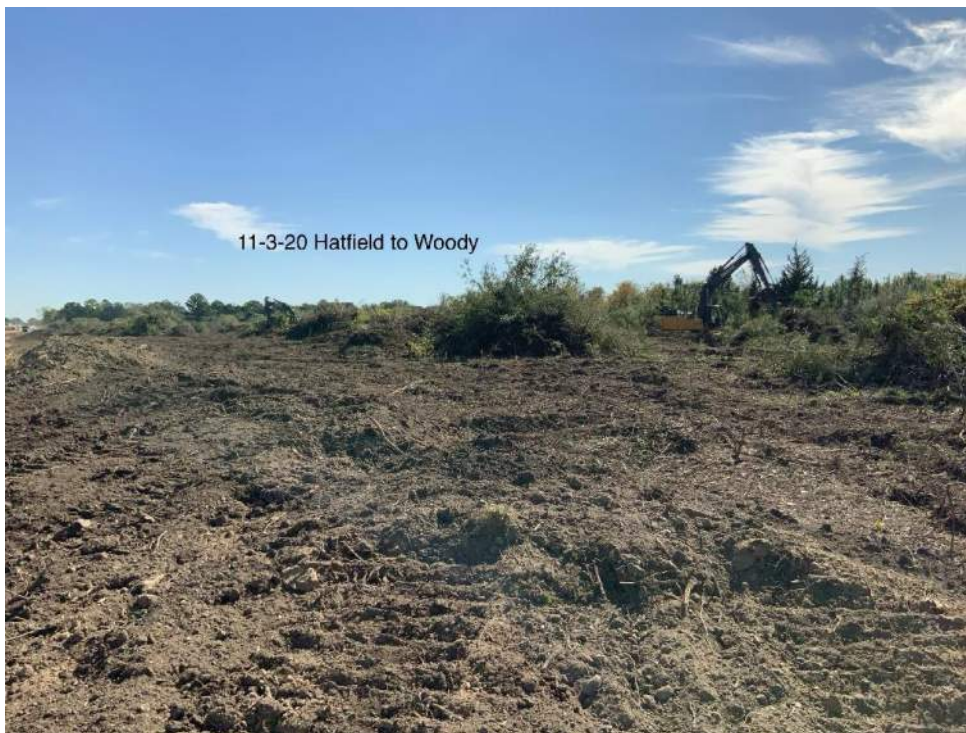
Clearing the Detention Basin
