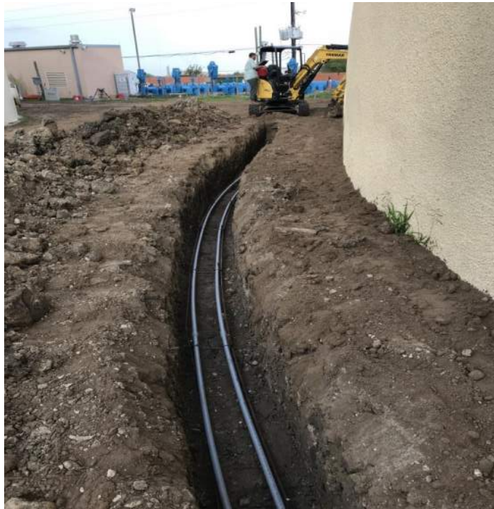
Ductbank install.
