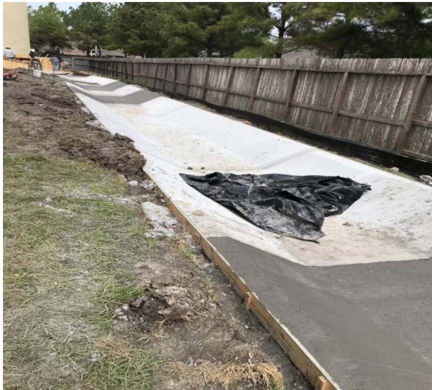
Concrete Spillway
