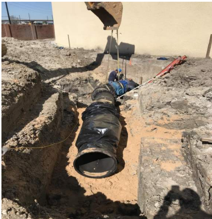
24" tie into the new tank
