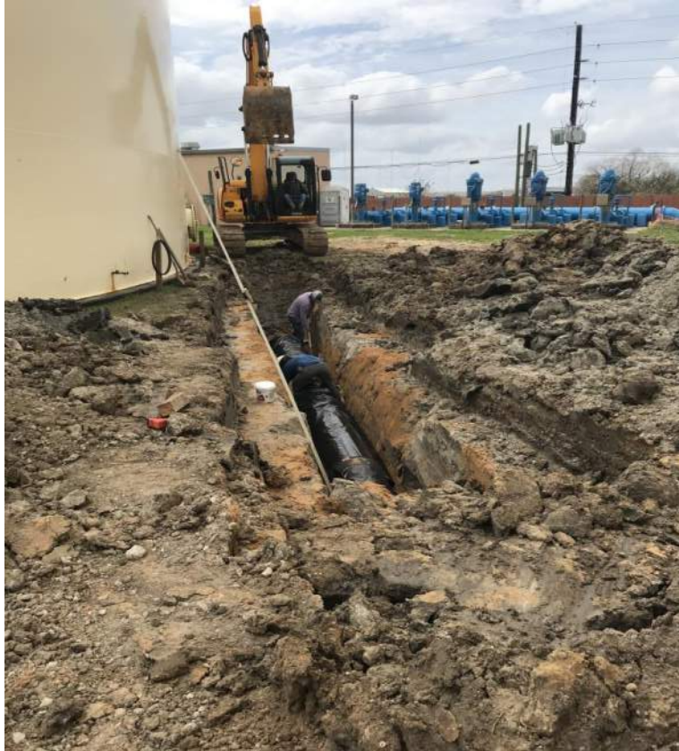
Trench and install 24" pipe.
