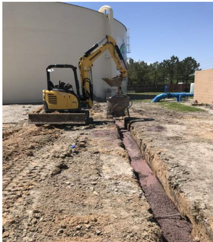
Placing red concrete
