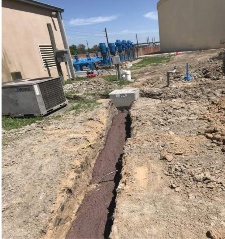
Red concrete and junction box.
