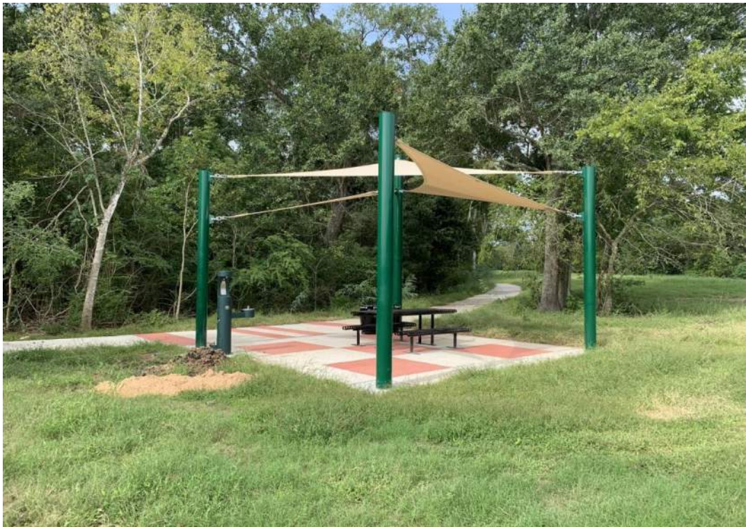
Amenity Structure w/ Water Fountain Installed
