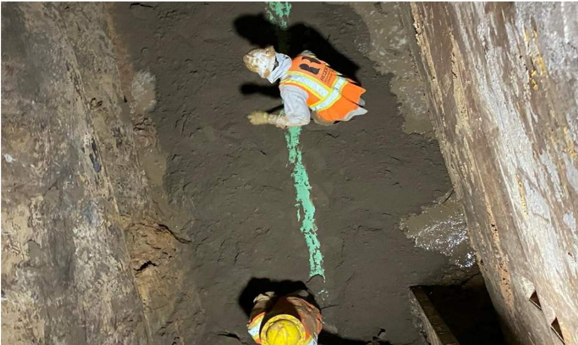
Recently installed 15" sanitary sewer being backfilled by cement stabilized sand.
