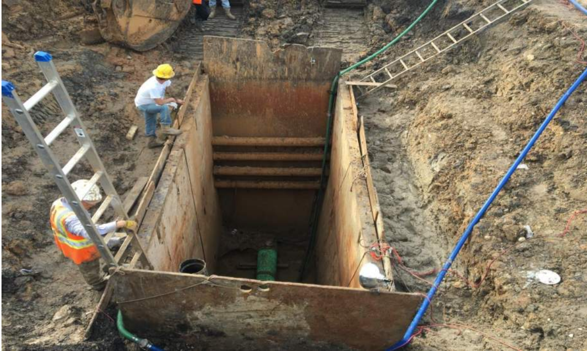
18" gravity sanitary sewer. Proper shoring and trench safety implementation.
