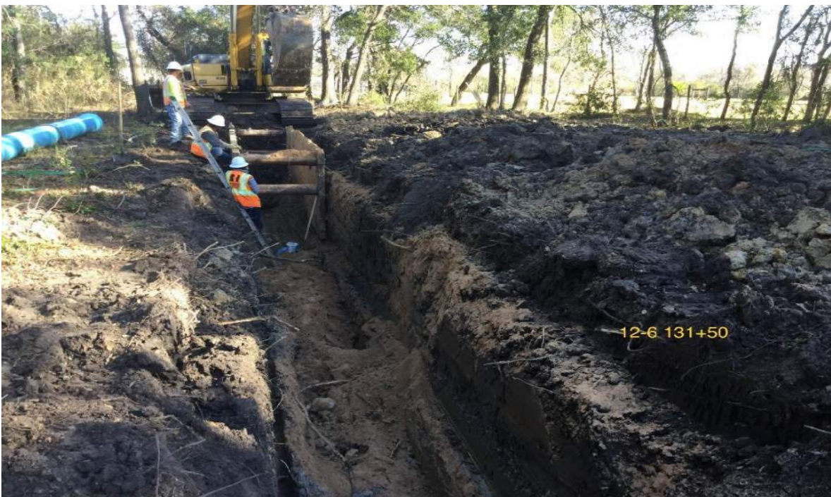
16" water line construction located in between O'Day Road and Hatfield Road.
