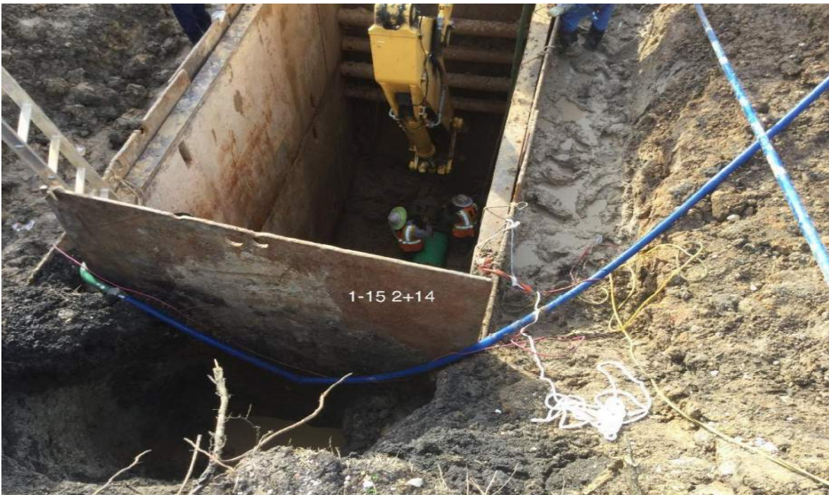
18" sanitary sewer installation. Avg. depth at this location, 26' depth.
