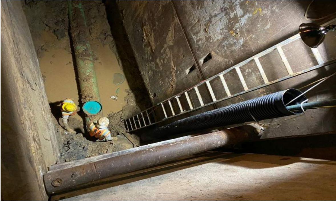
Recently bored 18" sanitary sewer at Cullen Blvd and McHard Road.
