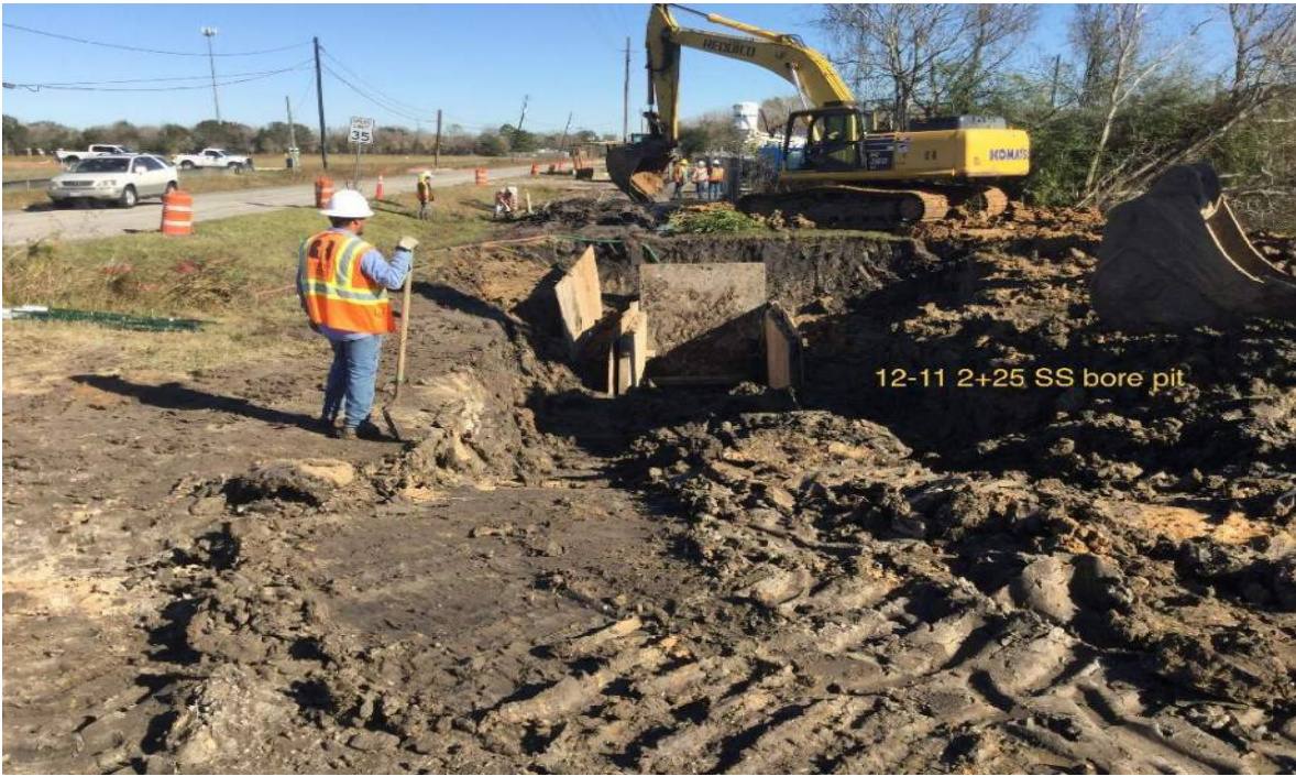
Bore Pit preparation for proposed 18" sanitary sewer line.
