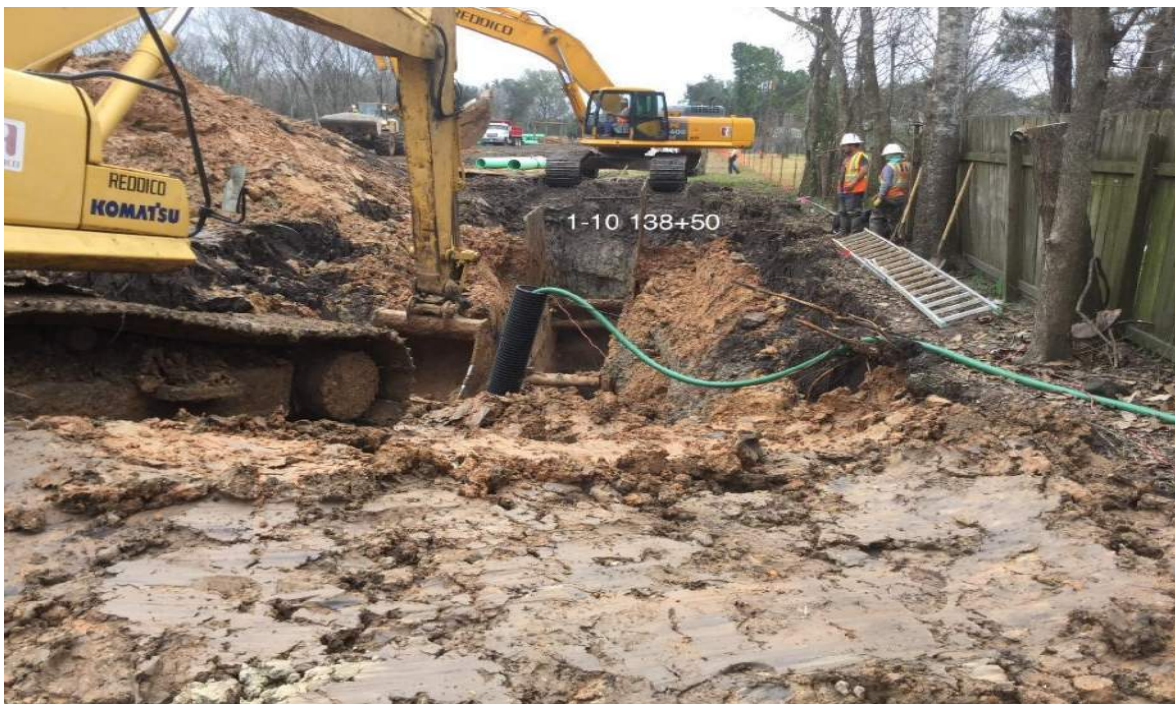
Sanitary sewer trench – dewatering bottom of trench.
