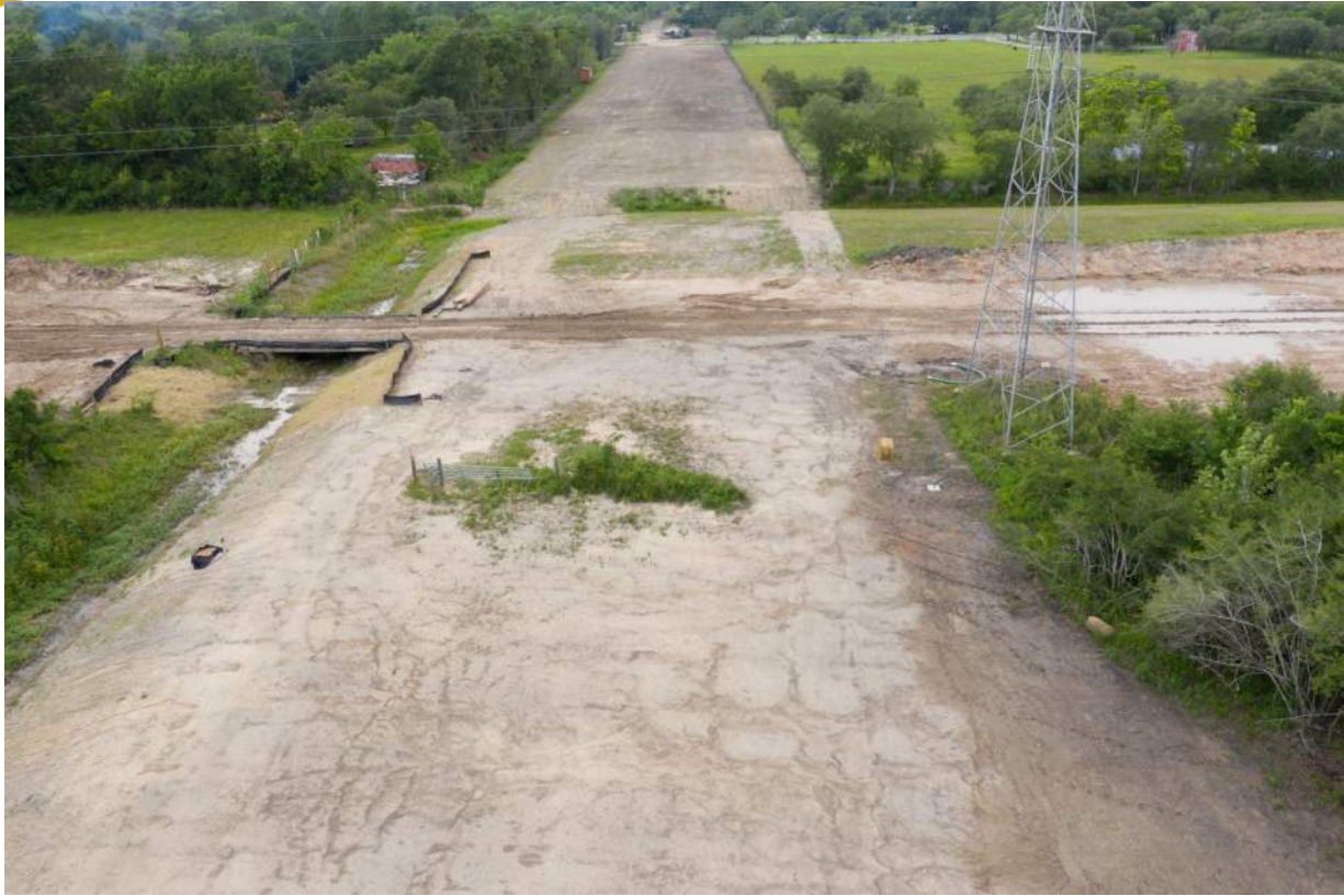
View looking down the cleared McHard Road corridor
