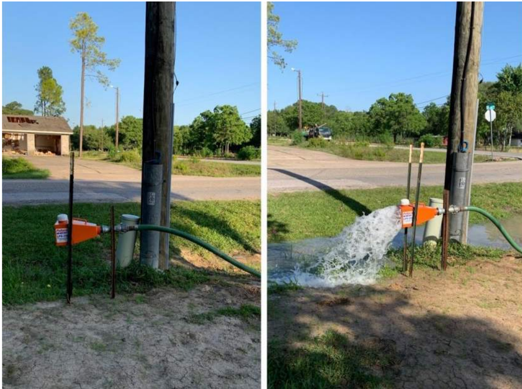
Flusing the 16" Water Line
