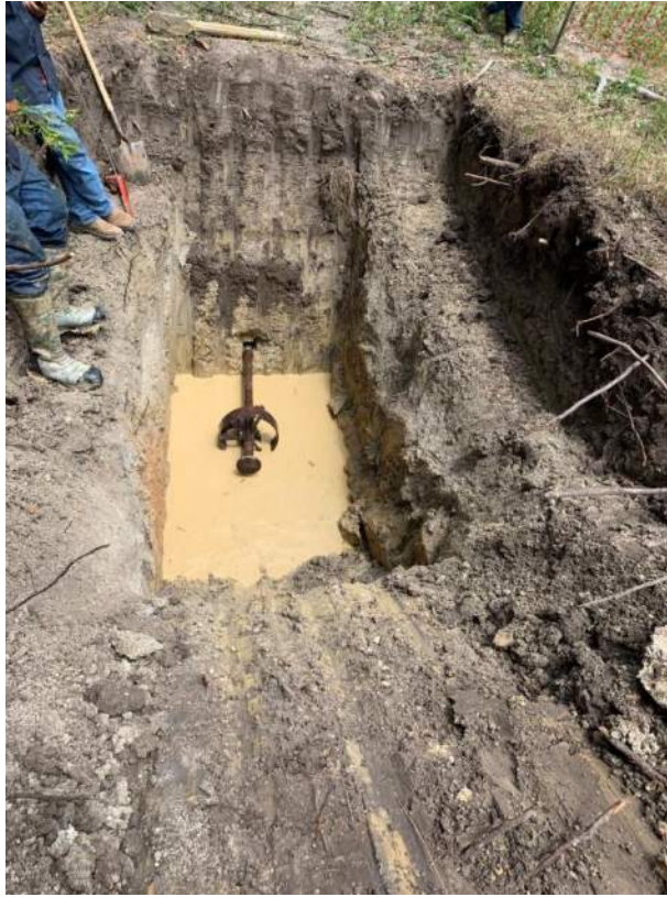
Pilot Head for 16" Directional Bore
