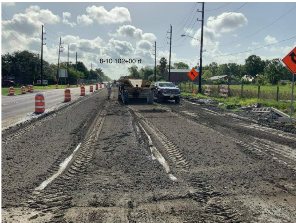
Construction of subgrade just east of Smith Ranch Road.
