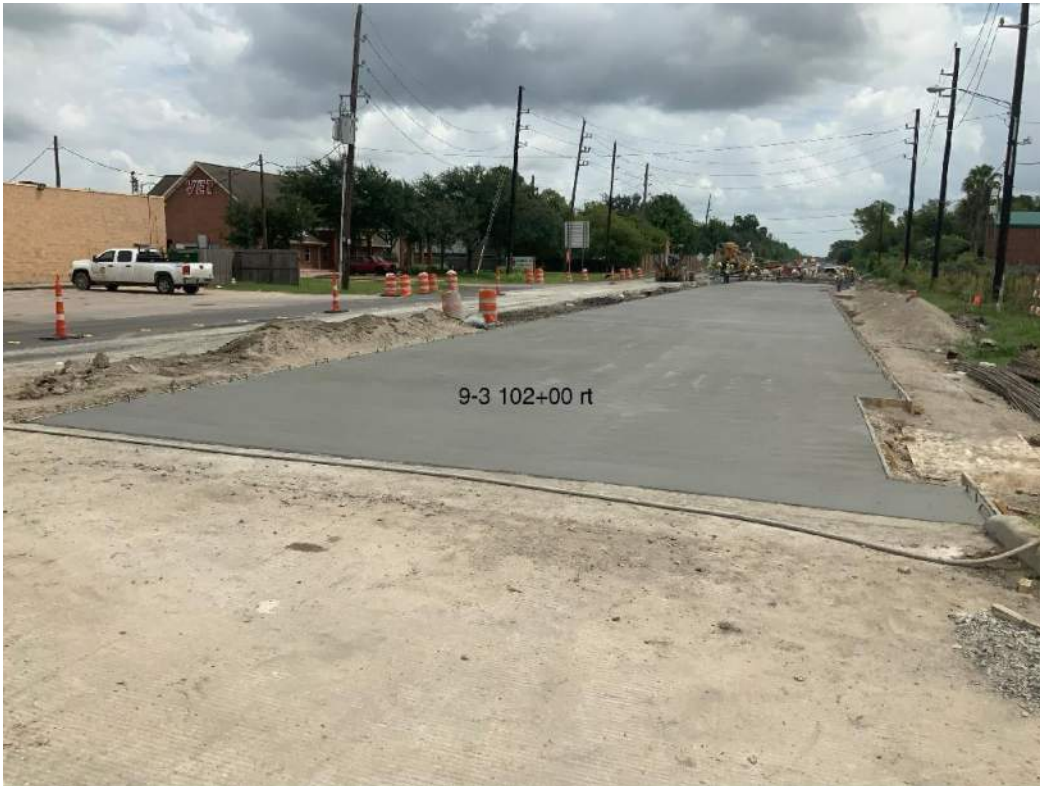
Construction of EB Hughes Ranch Road at Smith Ranch Road.
