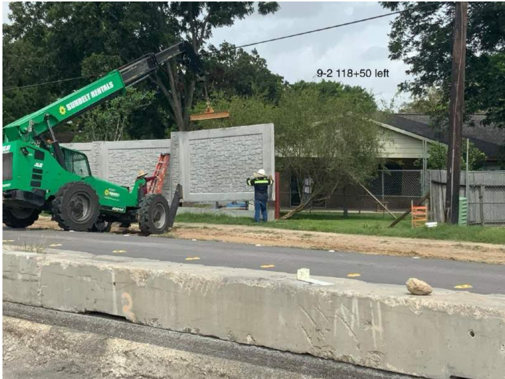
Erection of Sound Wall B.
