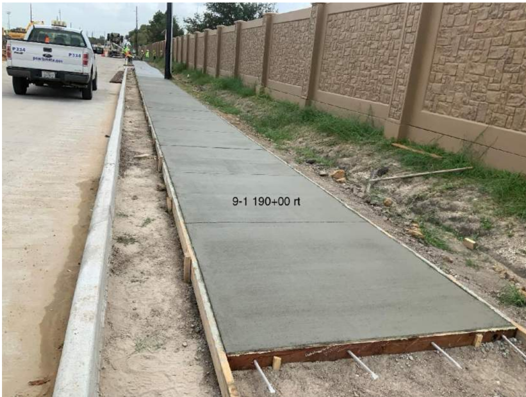
Sidewalk construction on south side of Hughes Ranch Road.
