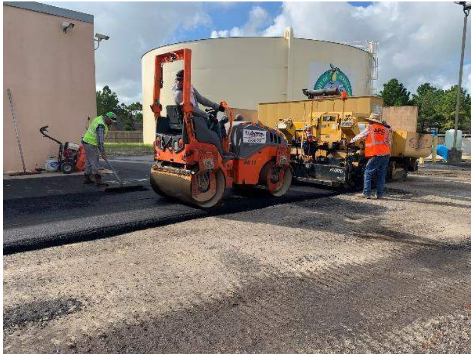
Placing asphalt and compacting it in using a roller
