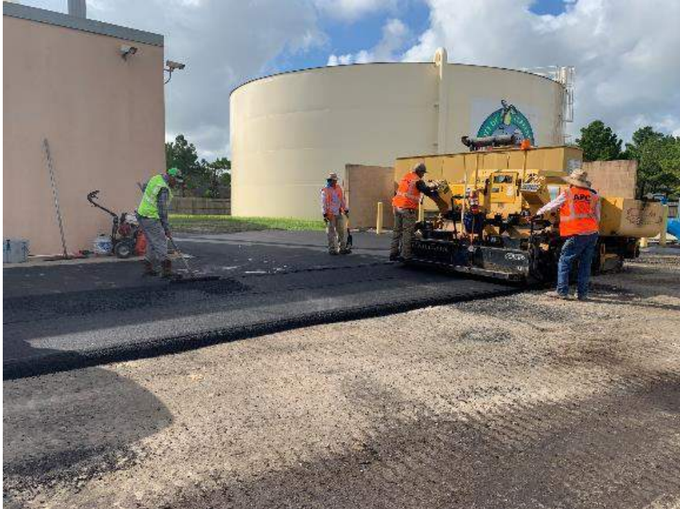
Installing Asphalt
