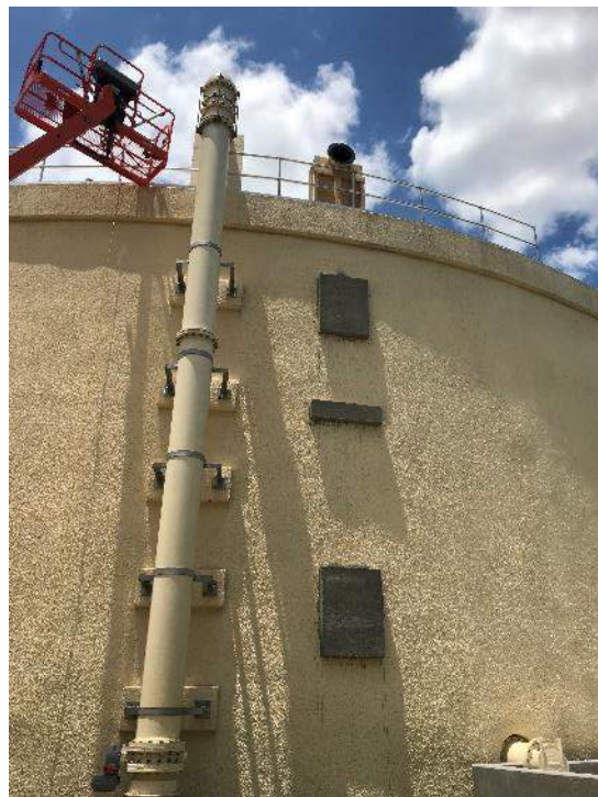
Embeds on the tank to install new 16" riser pipe.
