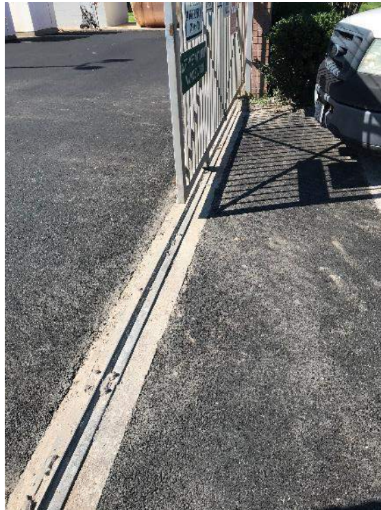
Gate track asphalt transition
