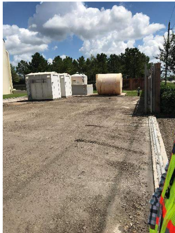
Base for the parking lott
