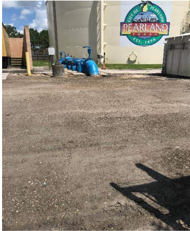
Parking lott cement base placed before asphalt
