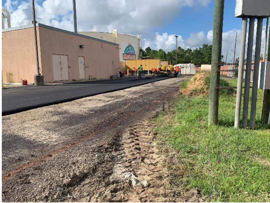
Placing asphalt lifts
