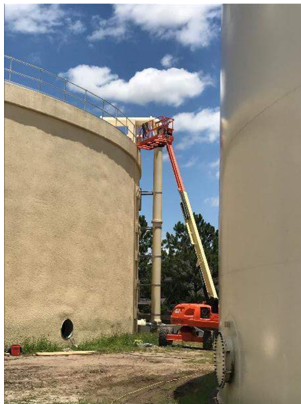
Installing 16" riser pipe for water from Surface Water Plant
