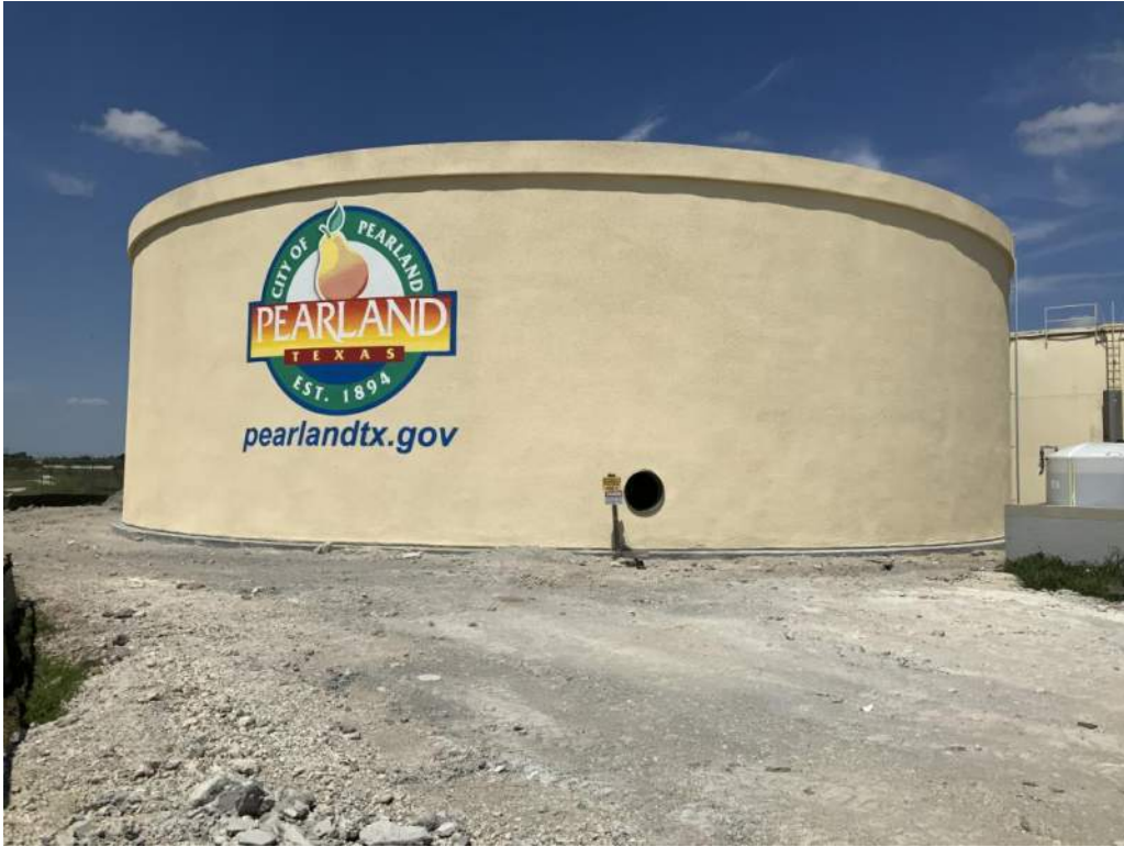
Phase I Completed Tank
