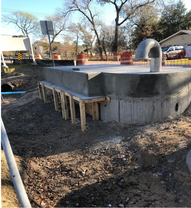
Poured in place lift station hatch
