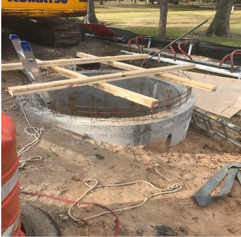
Wet Well installed
