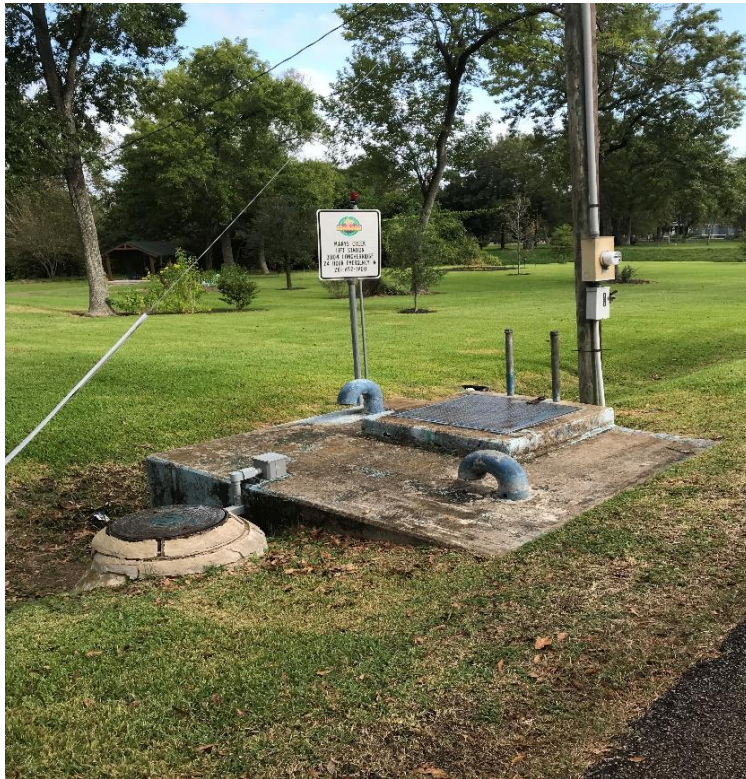
Existing Lift Station
