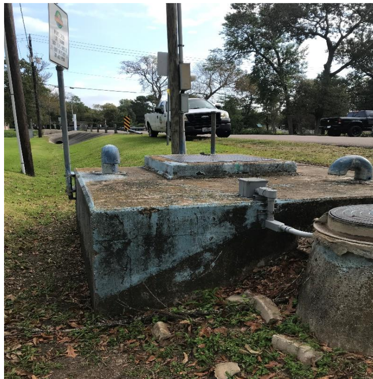
Existing Lift Station
