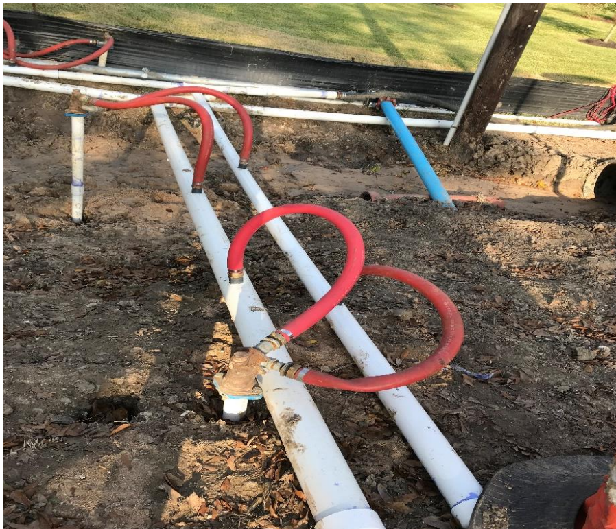
Well pointing system
