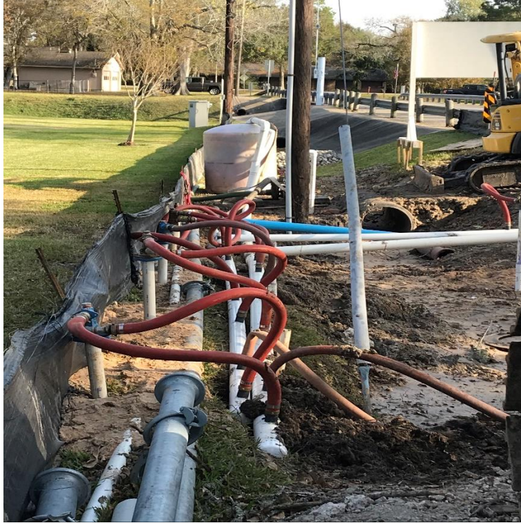
Well Pointing System
