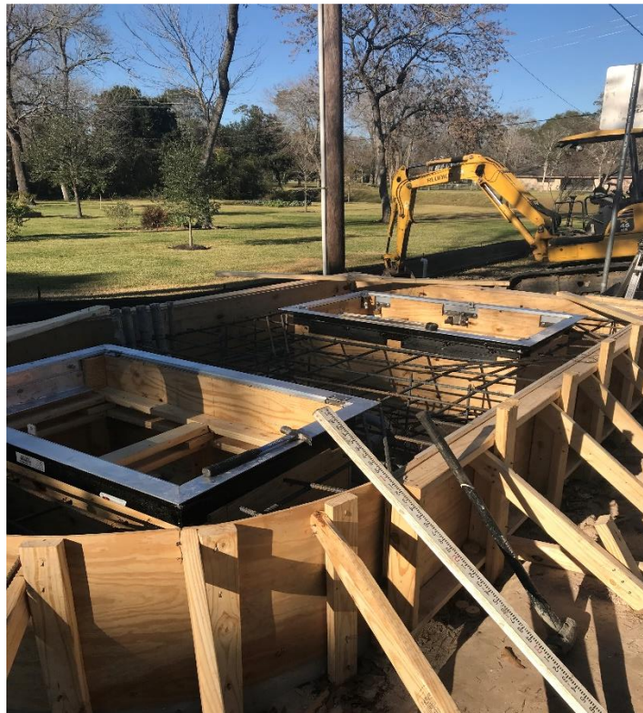
Form work for lift station hatch entrances
