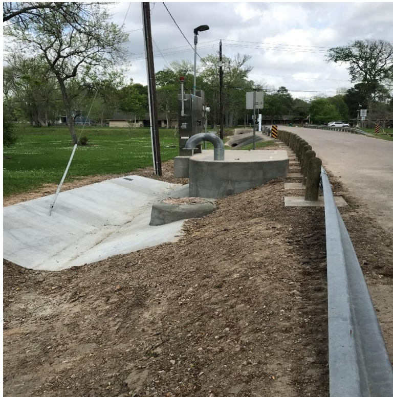
Slope paving and Guardrail
