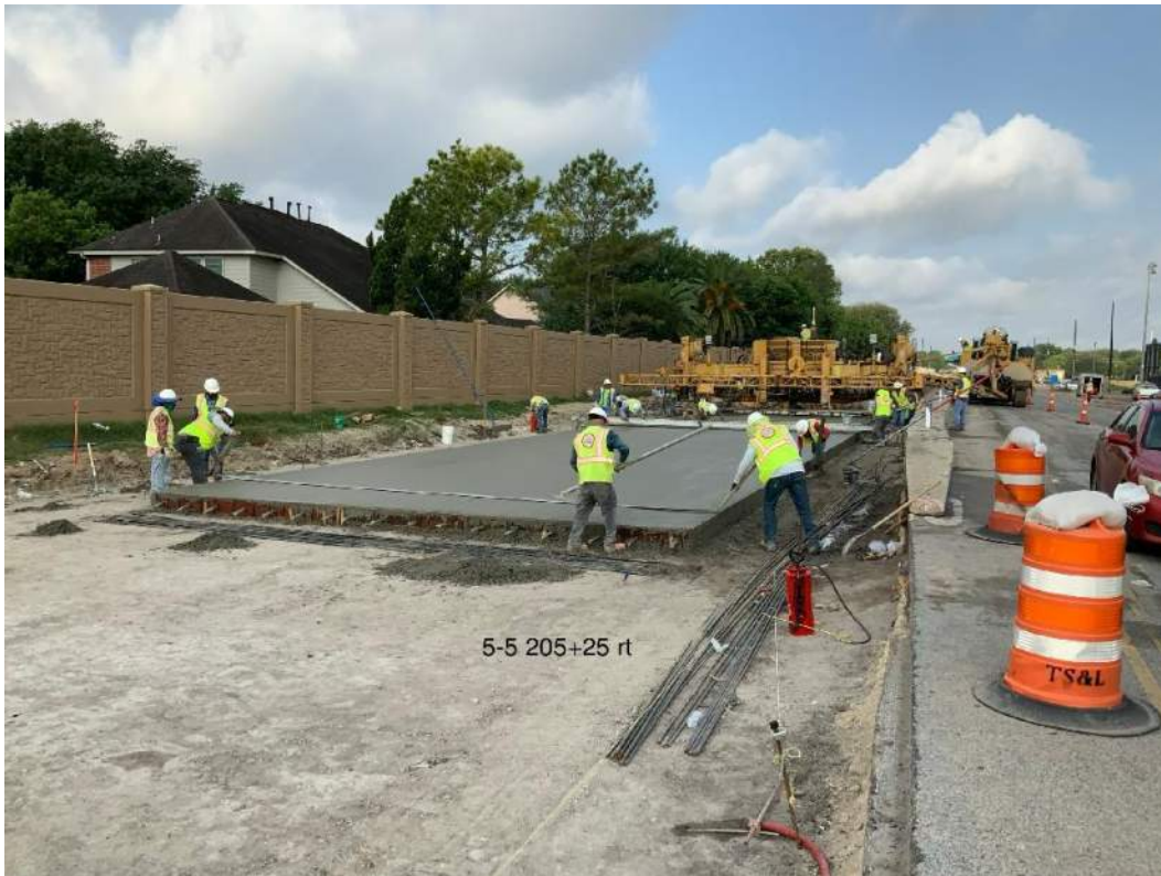
Concrete paving commences on east end of the project.
