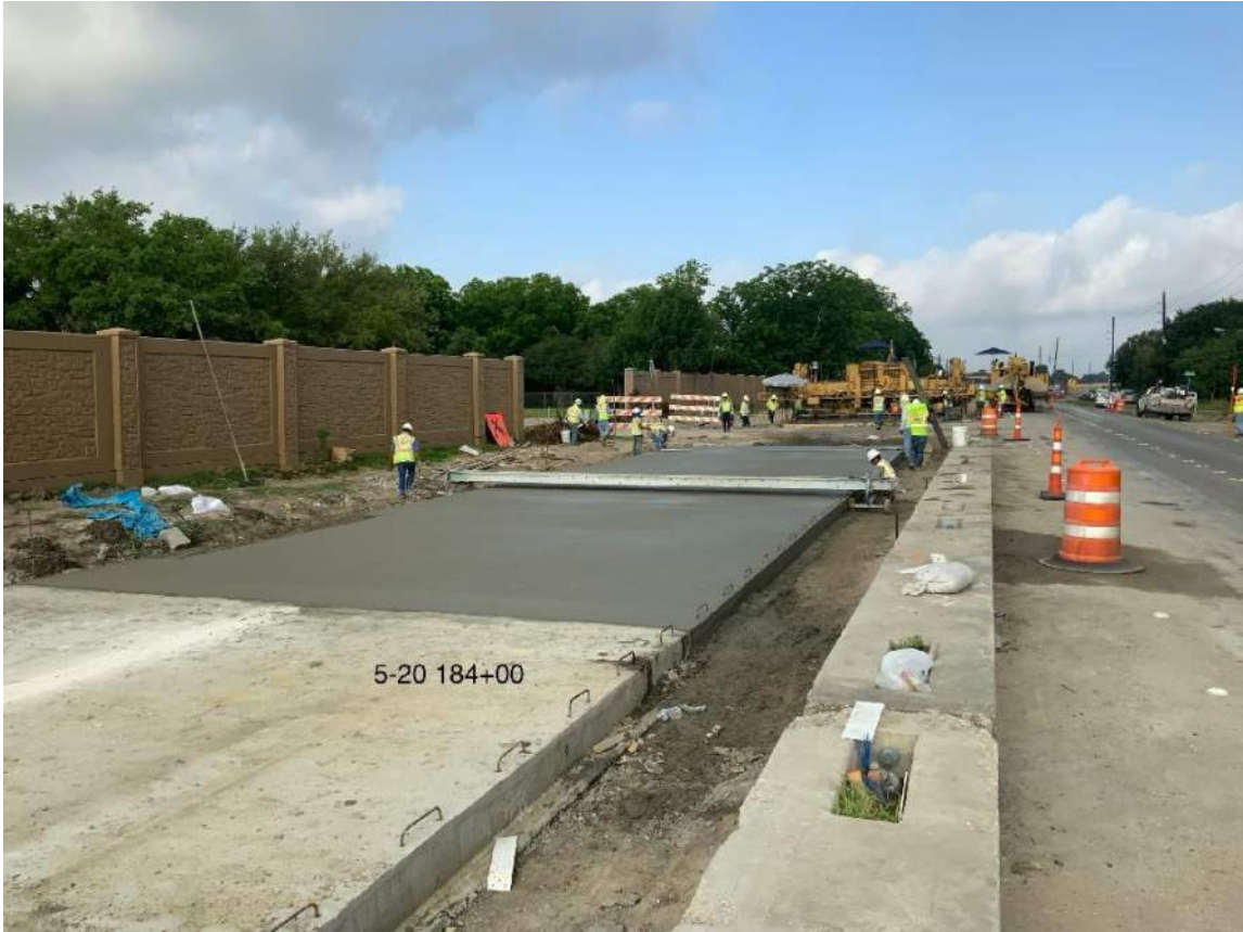
Concrete paving construction progresses past entrance to Crystal Lakes.
