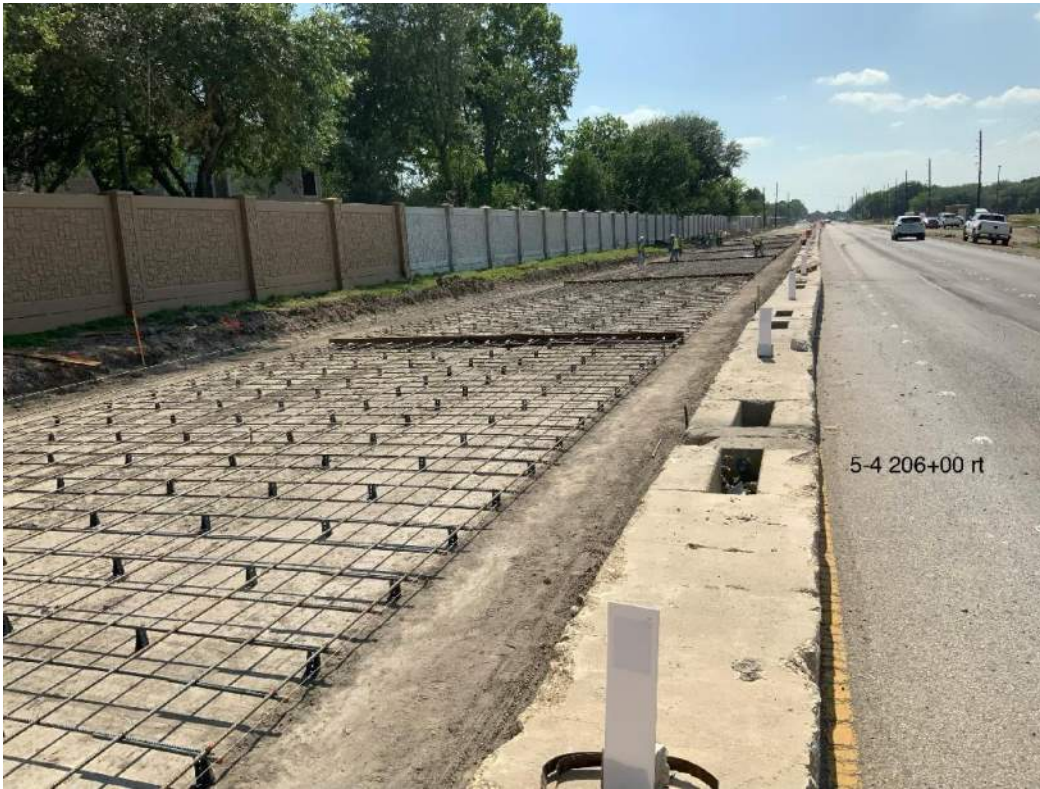
Steel reinforcement and expansion joints placed near Cullen.
