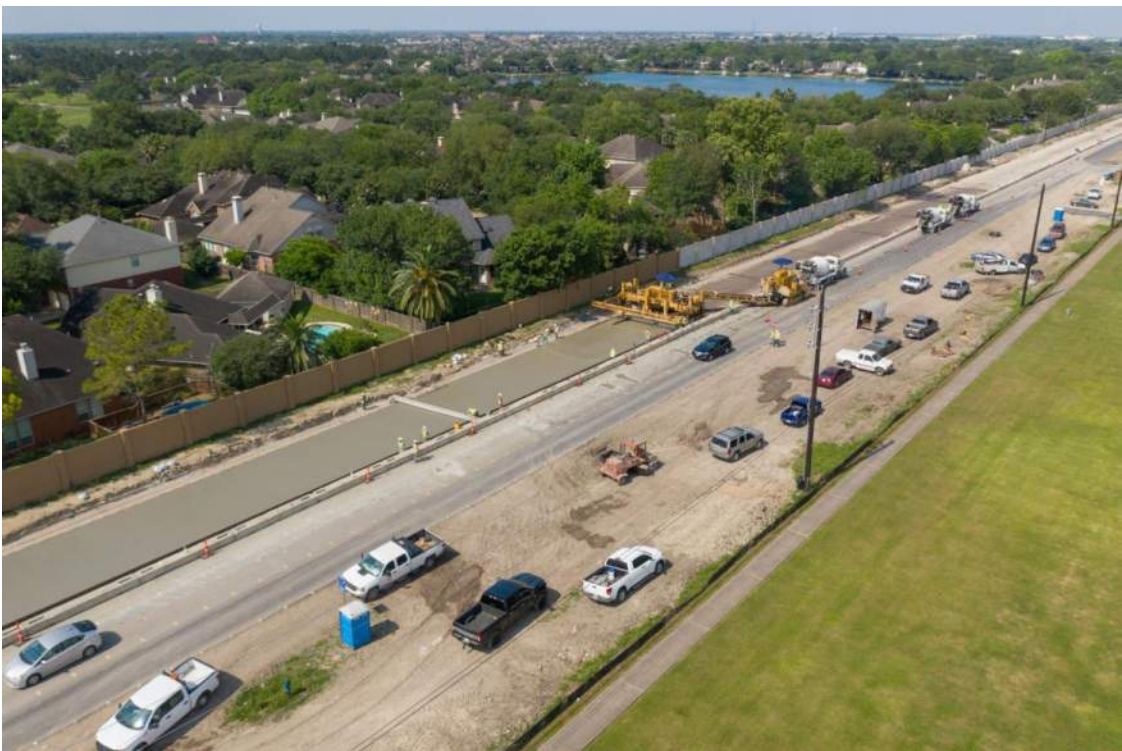
Concrete paving construction progresses fronting Crystal Lakes.
