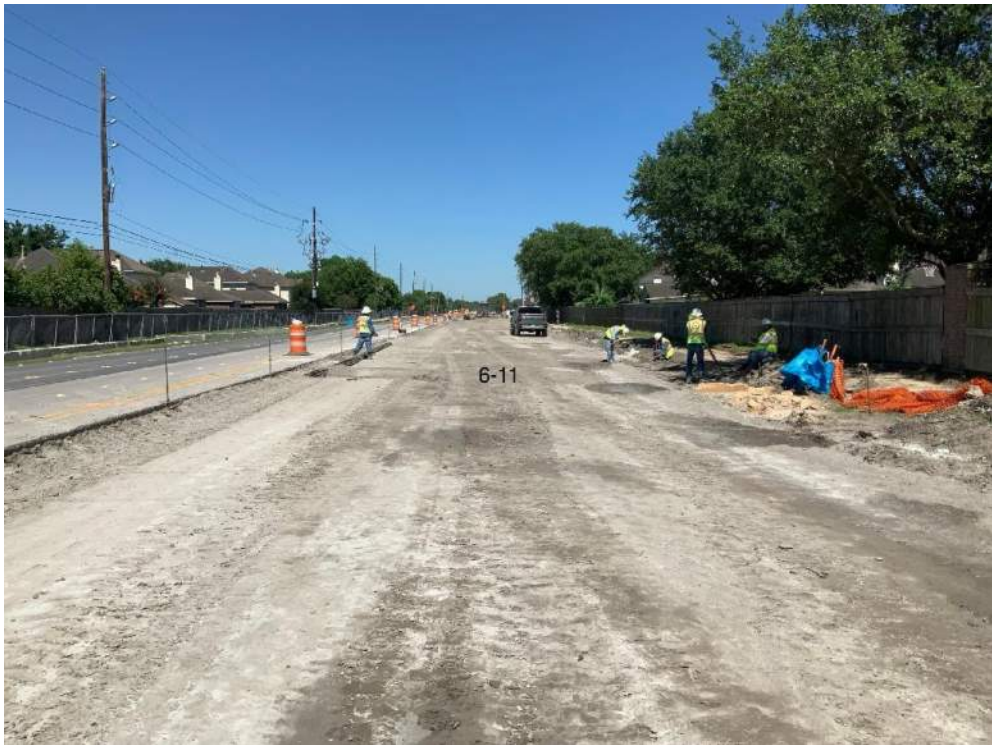
Setting stringline for paving machine.
