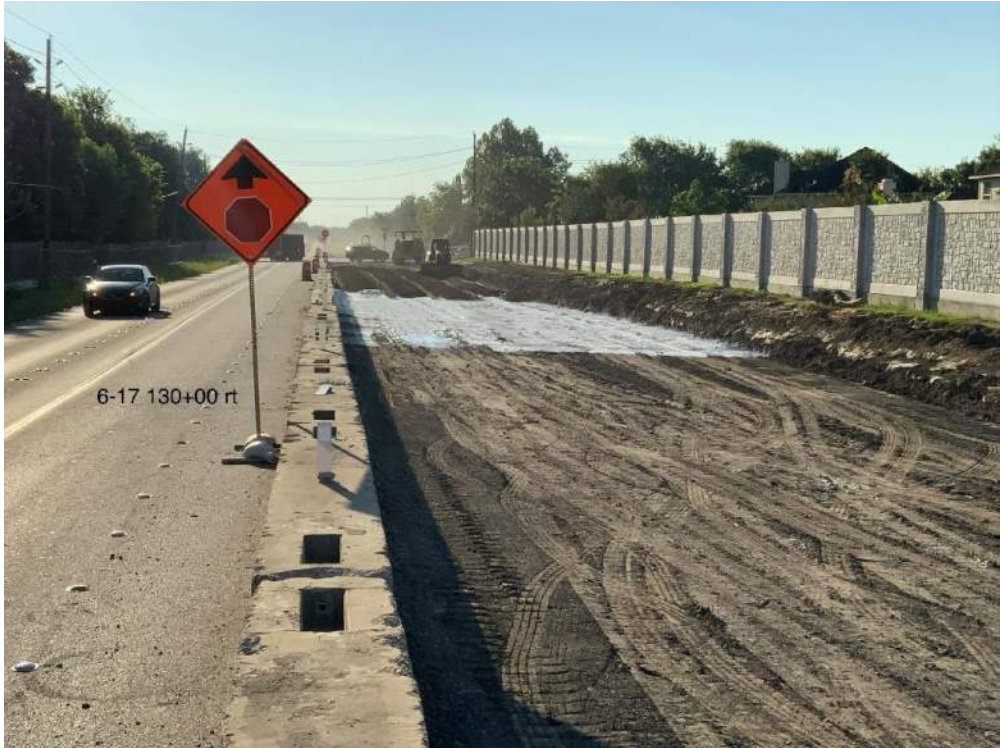
Lime Treatment of pavement subgrade.
