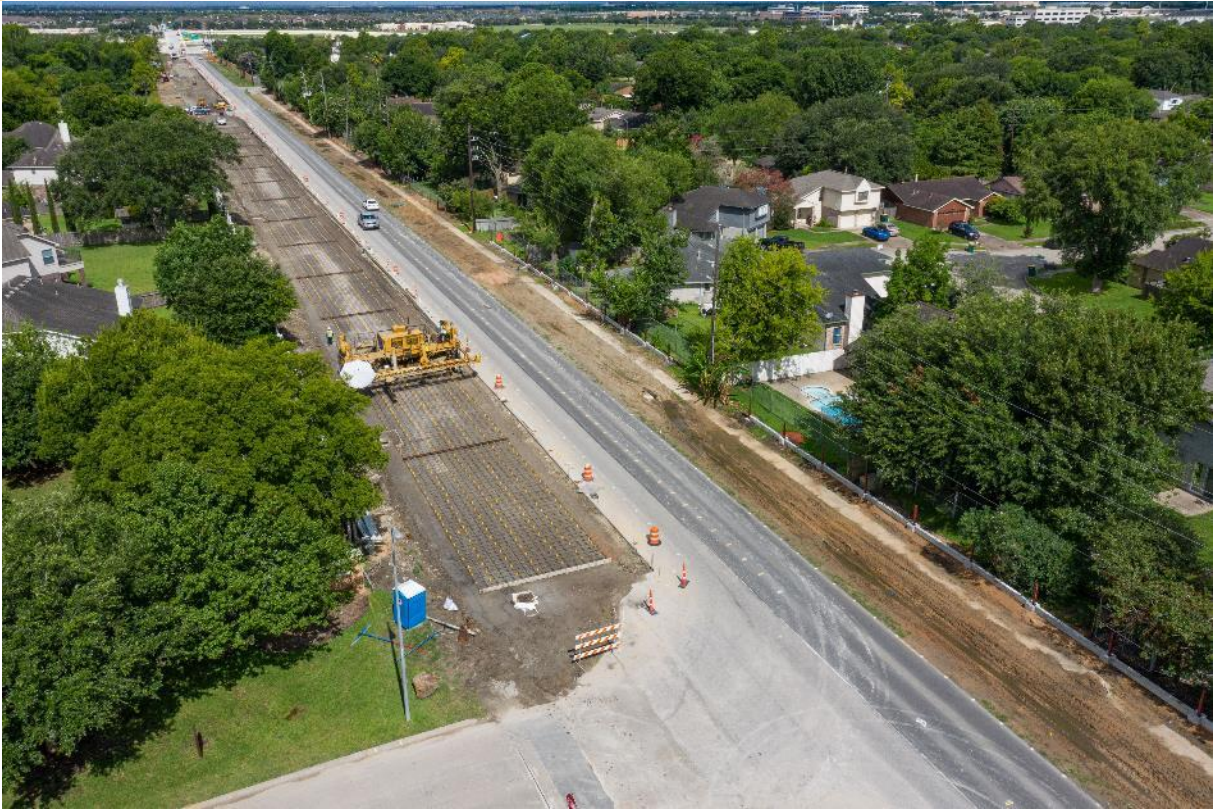
View of Project Looking West to Smith Ranch Road and SH288
