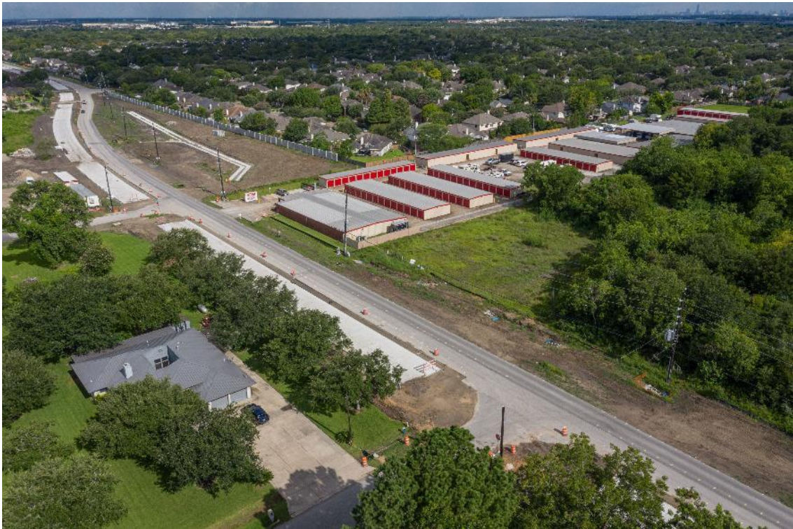
View of Project Looking Northwest
