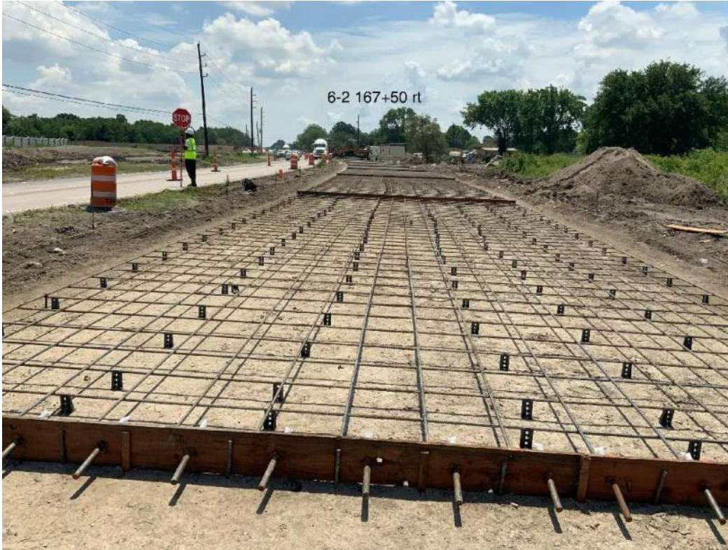
Steel reinforcement and expansion joints in place.
