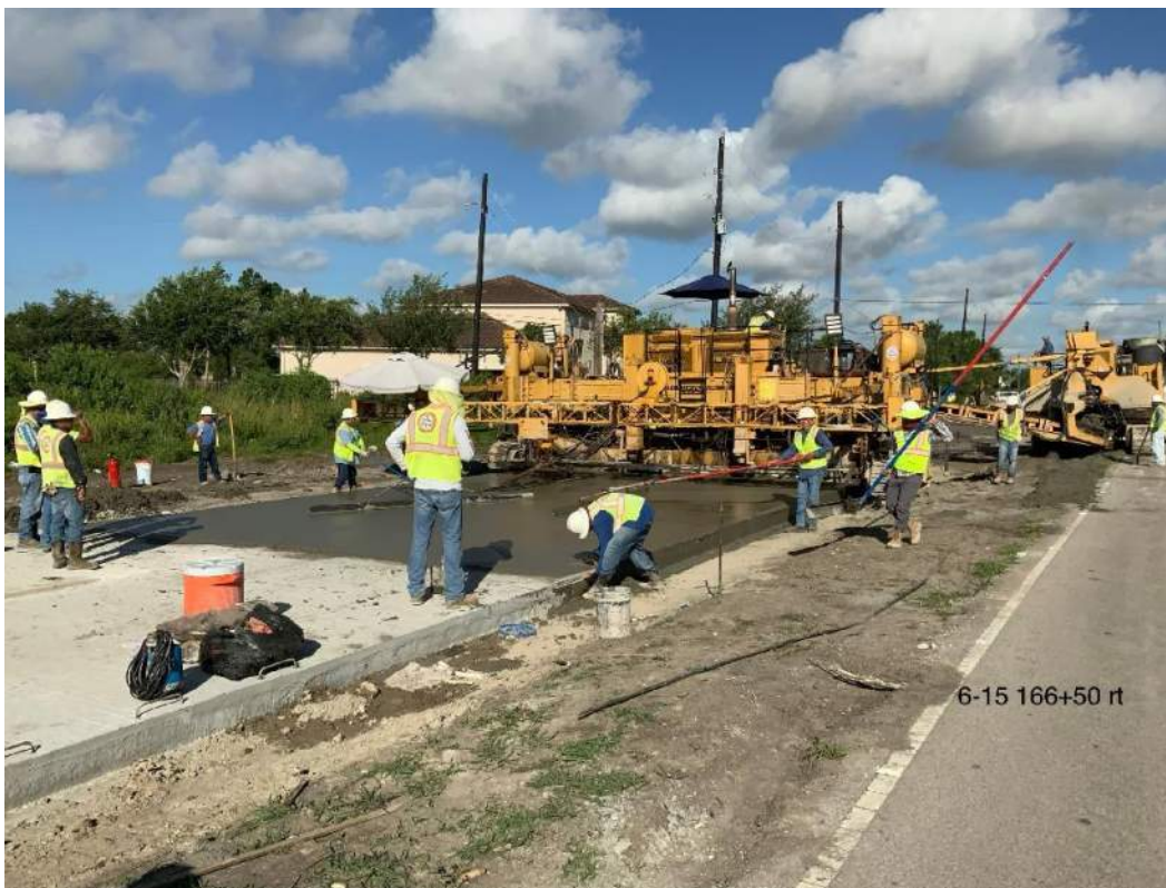
Slip form concrete paving construction.
