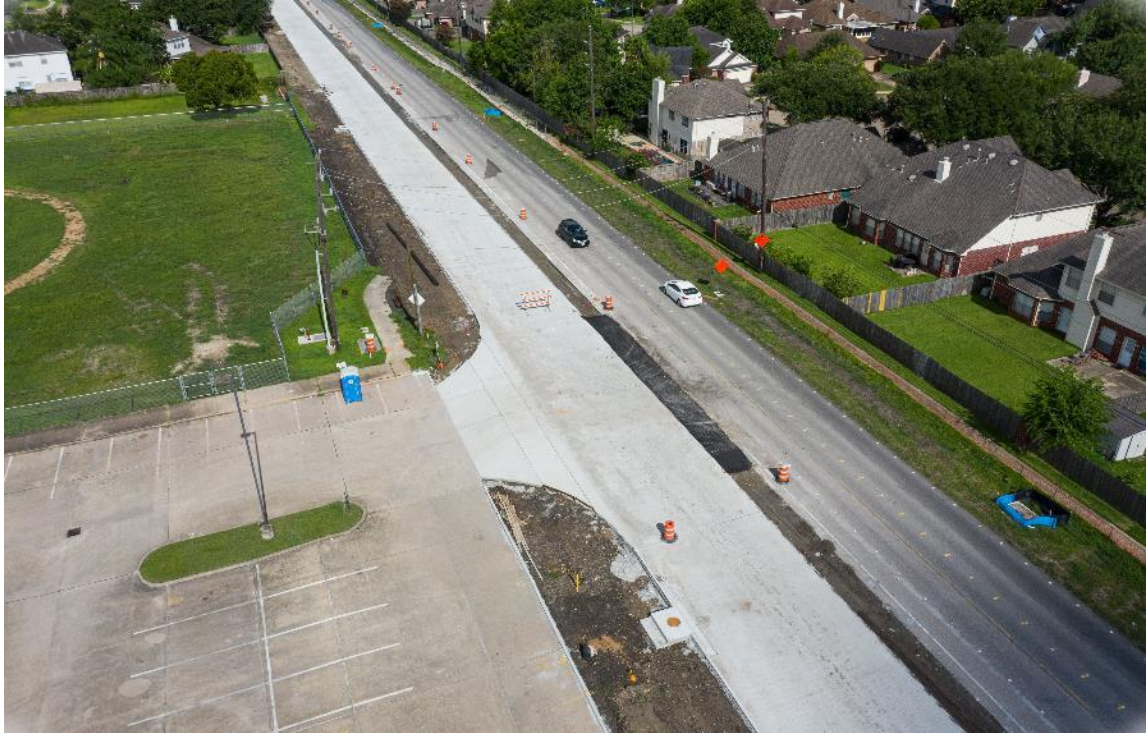
View of Project Looking at Challenger Elementary driveway tie-in
