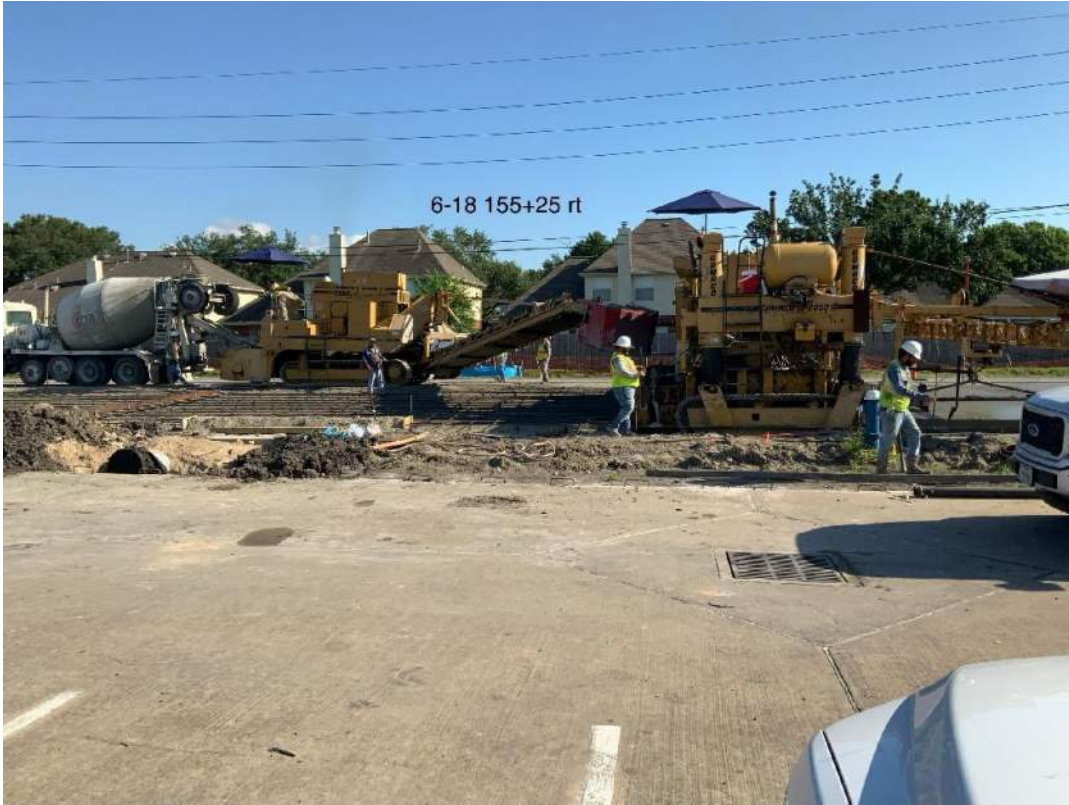
Slip form paving process
