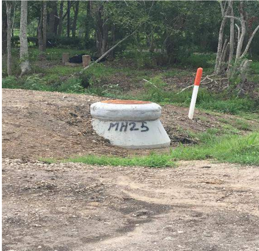
Manhole to grade and exterior grouted.
