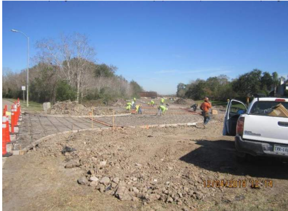
Setting steel for parking lot at Pearland Parkway
