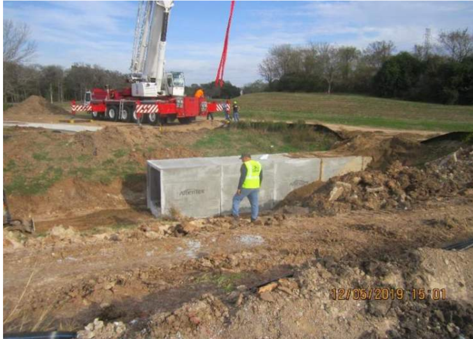
6X6 box installation at drainage ditch outfall to Clear Creek
