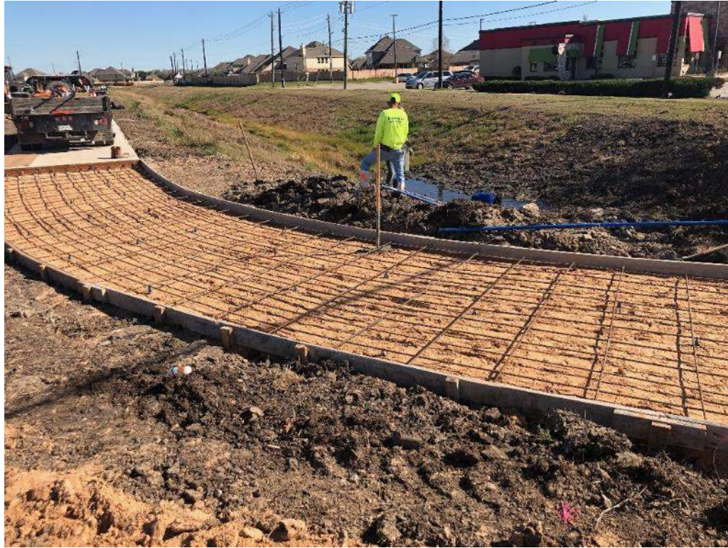
Steel placement at FM 518
