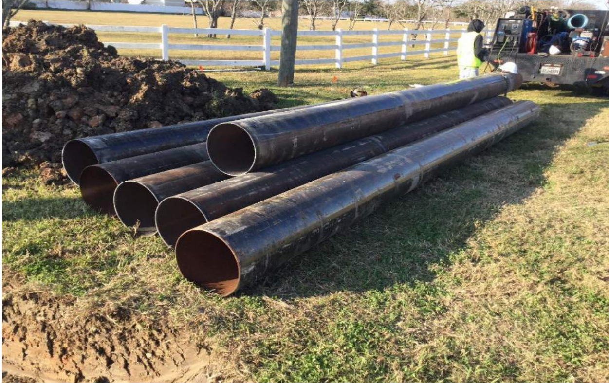
Steel casing for the bore under Magnolia Parkway.
