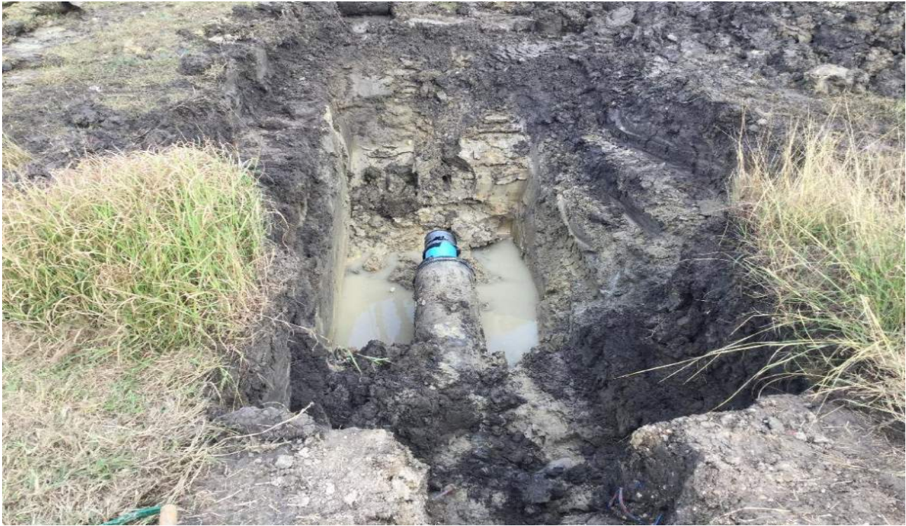
8" PVC water line being pushed in through the steel casing.
