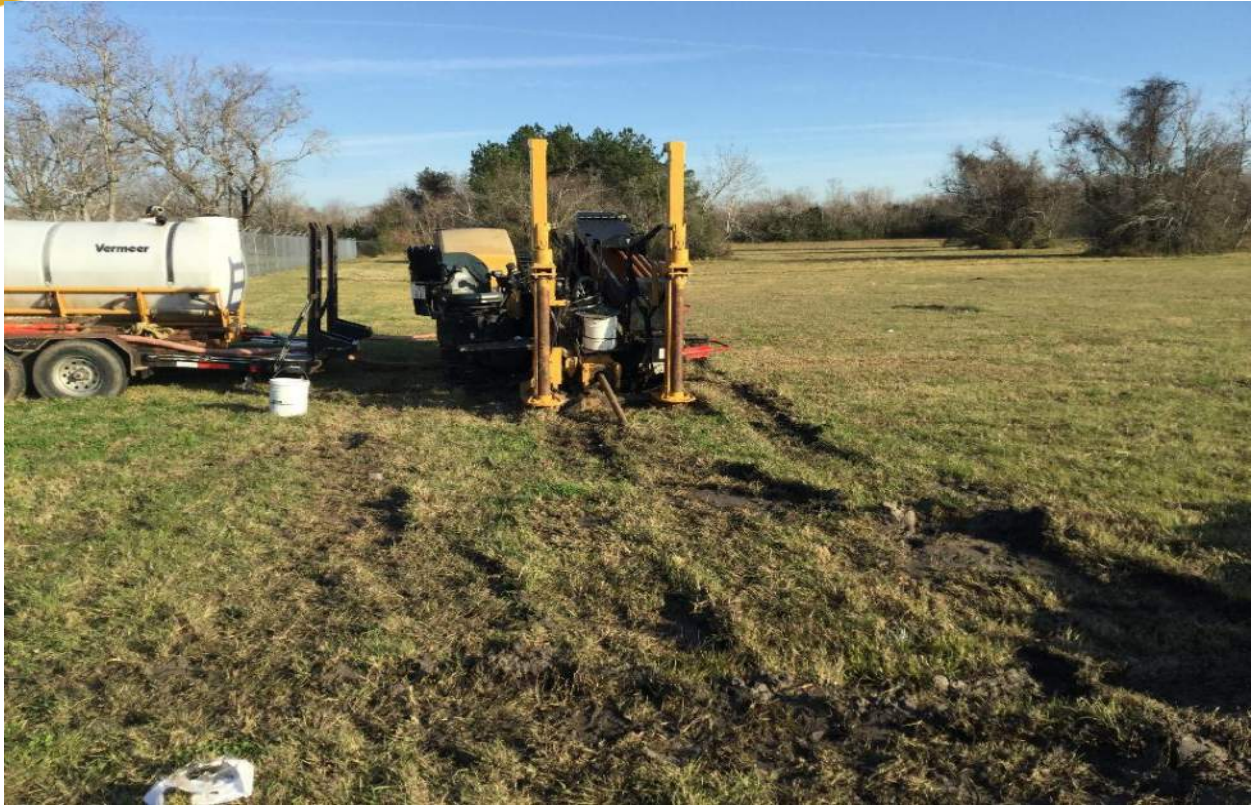
Boring rig on site.
