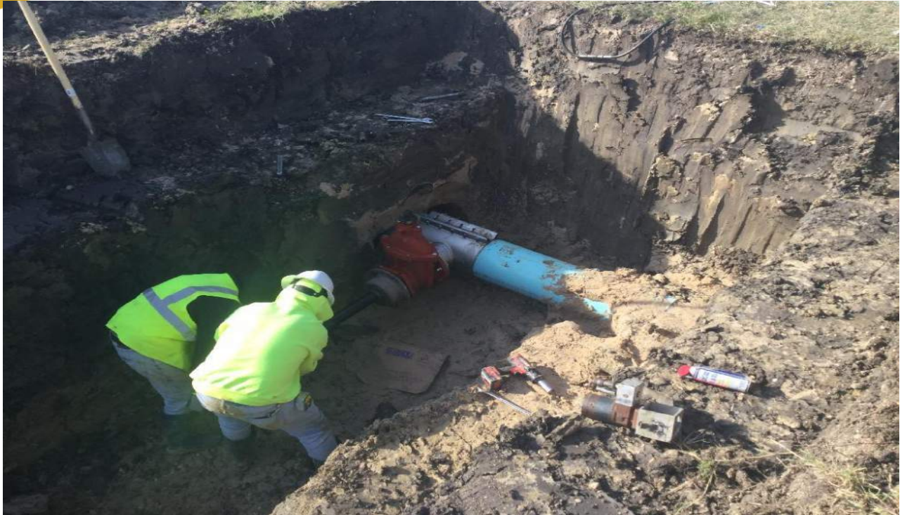
12" x 8" tapping sleeve and valve (TSV) located off of Magnolia Parkway.
