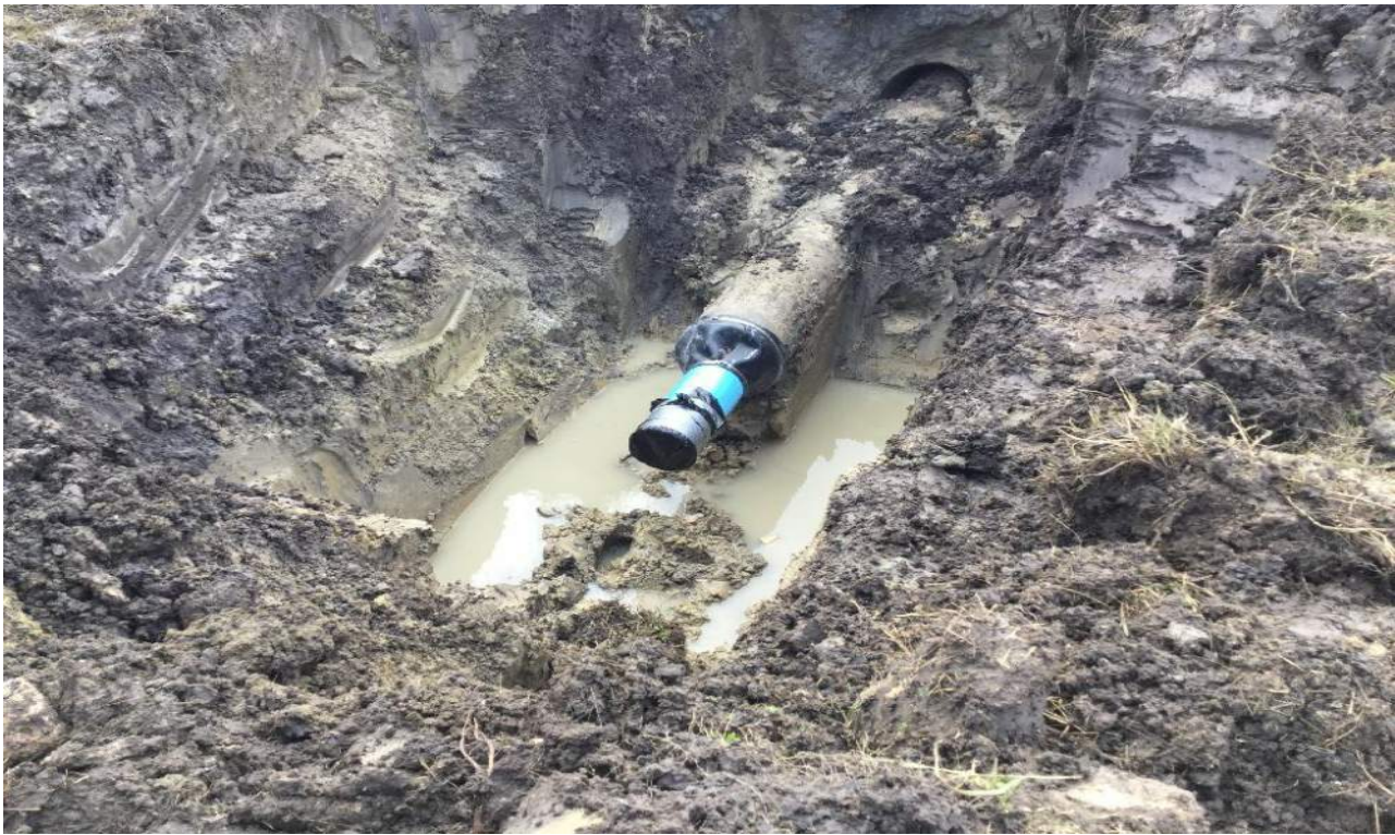
8" PVC water line complete in place through steel casing.
