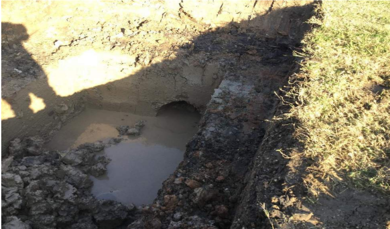
Test pilot bore – prior to pushing steel casing through.
