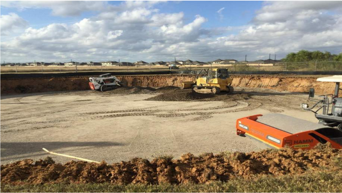
Grading and compacting TXDOT Flex-base.
