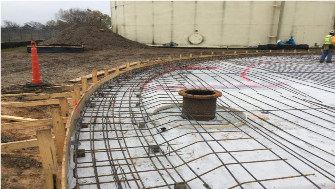
Depiction of rebar setting sequence for the perimeter footing.
