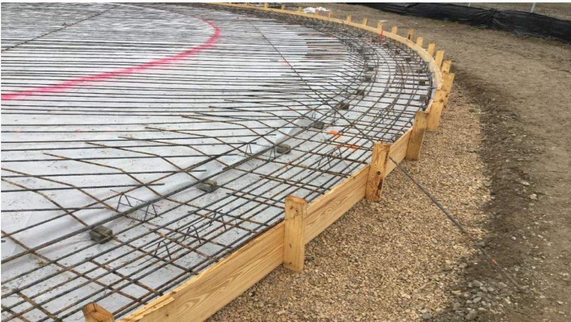
Depiction of rebar setting sequence for the perimeter footing.
