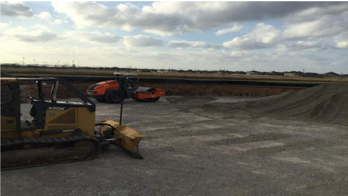
Grading and compacting TXDOT Flex-base.
