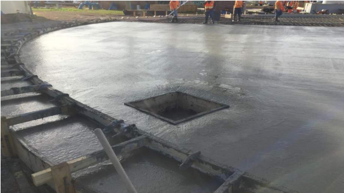
Post concrete pour. Slab is under water for optimum curing.
