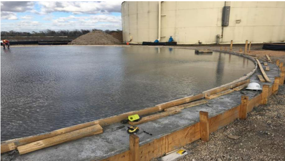
Post concrete pour. Slab is under water for optimum curing.
