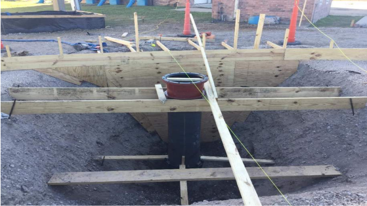
18" ductile iron piping encased in concrete.
