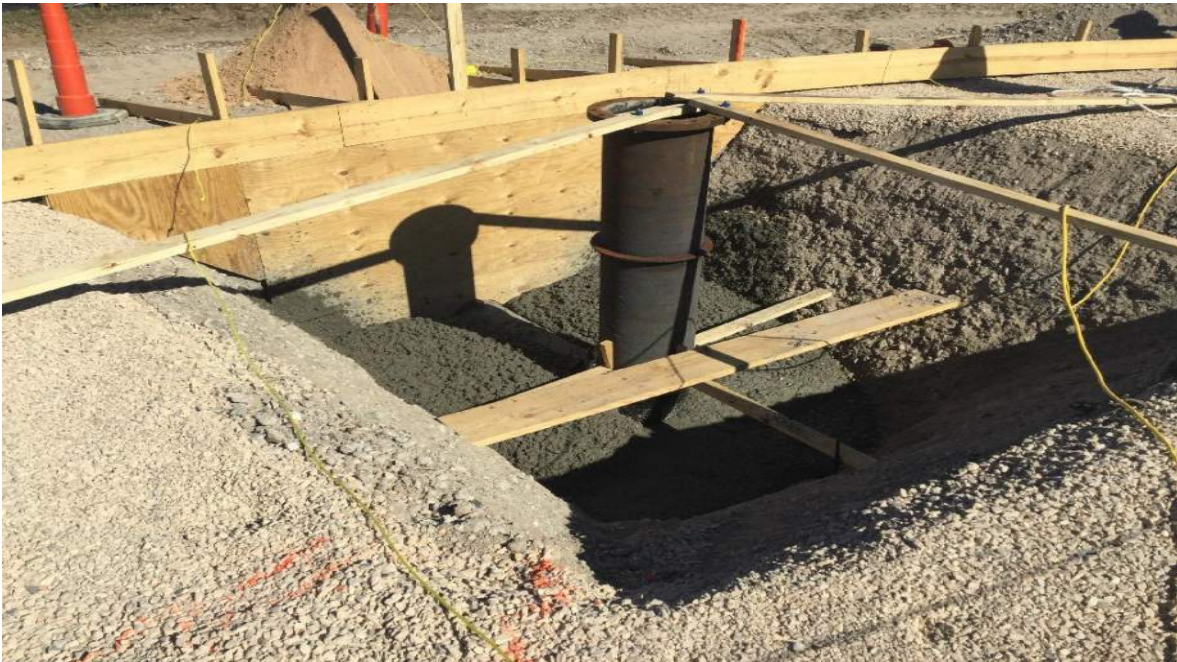
18" ductile iron piping encased in concrete.
