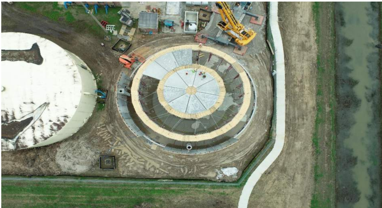
“Bird’s eye view” of the new ground storage tank
