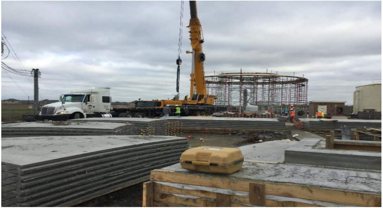
Staging of the 365-ton crane to hang the tank panels
