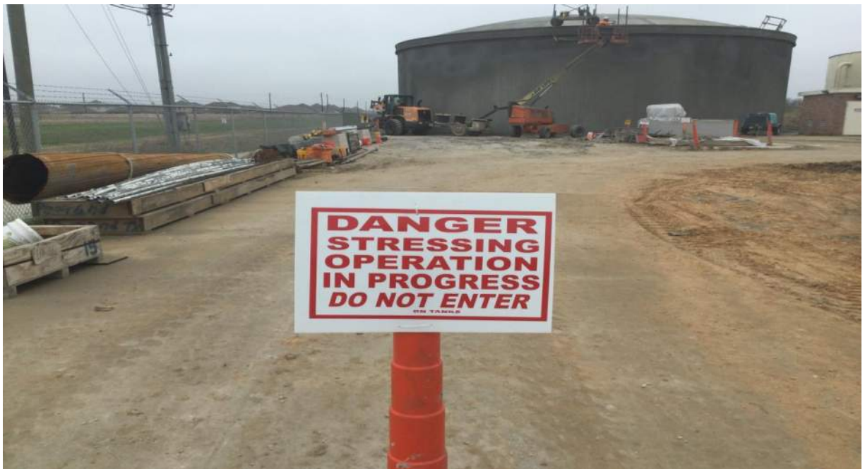
Winding in progress. Site closed during activity.
