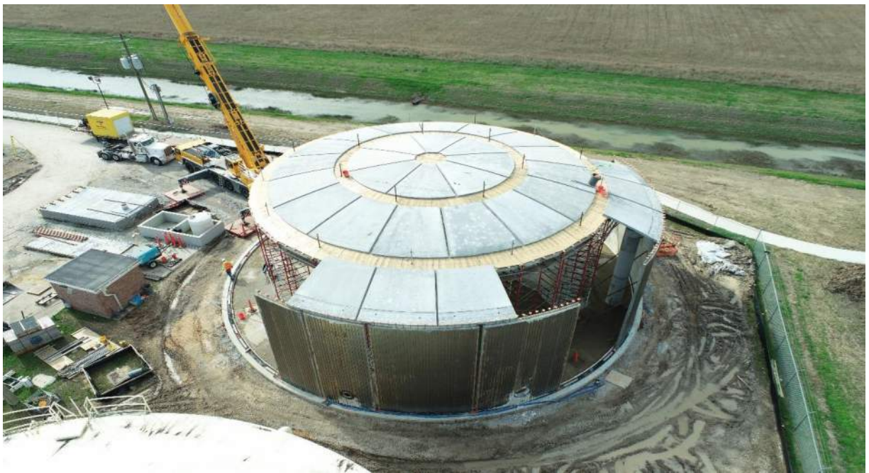
Wall panel erection activity and dome panel placement
