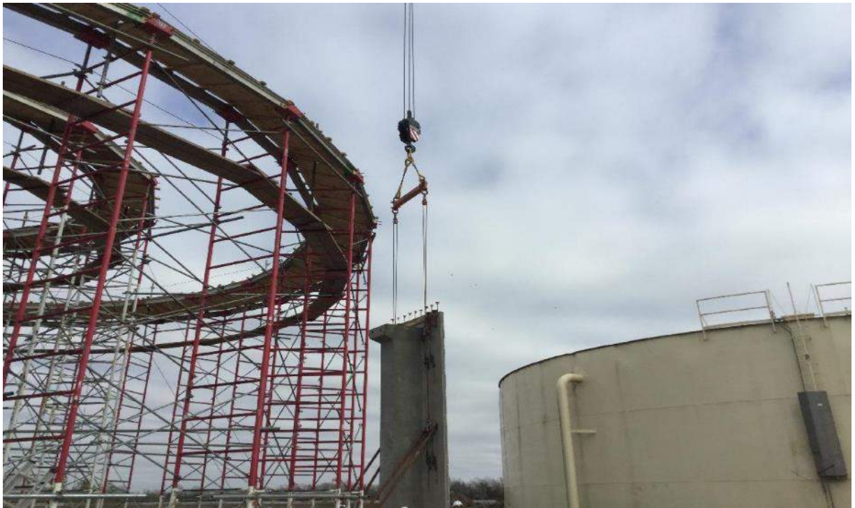
Ground view of the wall panel erection
