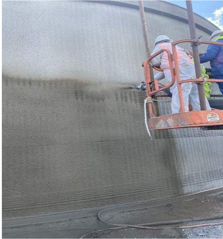
Shotcrete application in progress.
