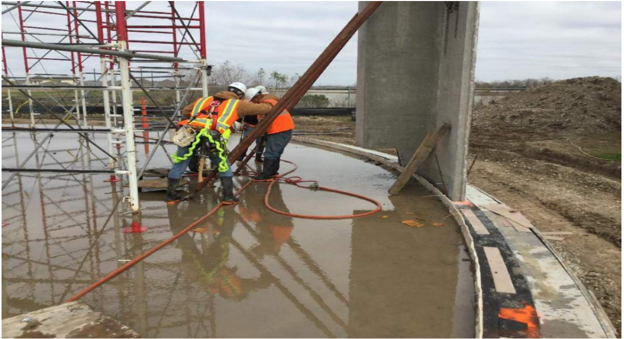
Tank crew bracing wall panel
