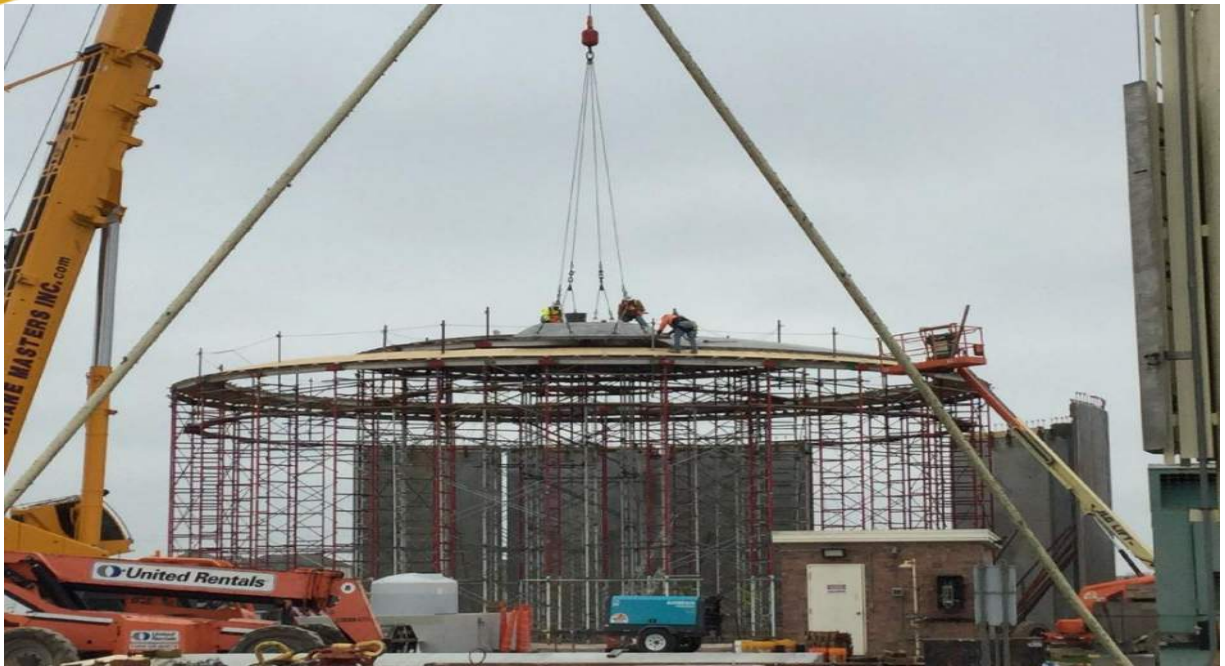
Ongoing progress of the dome-panel installation
