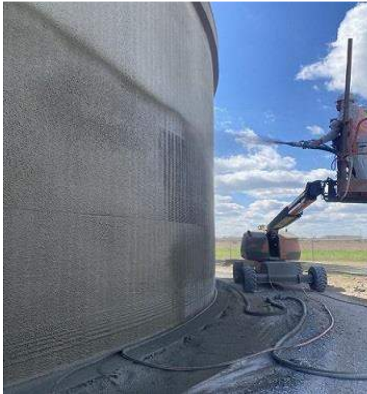
Shotcrete application in progress along the GST.
