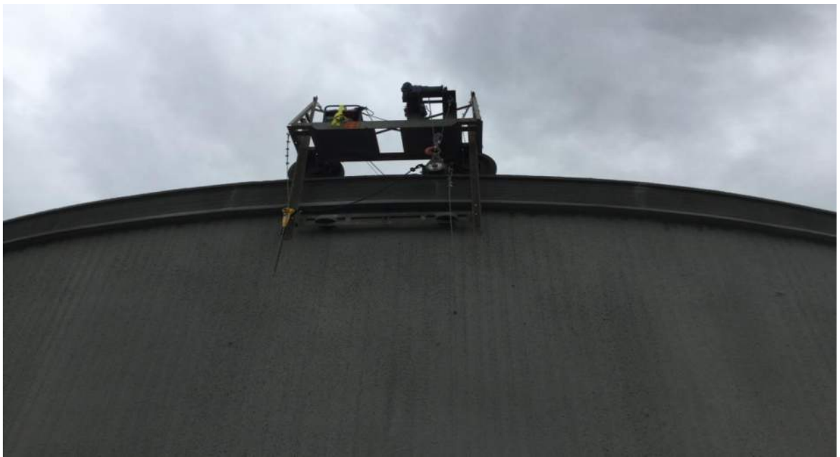
Equipment for pre-stress wire (winding) application around GST.
