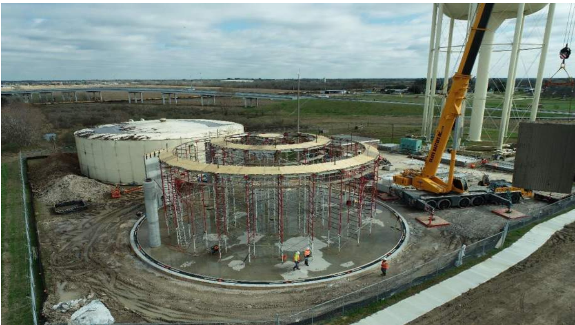
Aerial View of Ground storage tank
