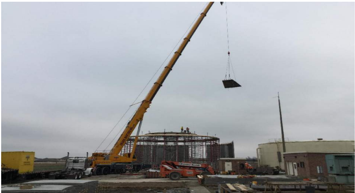
Dome panel being hoisted onto its permanent location
