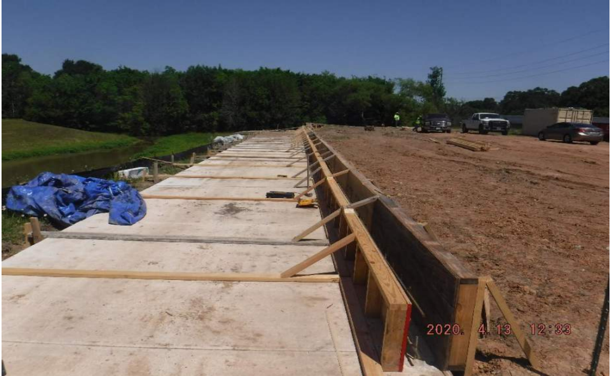
Retaining Wall Formed
