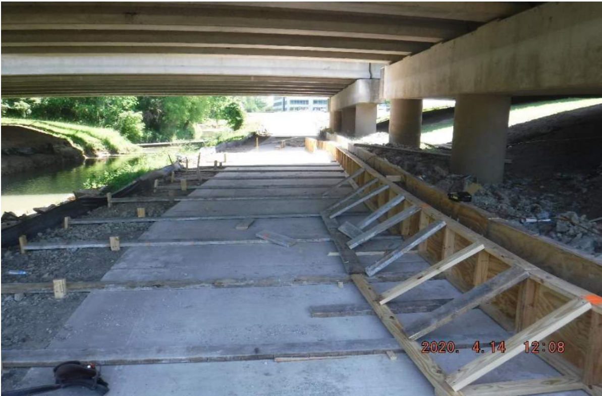
Retaining Wall Formed
