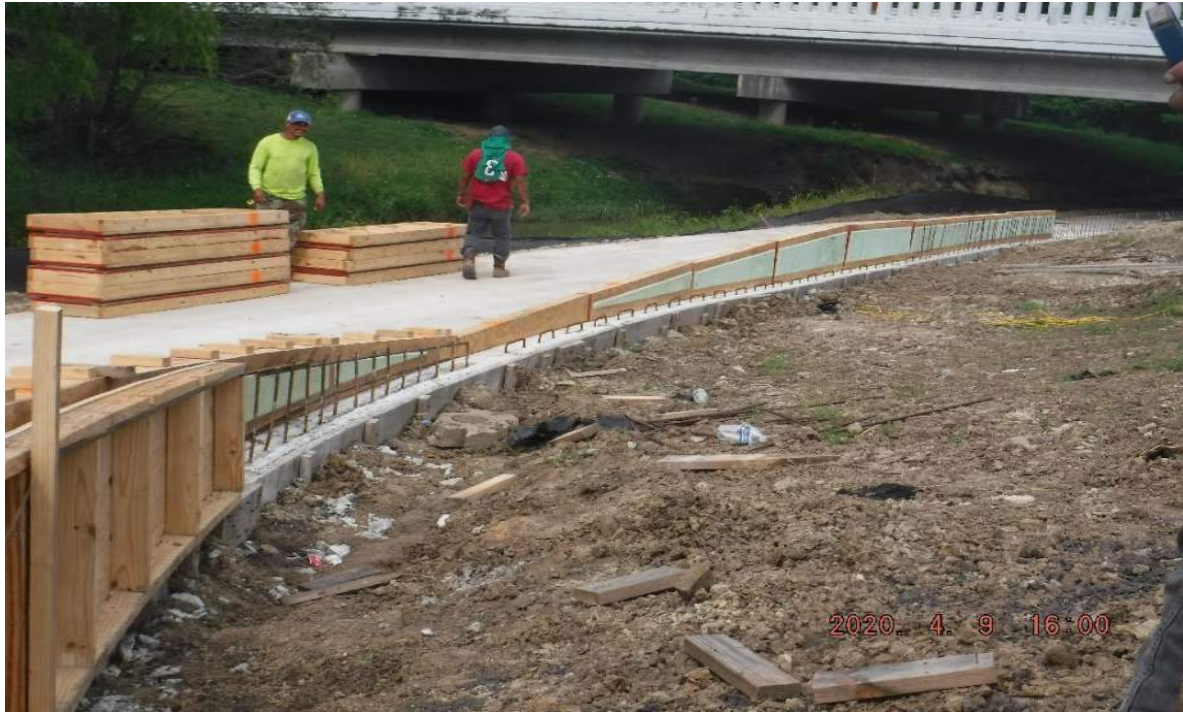
Retaining Wall Installation
