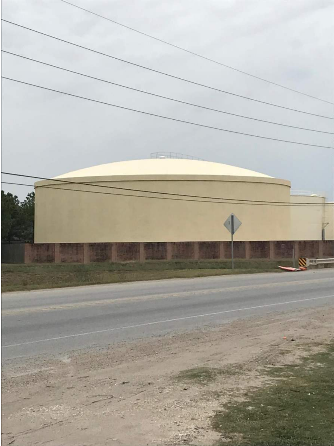
Figure 2: Newly construction 3 MG GST
