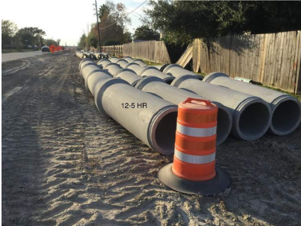
30" RCP staged on the project. 12-05-2019
