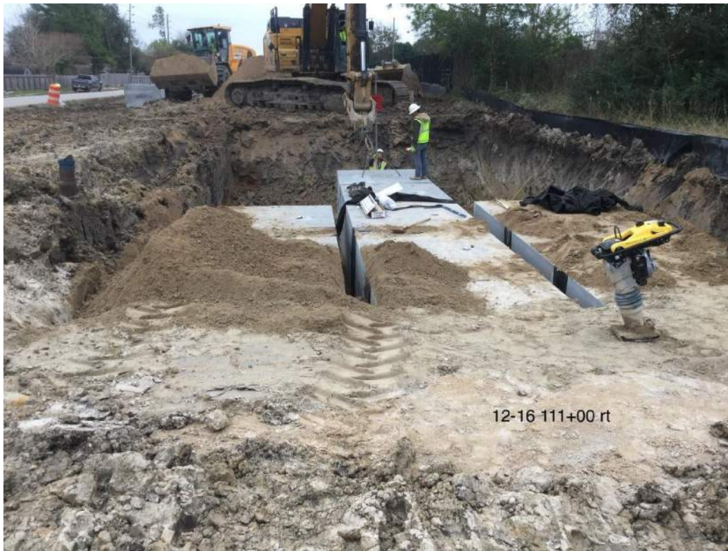
Inline detention installation. 12-16-2019
