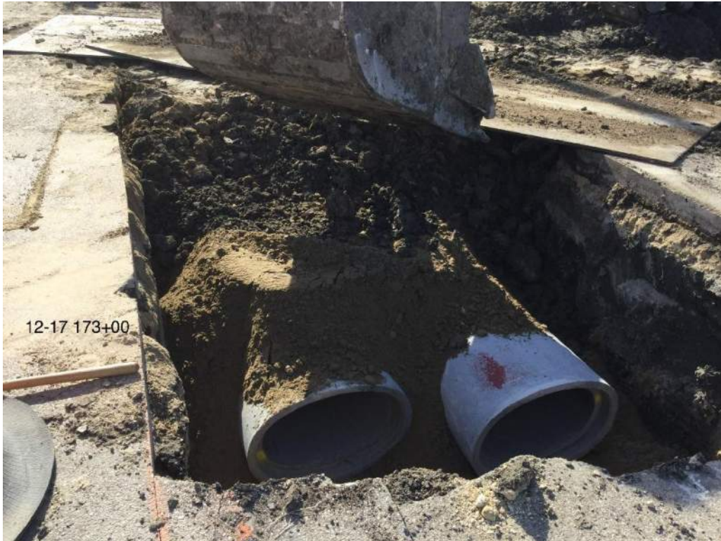
Dual elliptical RCP, storm sewer system B. 12-17-2019
