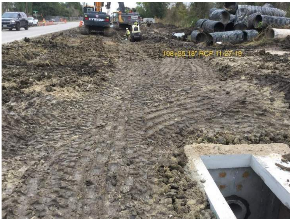
Installation of storm sewer. 11-27-2019
