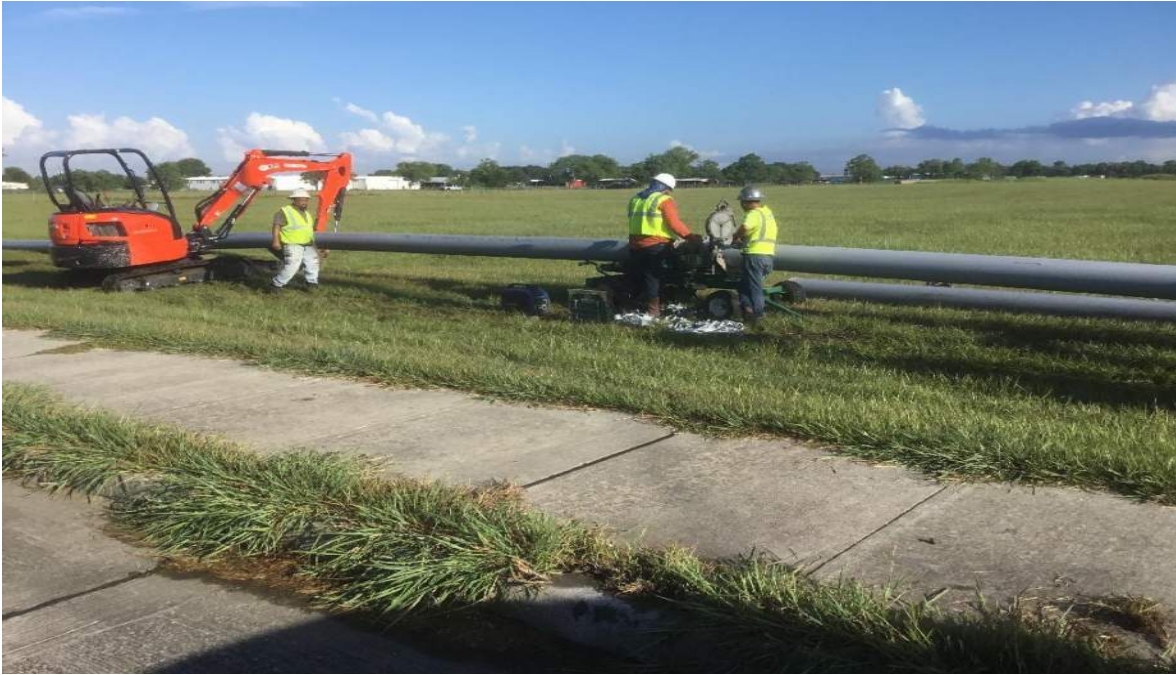
Pipe fusing prior to installation.
