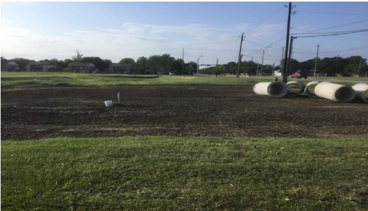
Clearing and grubbing of the proposed Orange-Mykawa LS site.
