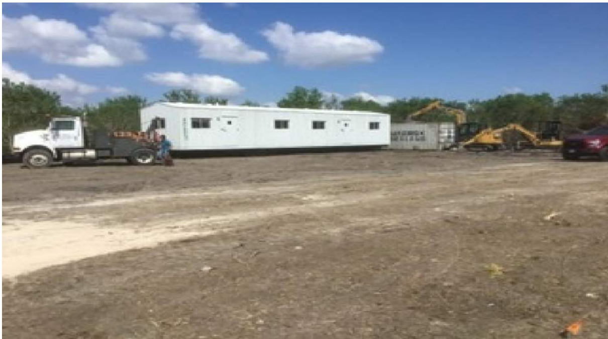
Clearing and grubbing of the proposed Scott-Mykawa LS site and office trailer delivery.
