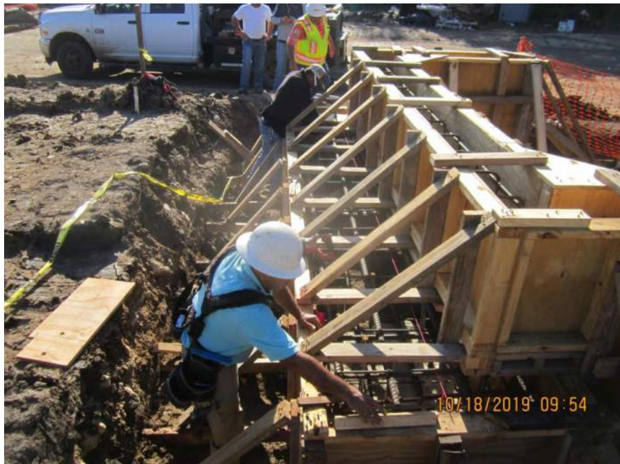
Construction of abutment one.
