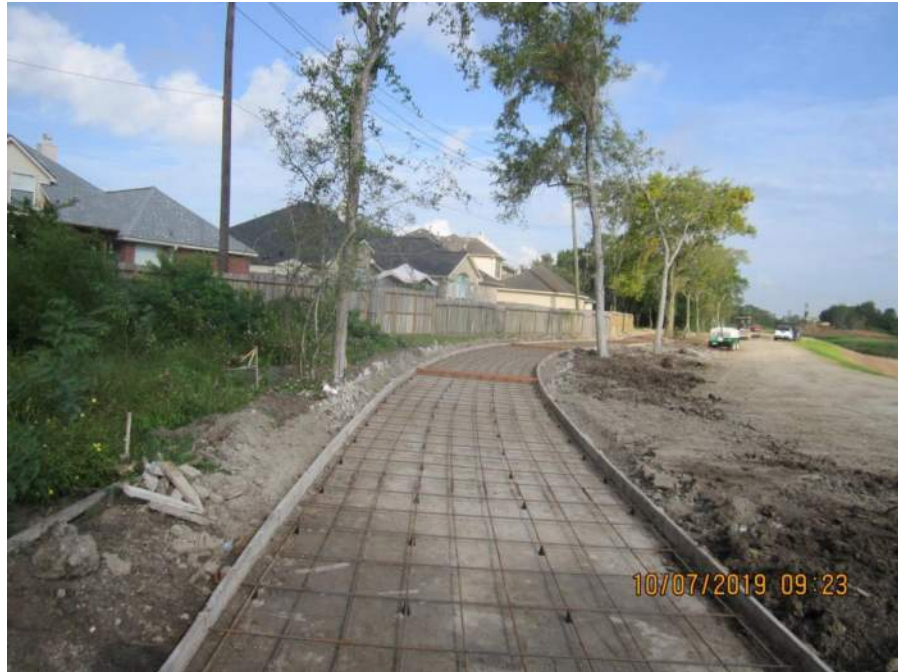
Brazoria County Portion of Trail, formwork behind Clear Creek Park Subdivision.
