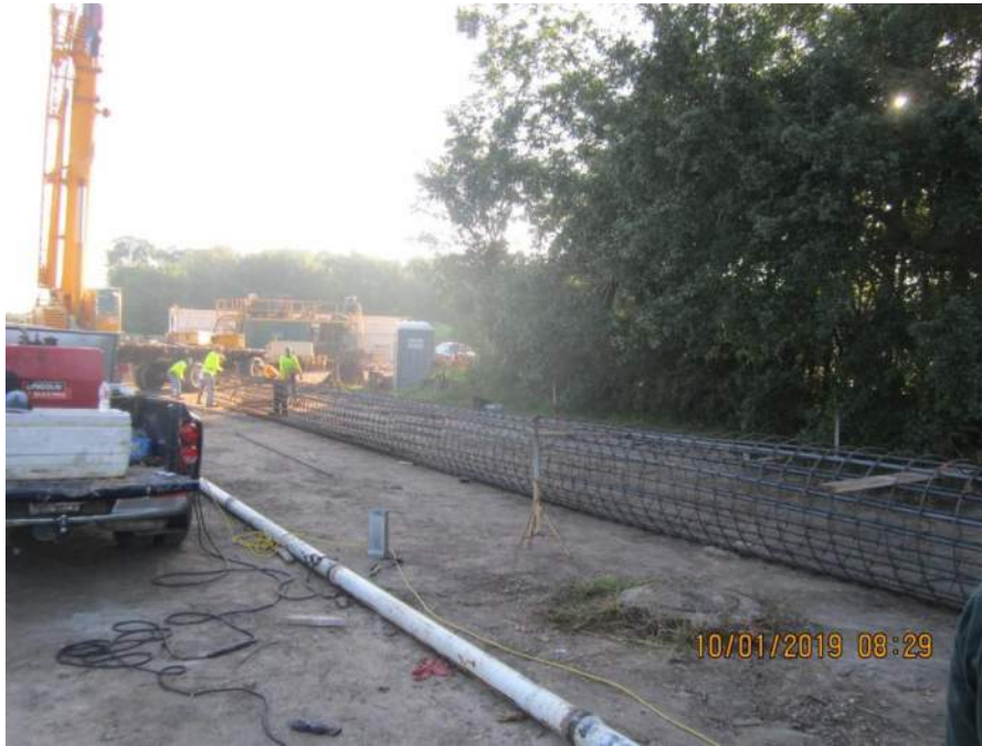
Placing 36-inch drill shaft steel for abutment one.
