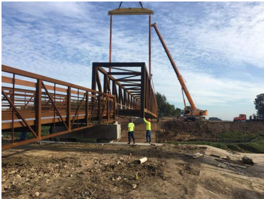
Placing bridge (2 of 2)
