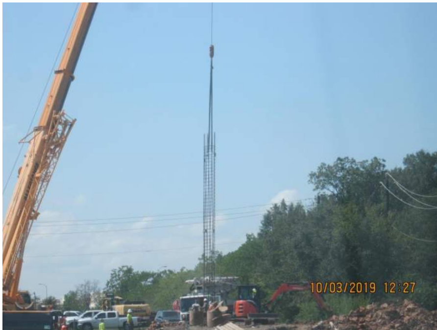
Placing 36-inch drill shaft steel for abutment one.
