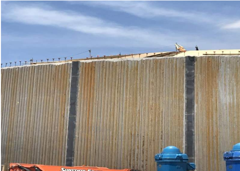
Installing Tank dome forms to pour dome ring.
