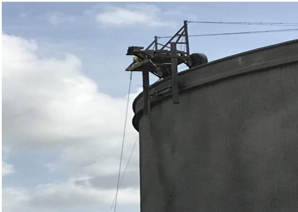
Wire winding of the tank walls for reinforcement.
