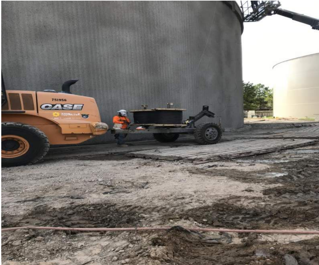
Wire winding of the tank walls for reinforcement.
