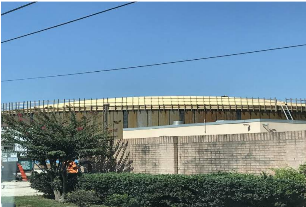
Installing Tank dome forms to pour dome ring.
