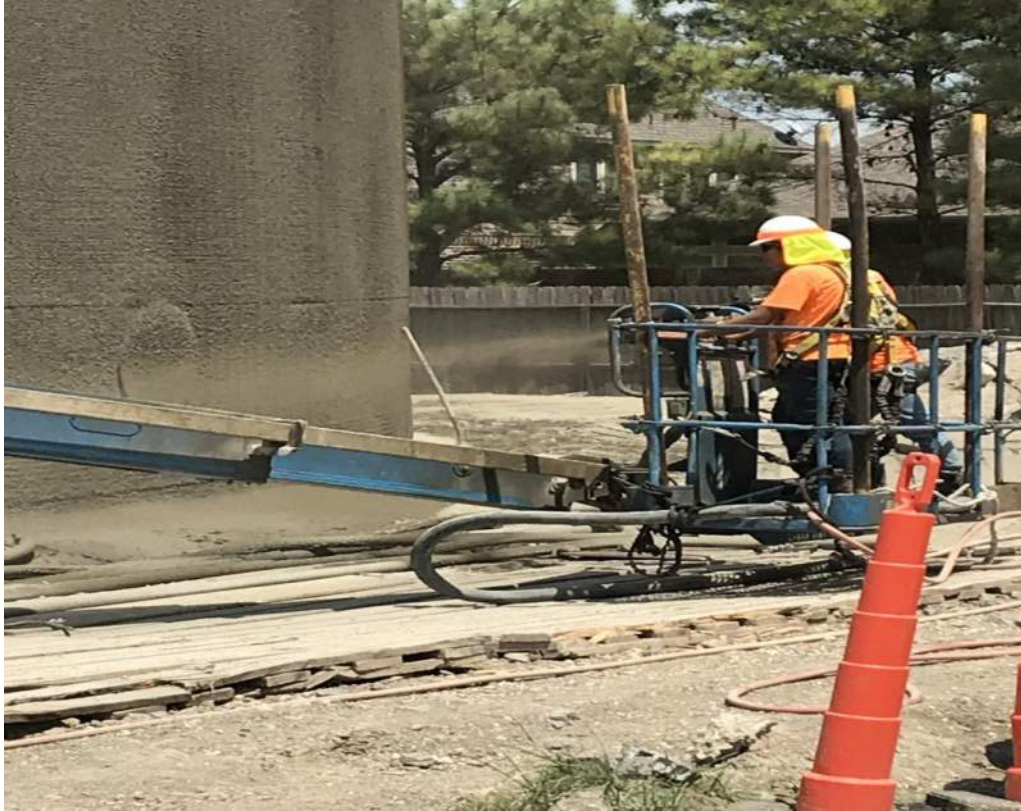
Shotcrete walls of the tank
