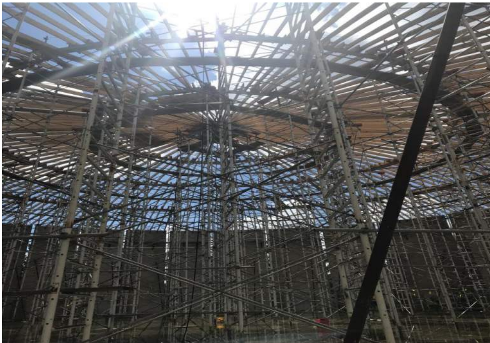
Building forms for the dome ring to be poured
