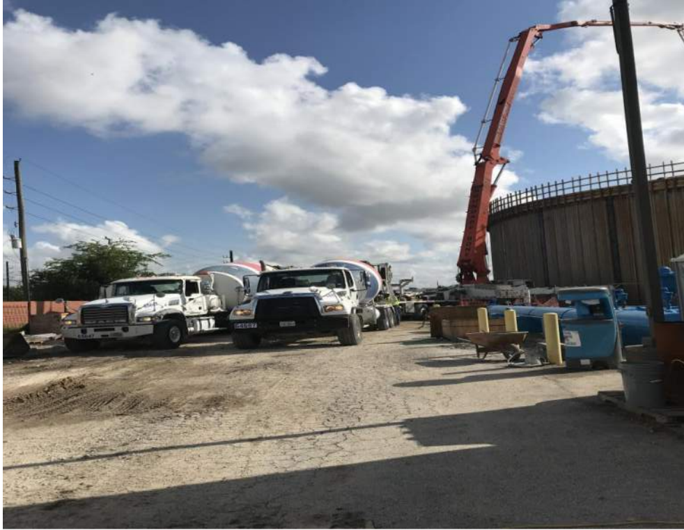
Shotcrete walls of the tank
