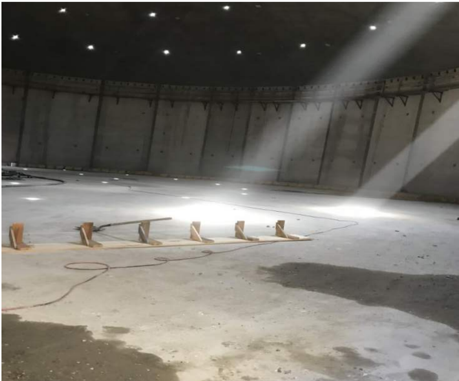
Removal of dome forms and scaffolding.
