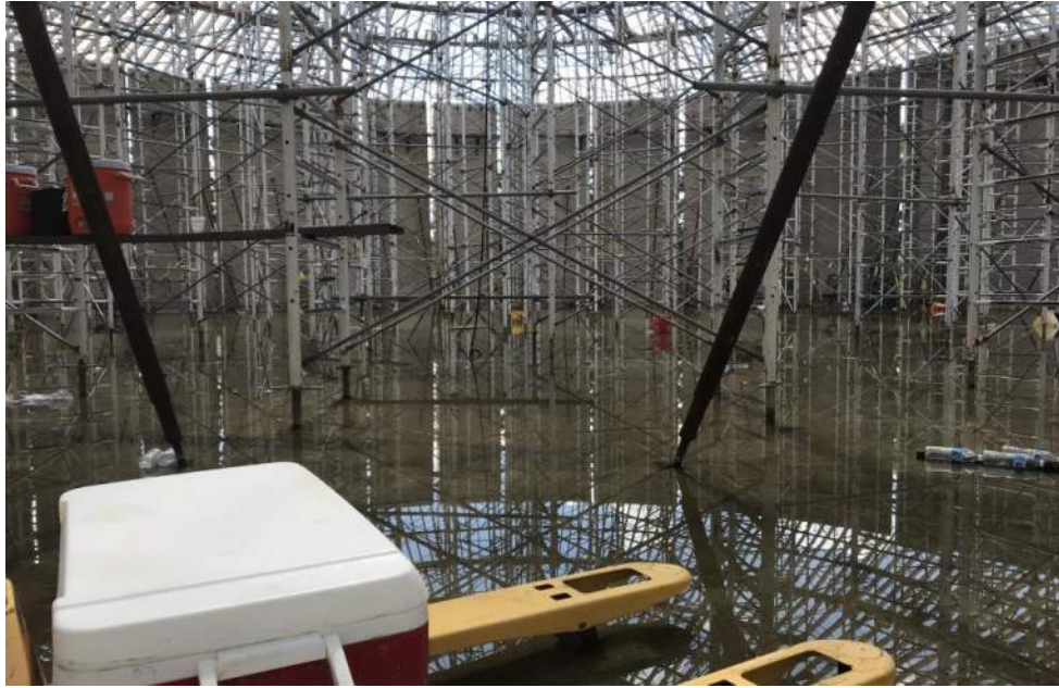
Tank walls set into place and braced
