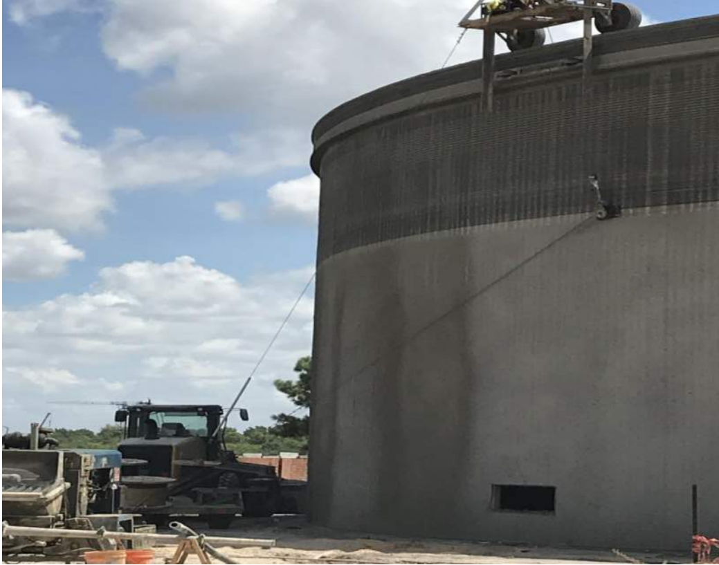
Wire winding of the tank walls for reinforcement.
