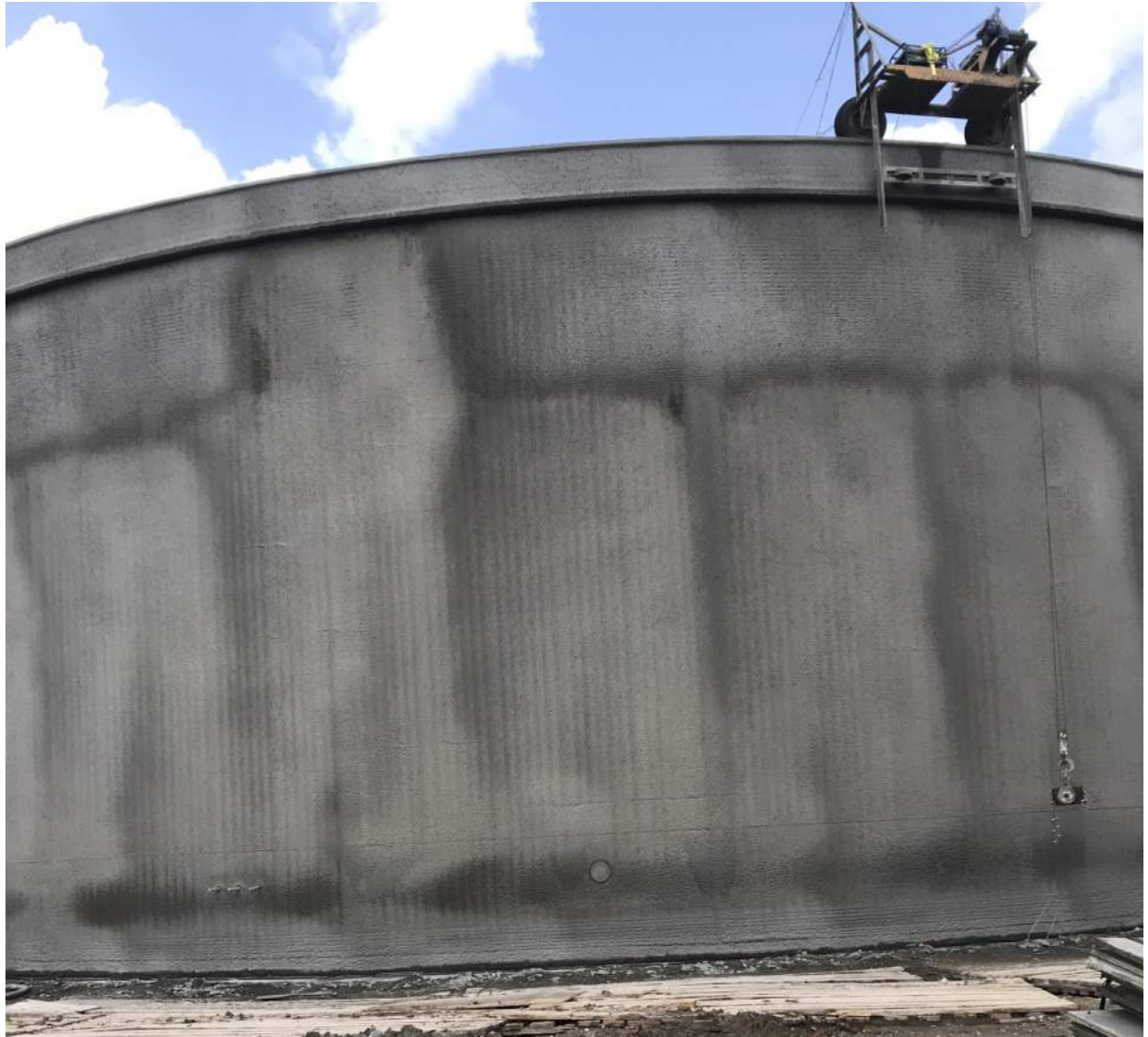
Final Wire winding and Shotcrete of the tank walls for reinforcement.
