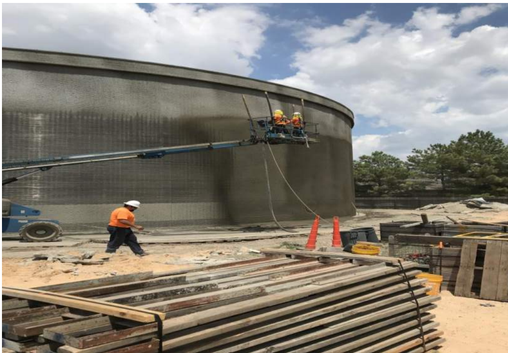
Shotcrete walls of the tank
