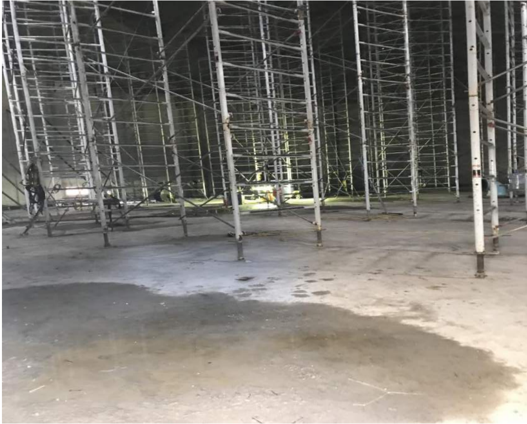
Removal of dome forms and scaffolding.
