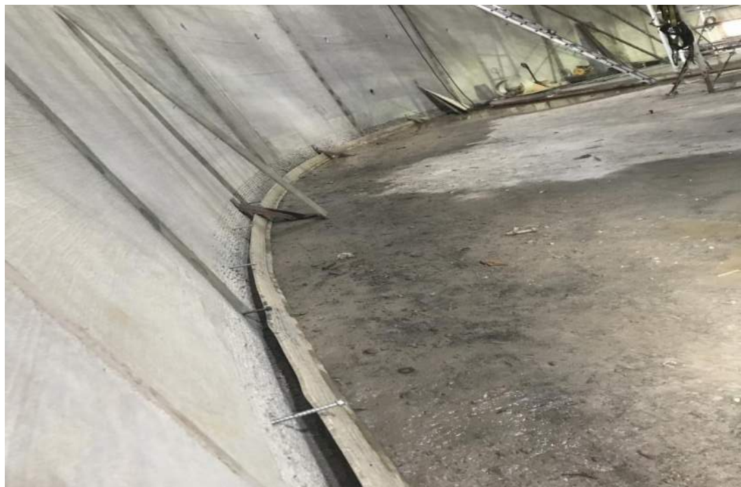
Removal of dome forms and scaffolding.
