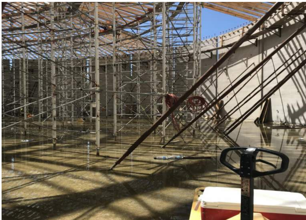
Tank walls set into place and braced
