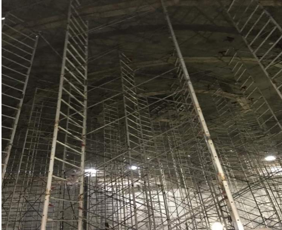
Removal of dome forms and scaffolding.
