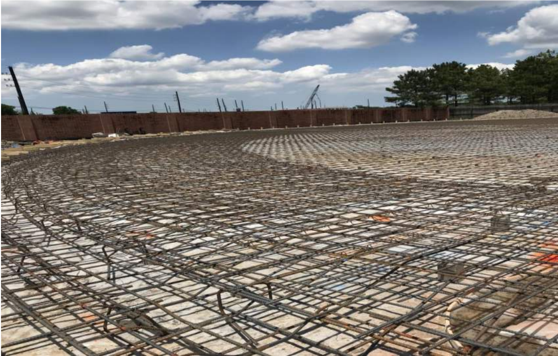
Steel for the tank pad
