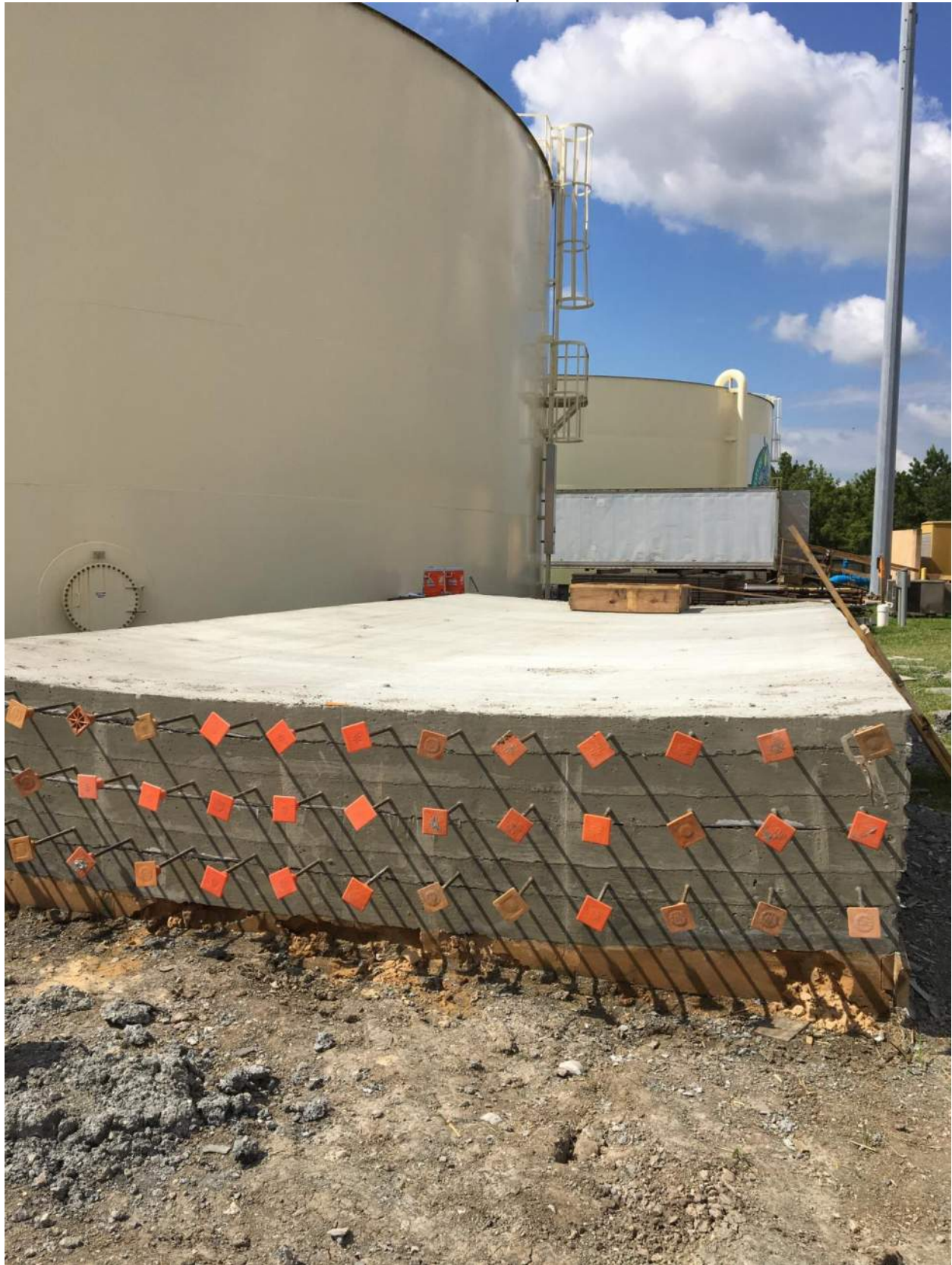
Pre-cast wall panels
