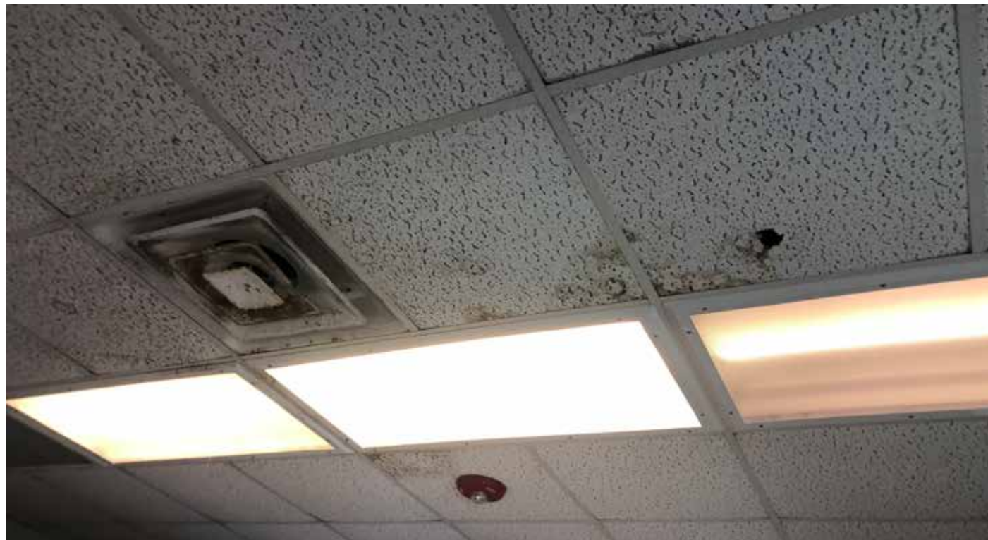
Kennel Room- Ceiling
