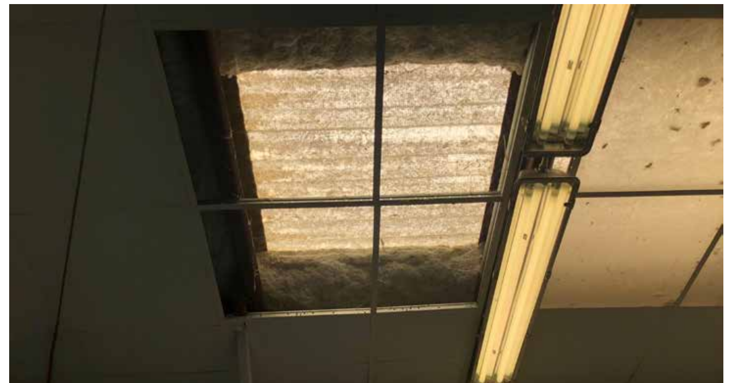
Dogs - Stray Hold Kennels - Ceiling Condition / Natural Daylighting
