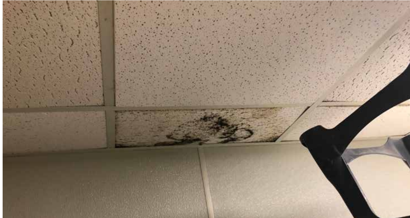
Existing Ceiling Tile
