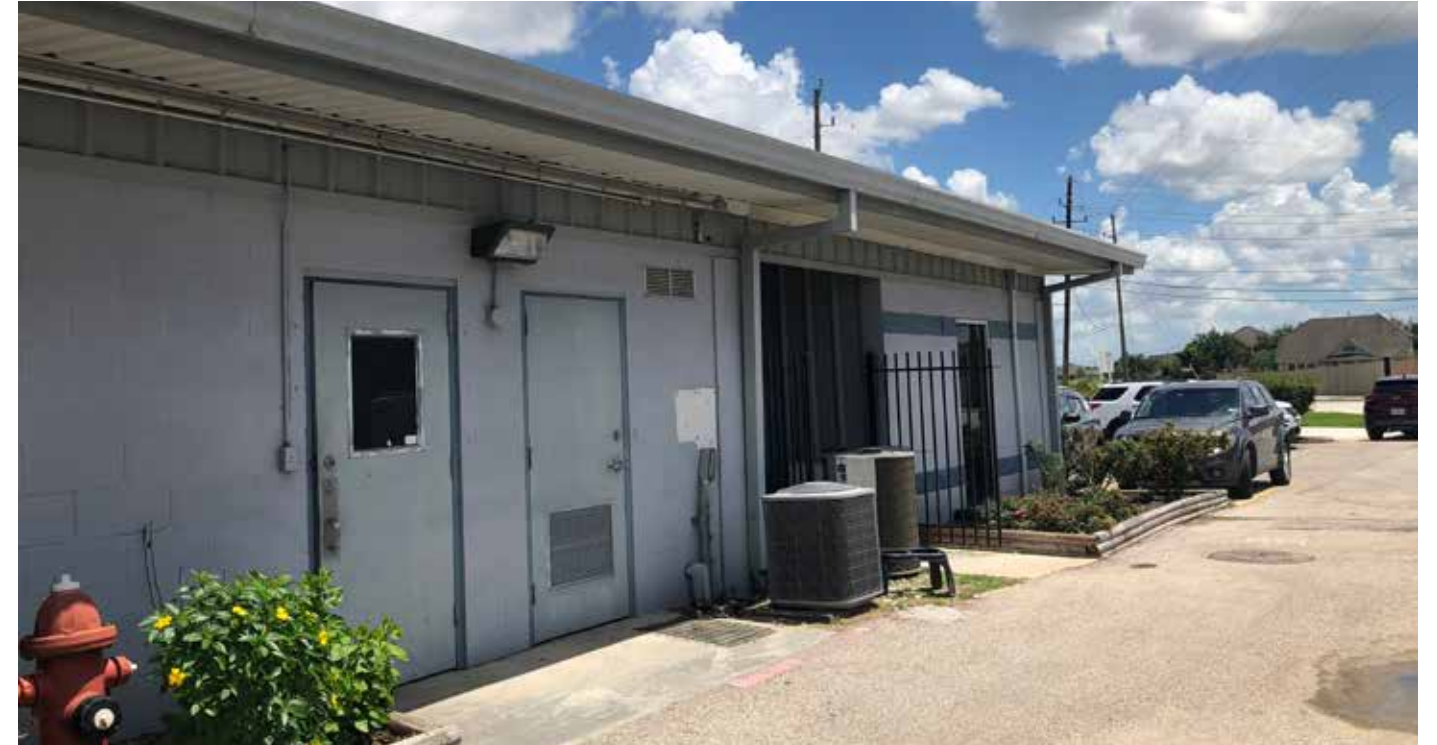
Exterior at Medical/Vet Clinic
