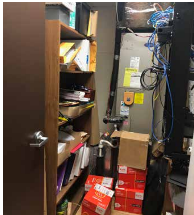
Mechanical Room - with Storage
