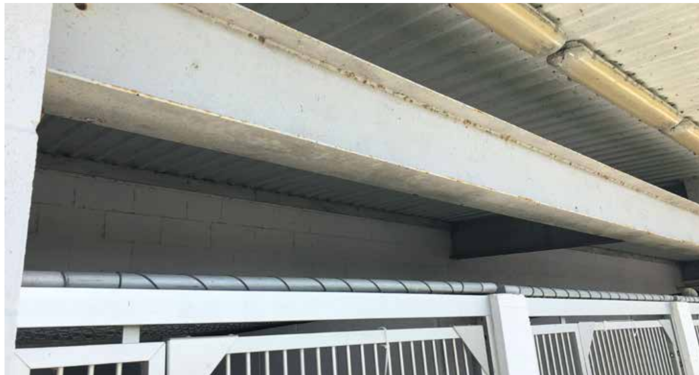
Outdoor Run - Structure
