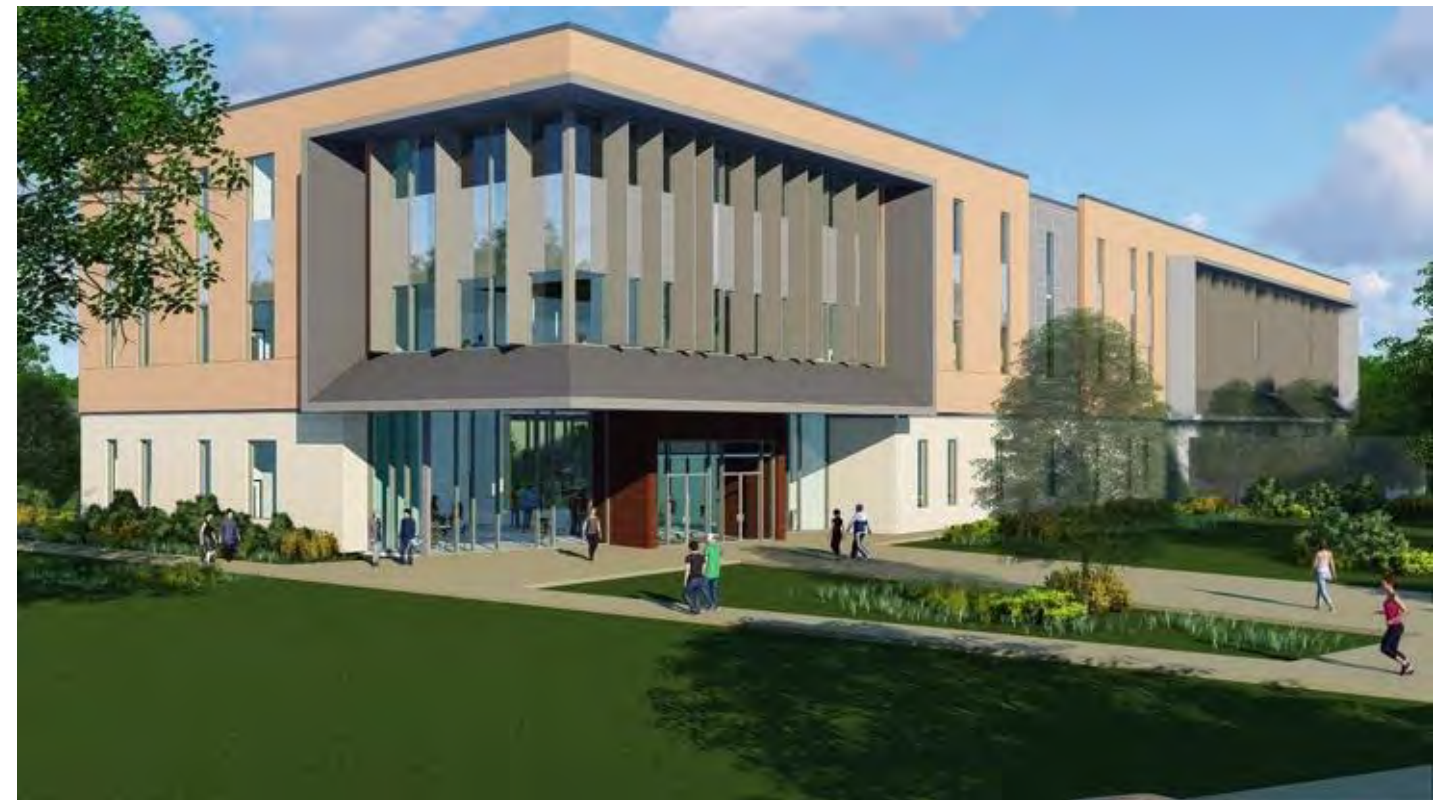
The Health Sciences building will provide laboratories, graduate nursing programs and classrooms
