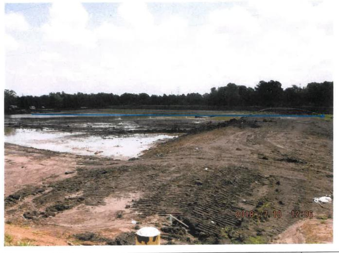
**Description:** View of the sedimentation basin, showing stormwater flow from the north ditch, through a cut in a berm (looking northeast). 42 (DSCF0857)
