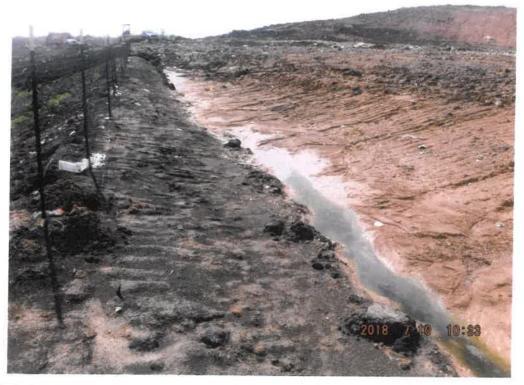
**Description:** View of the truck clean-out area, noting trash accumulation in the background and the stormwater flow-path.
