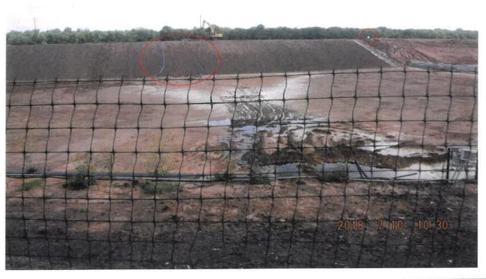
**Description:** View of temporary stormwater pump (not running) and two hoses in new cell being constructed, noting a groundwater seepage pump on the right.
