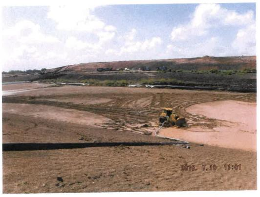
**Description:** View of temporary stormwater pump in new cell being constructed, discharging to the north ditch.
