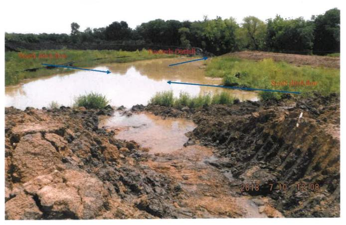
**Description:** View of the mixing area in the sedimentation basin, prior to discharge through the outfall, noting the silt fencing and water color/clarity (looking east).
