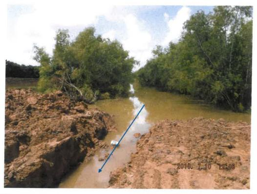
**Description:** View of the south ditch, showing stormwater flow through a cut in a berm, into a mixing area for the north and south ditch, and towards the outfall. (looking east).
