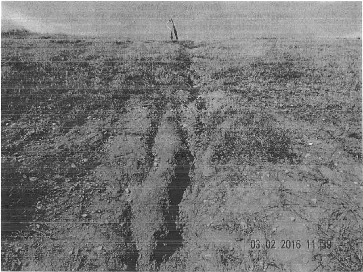
Photograph 2 of 2: Another area of erosion of cover was observed.
