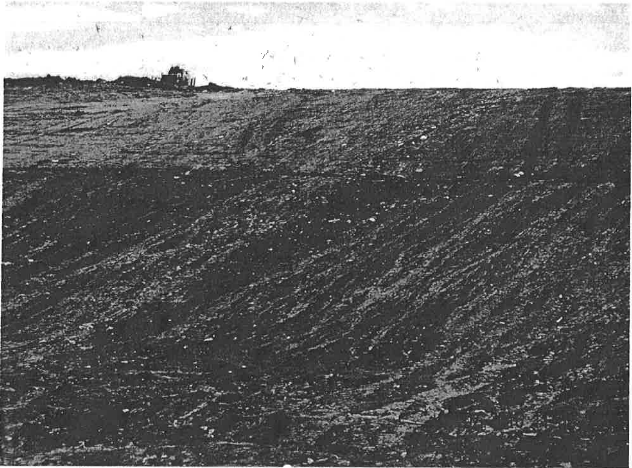
Photograph 1 of 2: The erosion of cover previously observed on December 18, 2015 appeared to have been repaired.
