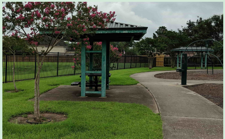
Current condition of Buildings | Shelters | Pavilions at Pine Hollow Park.
