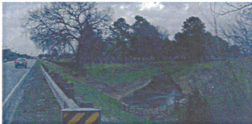
CURRENT DRAINAGE AT MARY'S CREEK IN PEARLAND
